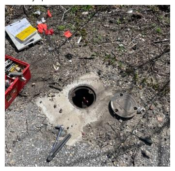
**Below: Well MW-05**. This well was found to be undamaged, although the lid of the steel casing could no longer be secured and appeared to have been broken off forcibly to obtain access to the well. The well cap was also missing. The well was sounded and found to be fully open.
