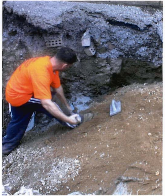
Plugging former effluent pipe with concrete.
