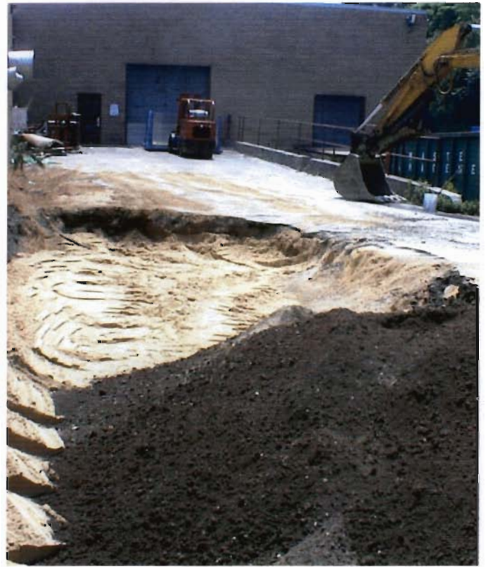
Backfilled excavation with clean fill and RCA.
