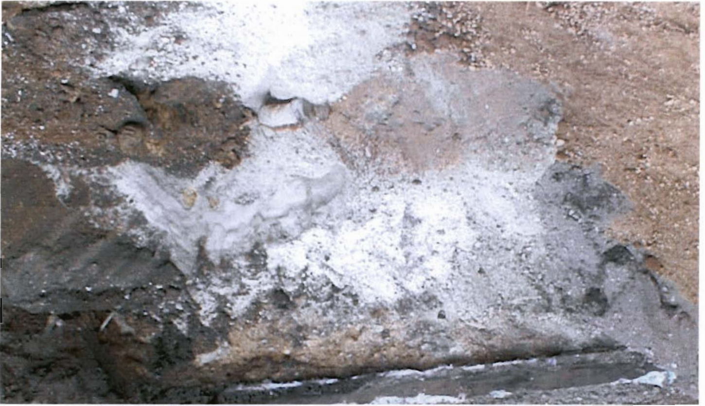
View of south bottom of excavation and exposed building footing.
