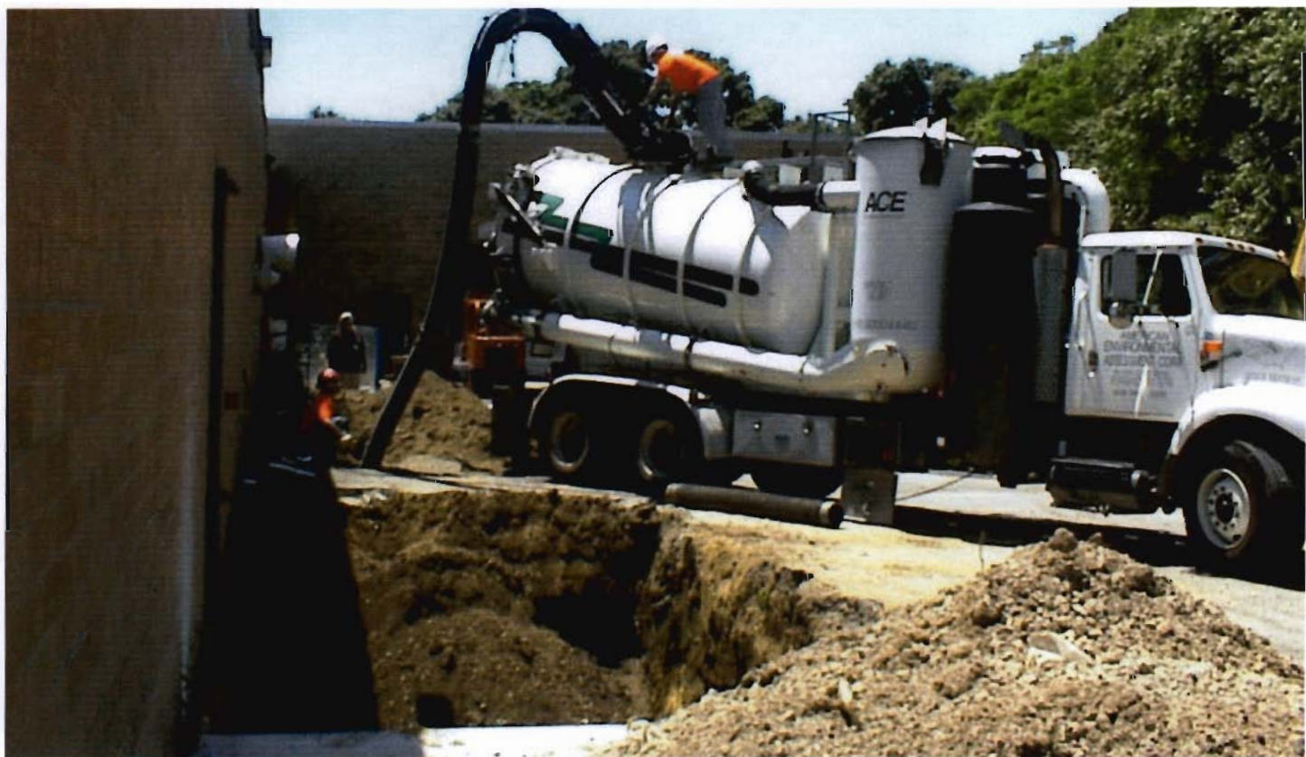
High vacuum excavator removing bottom sediments from the "distribution box" .
