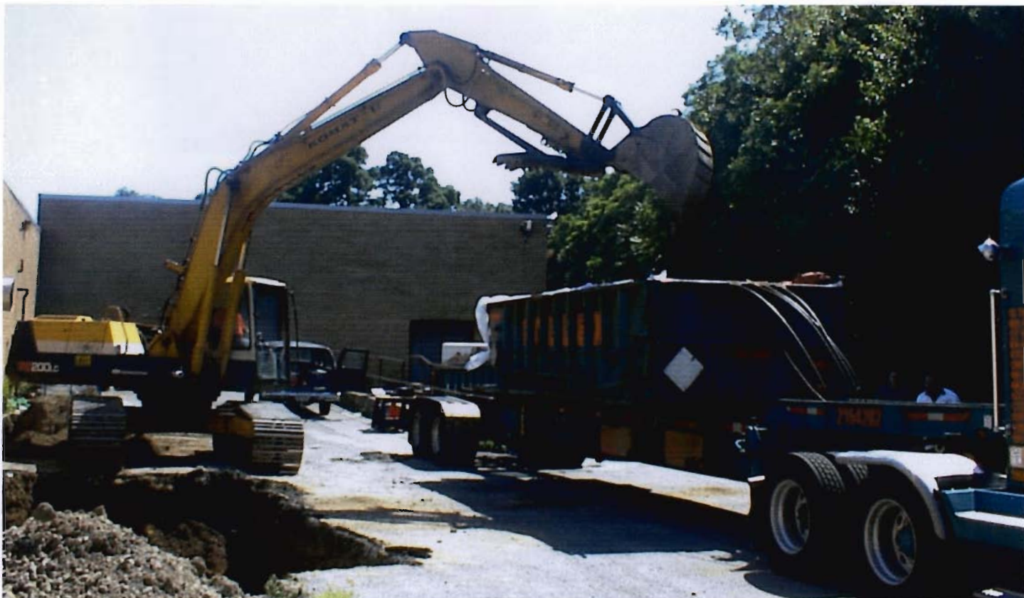
Loading of contaminated soil for immediate shipment to the Stablex Facility.
