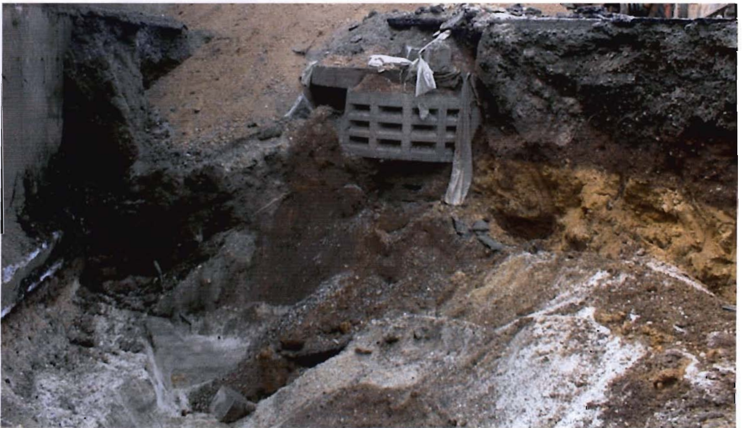
Southern view of excavation showing exposed side of "OF-1" and building footing.
