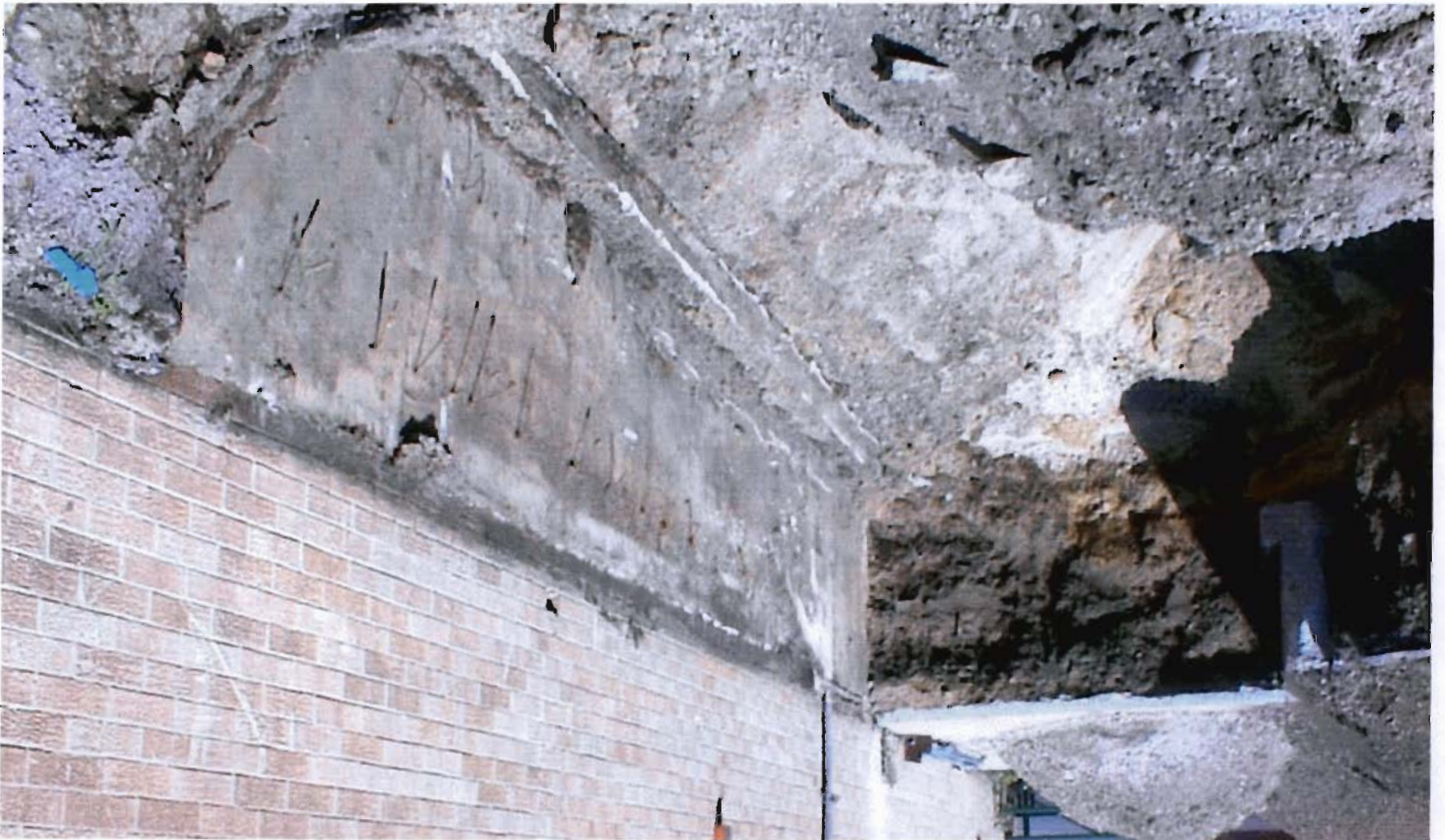
Northern view of excavation and exposed building footing.
