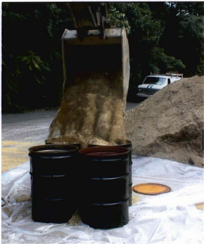
Loading of soil from the south bottom into drums.
