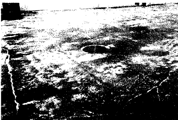
SD-3 Prior to cleanup
