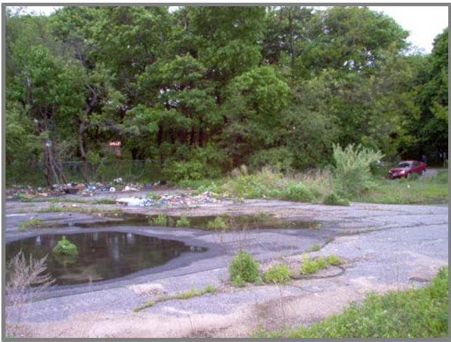
Photo left. Looking accross the pad towards the entrance way.
