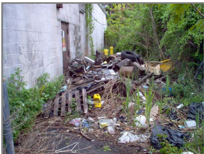
Photo left. ServAll's locked side doorway.
