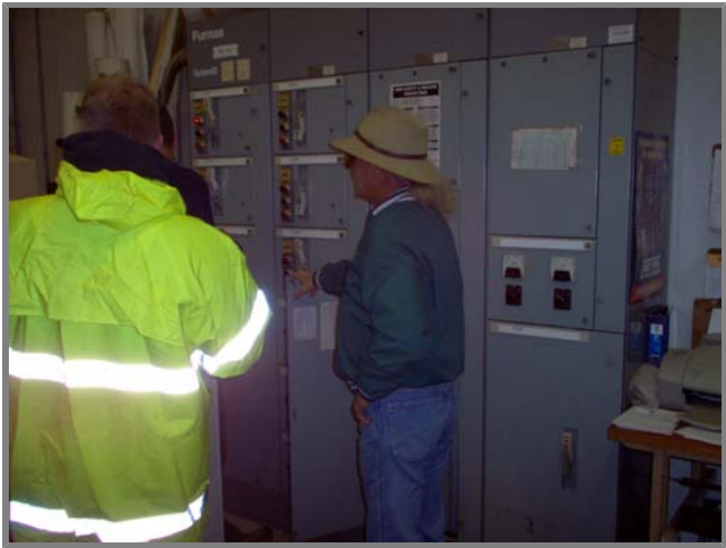
Photo left. Inside the treatment plant.
