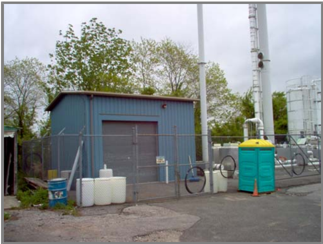
Photo left. Treatment building
