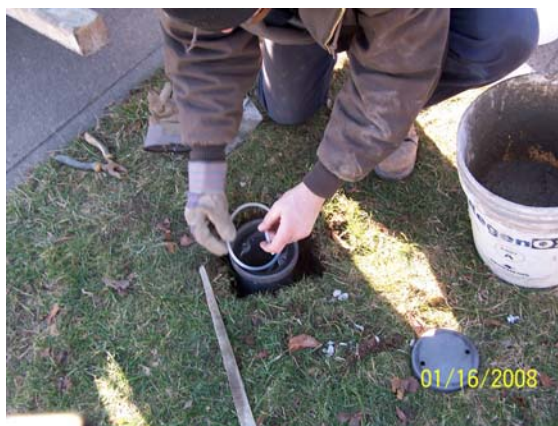
AI DP08 Installing Flushmount
