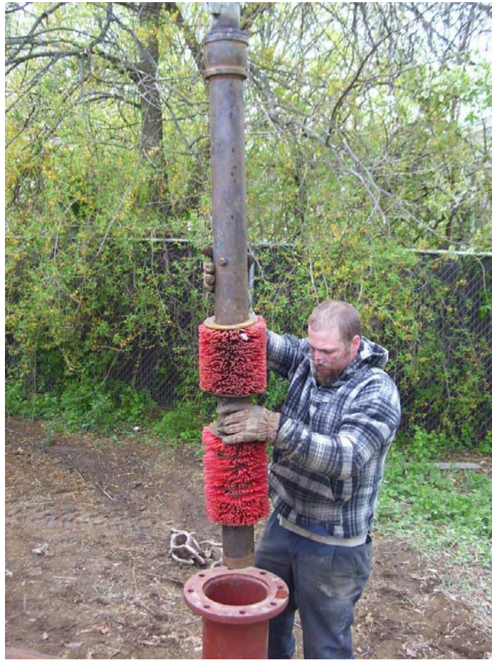
Brush used to clean well casing and screen.
