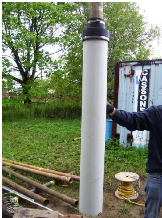
Casing installed around pump/motor before installation.
