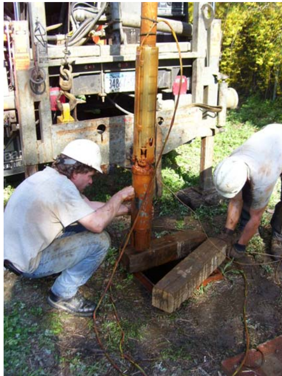
Condition of RW-1 pump/motor prior to well rehabilitation.
