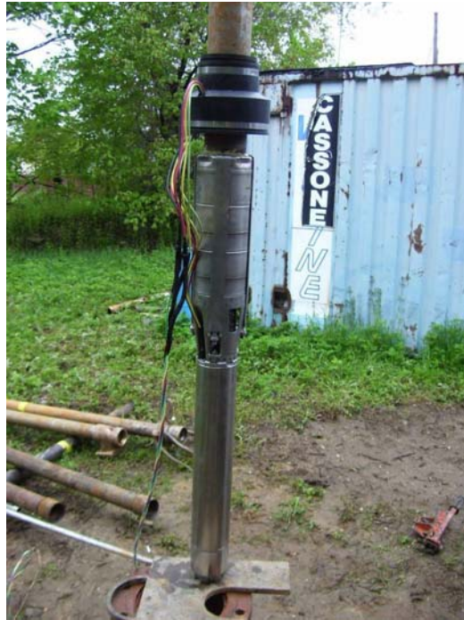
Grunfos pump/motor installed post well rehabilitation.
