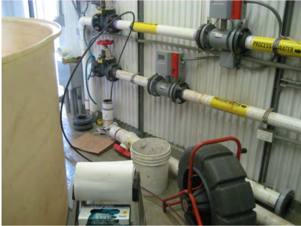
Photograph 1 – Borescoping of effluent piping.
