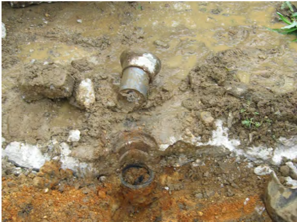
Photograph 10 – Below grade floor drain.
