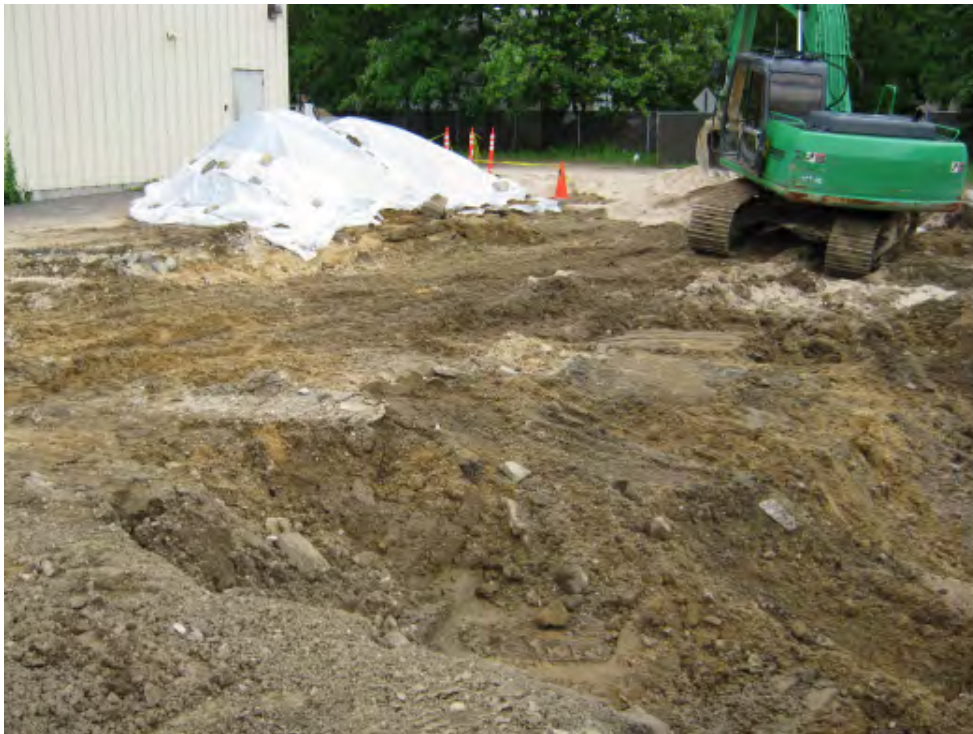
Photograph 14 – Excavation of soil utilizing an excavator.
