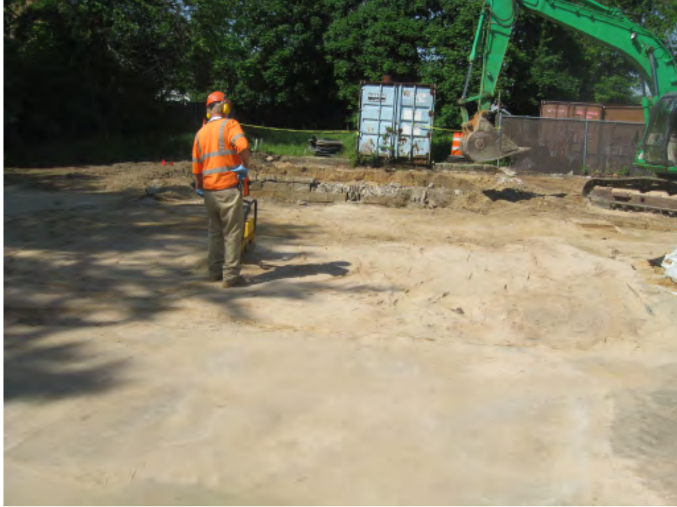
Photograph 25 – Spreading and compaction of clean fill.
