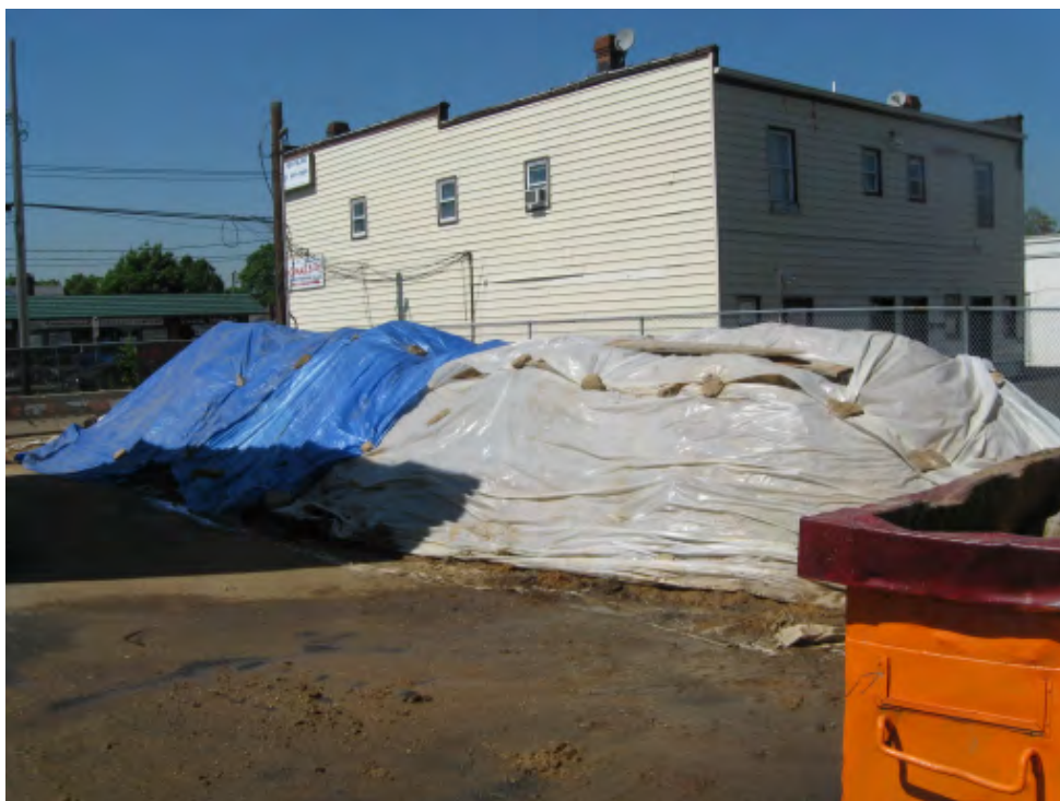
Photograph 22 – Soil pile staged on eastern portion of the site.
