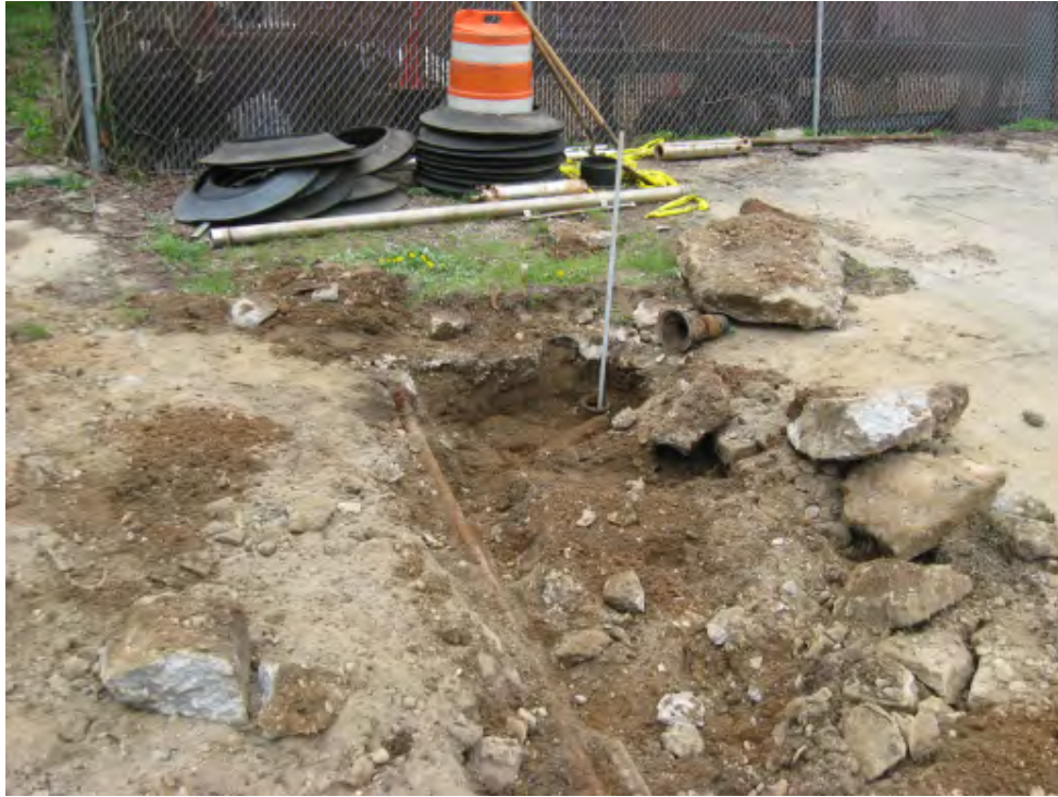
Photograph 13 – Below grade piping network, showing a below grade floor drain.
