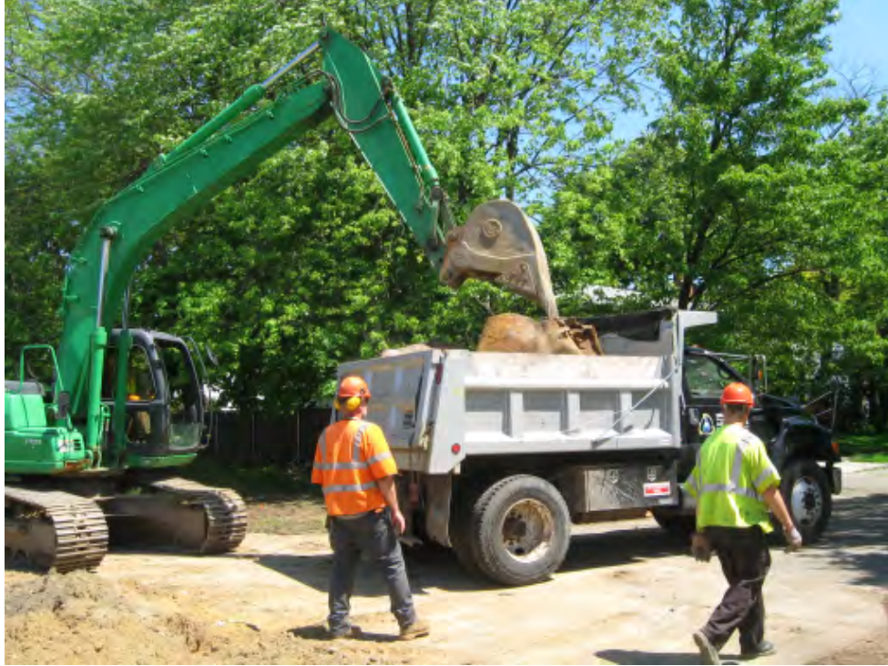
Photograph 23 – Loading of metal debris for later recycling.
