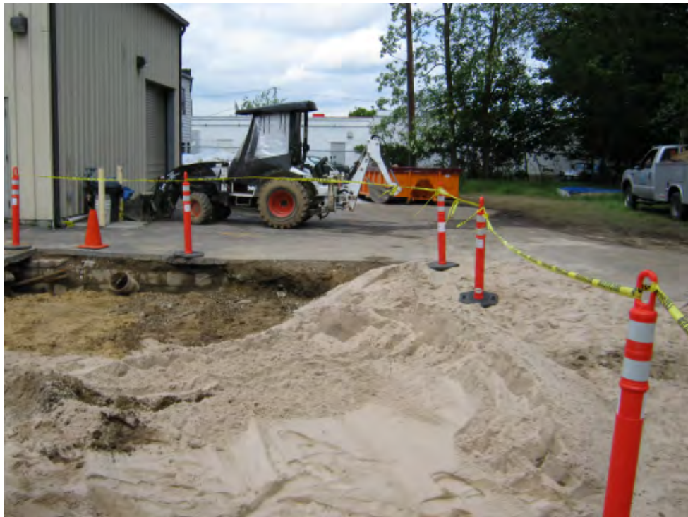
Photograph 24 – Clean fill installation in the southern portion of the overall excavation.
