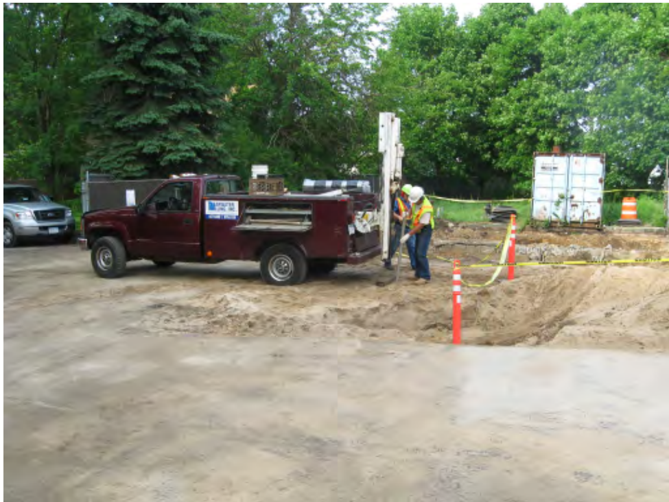
Photograph 26 – Geoprobe investigation at Dry Well 2.
