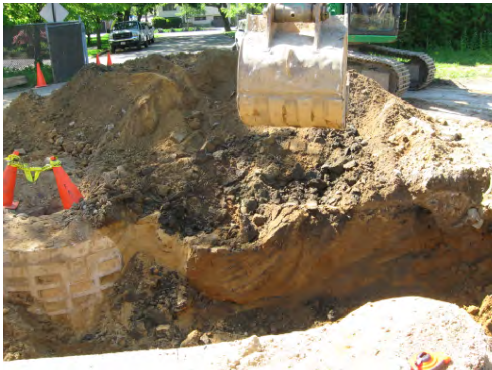
Photograph 20 – Southernmost identified dry well and stained soil.
