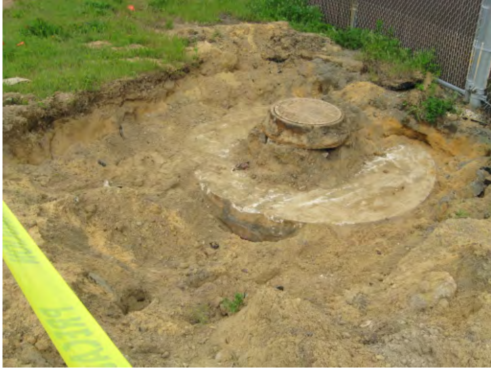
Photograph 17 – Northernmost identified dry well.
