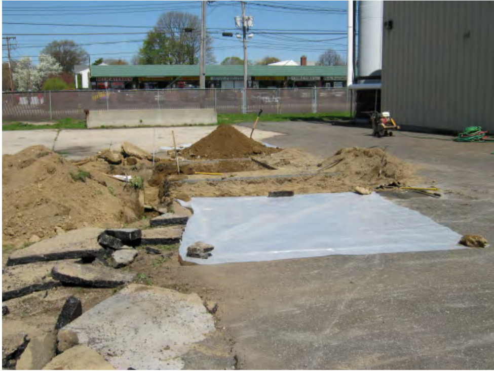
Photograph 7 – Excavation of UST area and staging of soil on poly-sheeting.
