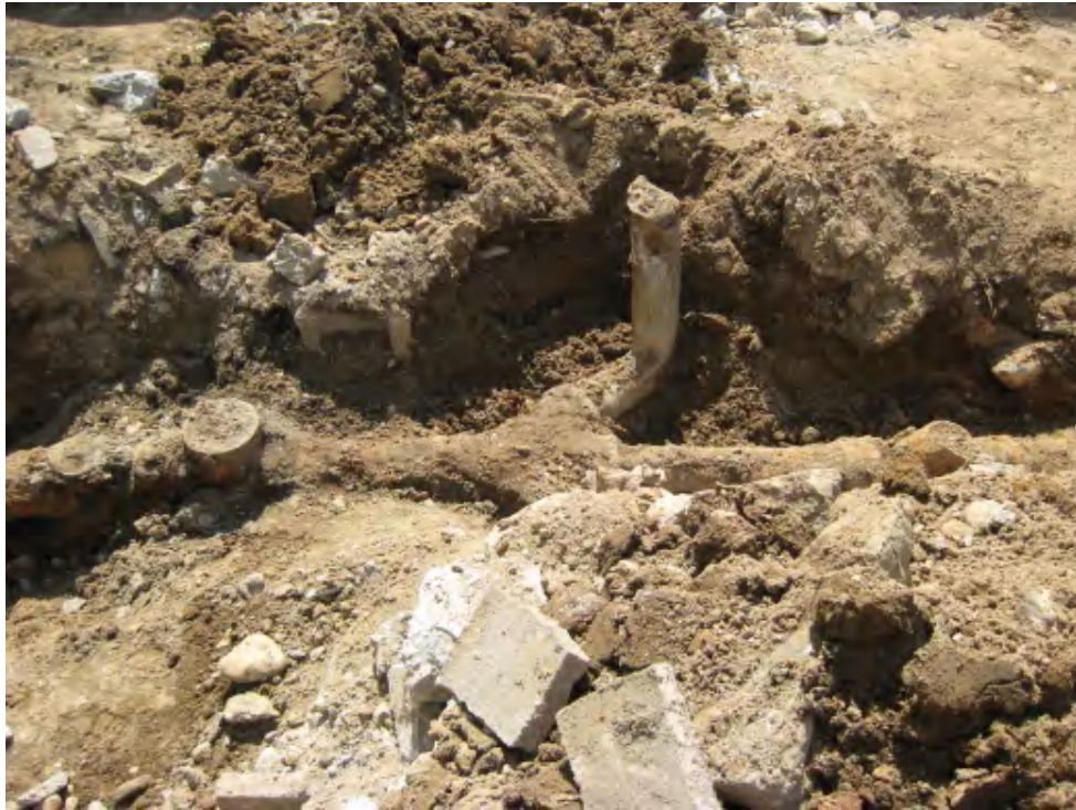
Photograph 9 – Portion of below grade piping and below grade drainage structure network.
