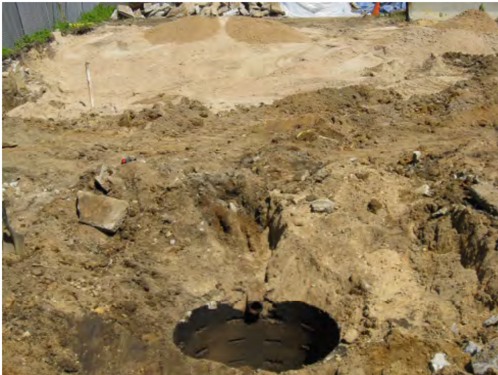
Photograph 18 – Westernmost identified dry well, showing discharge piping.
