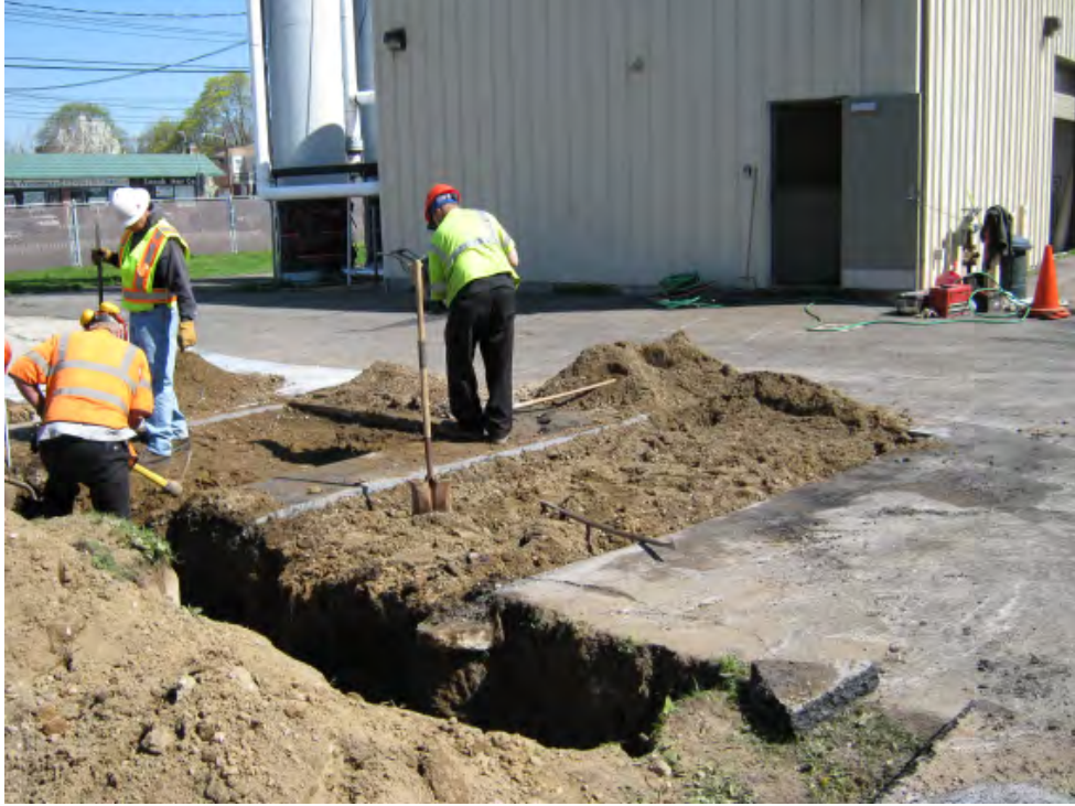
Photograph 3 – Hand-clearing at Wash Water UST excavation area.
