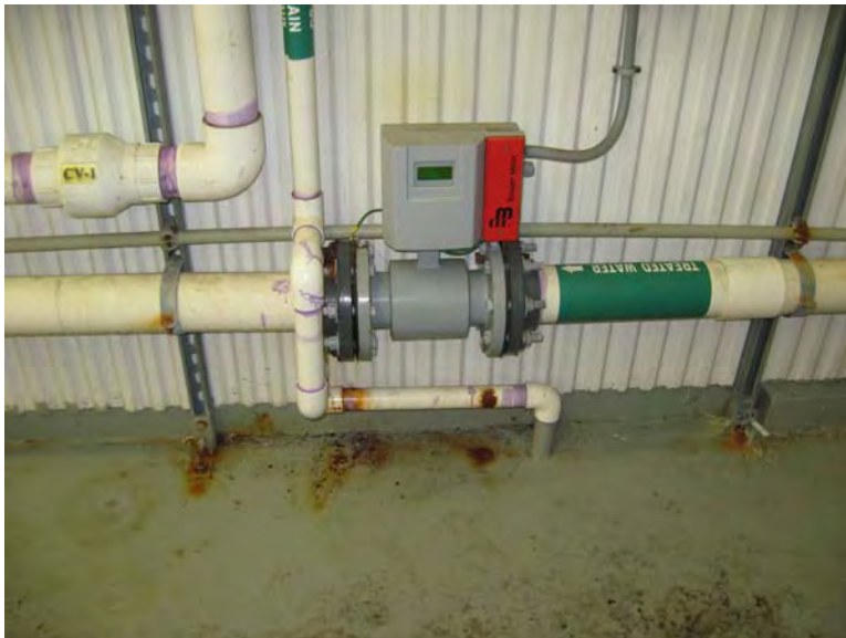
Drain Pipe In Front Of Flange
