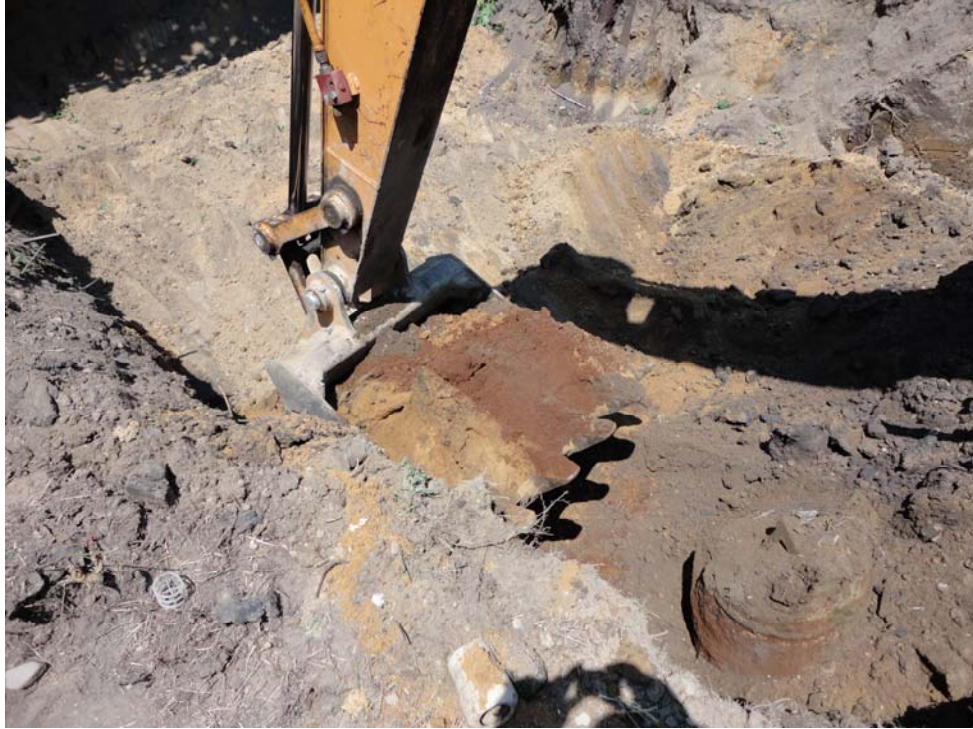
Drum/Drywell structure encountered in central portion of the IRM excavation area.
