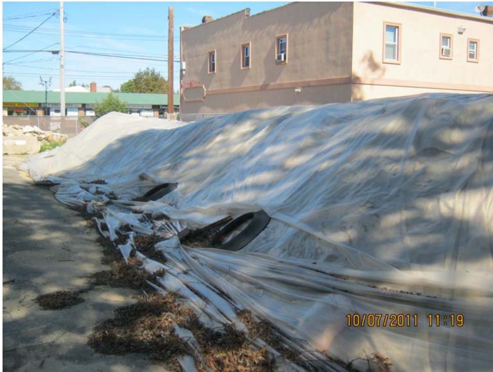
Completed ex-situ soil pile arrangement.
