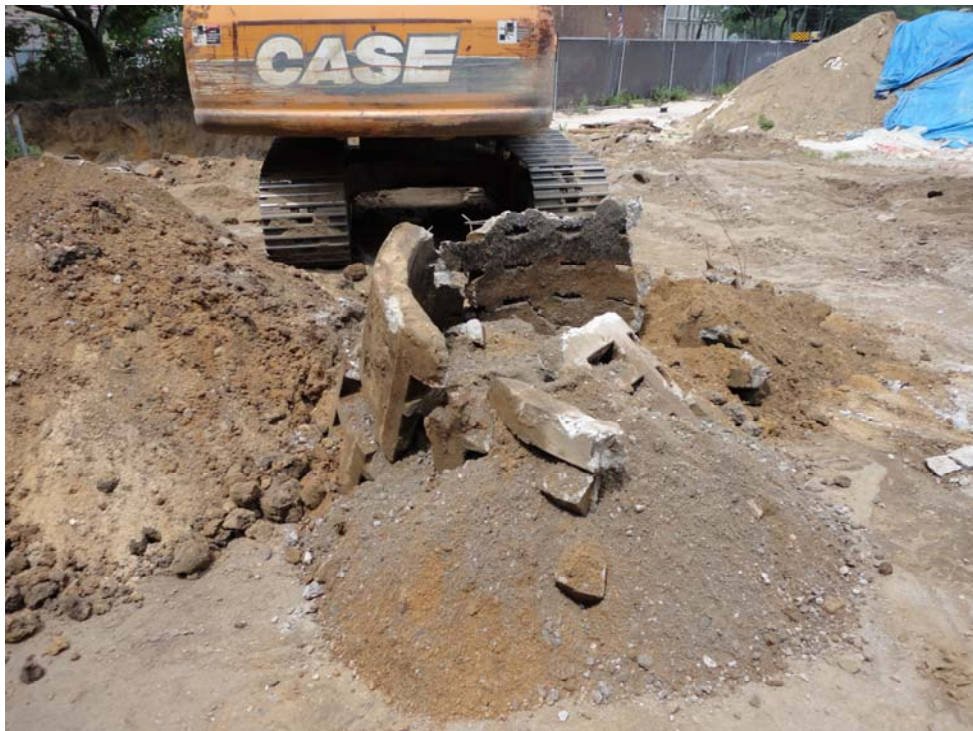
Removal of a Dry Well 3 structure to the east of the IRM excavation area.
