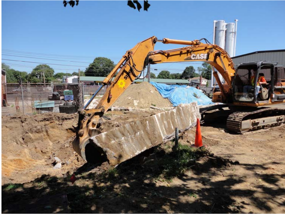
Removal of a below grade foundation wall from the eastern portion of the IRM excavation area.
