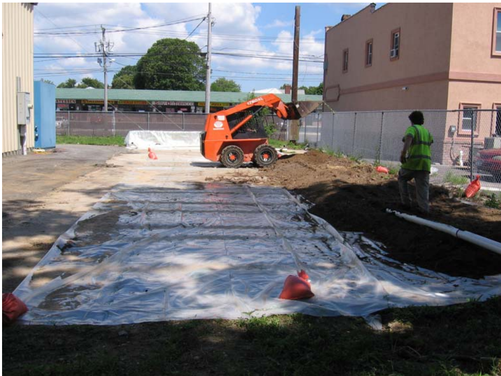
Loading of excavated soil at the soil staging area/ex-situ SVE system to the east of the treatment system building.
