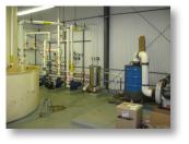
The GWE&TS consists of two, 8-inch diameter extraction wells; one located on-site in the southwest portion of the Site (RW-1), and one located off-site, approximately 1,500 feet southwest of the Site (RW-2). As per NYSDEC direction, extraction well RW-2 was shutdown in April 2010 due to historically low VOC concentrations, and is now being monitored on a quarterly basis. Extracted groundwater is conveyed to the GWE&TS building via
