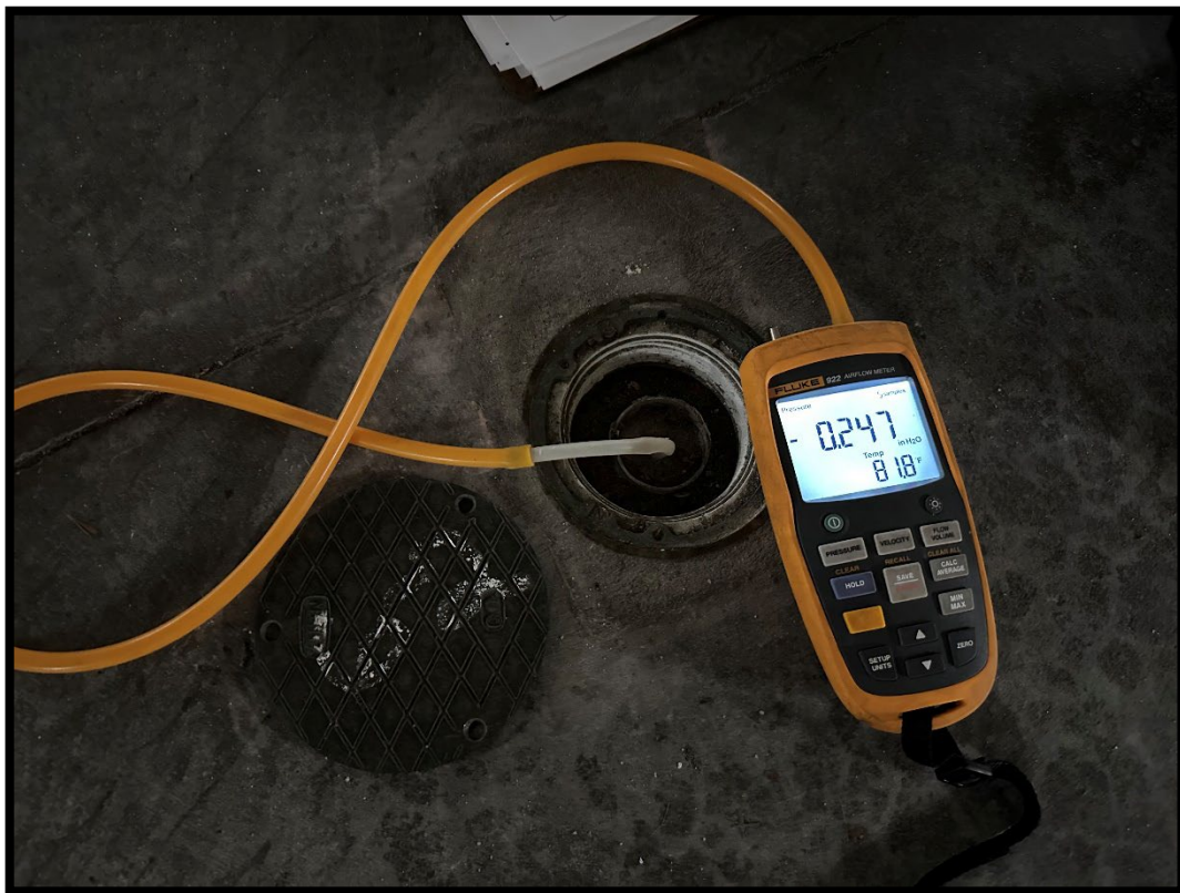
Photograph 12: View of MP 6-2 undergoing field pressure test.
