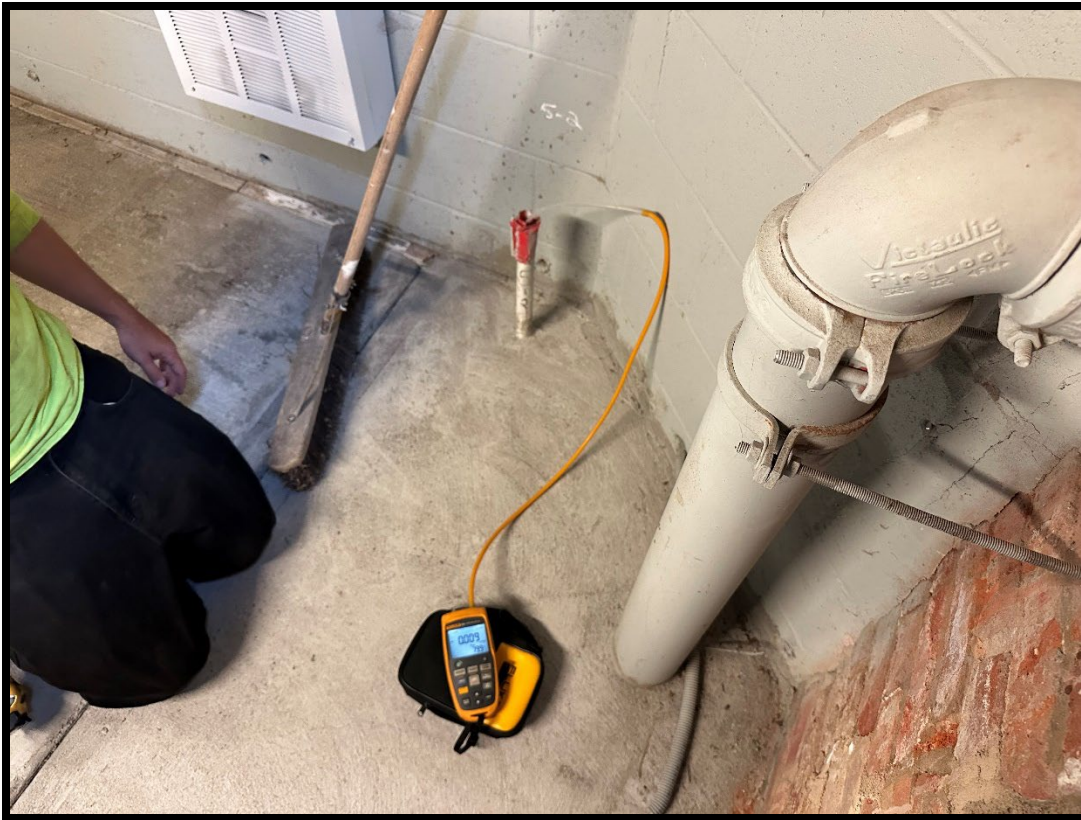
Photograph 7: View of field vacuum monitoring performed for MP 5-2.
