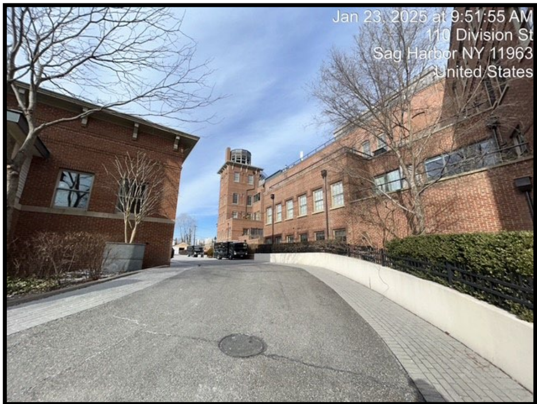
Photograph 20: View of southern asphalt ramp accessway for the Site.
