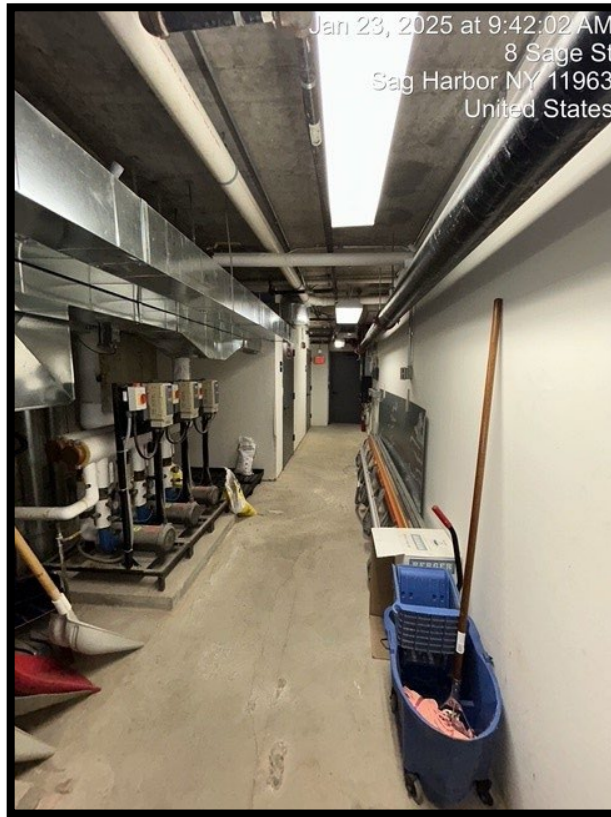
Photograph 23: Photo of maintenance room hallway during Site walk activities
