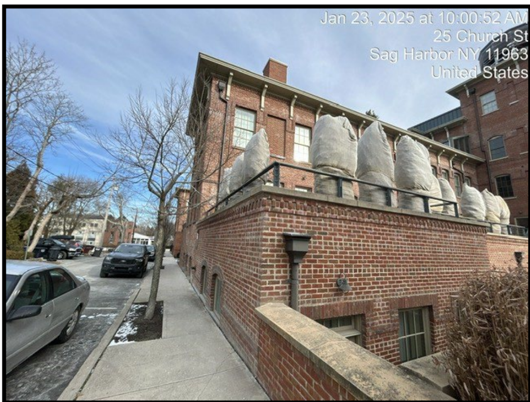
Photograph 18: Photo along the Site perimeter on Church St., facing north.
