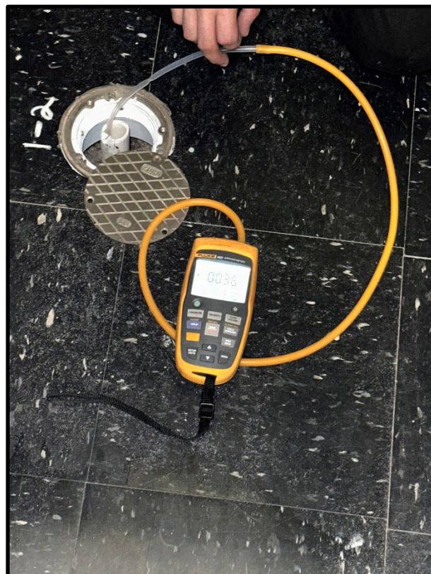
Photograph 6: View of MP 1-2 during vacuum monitoring.
