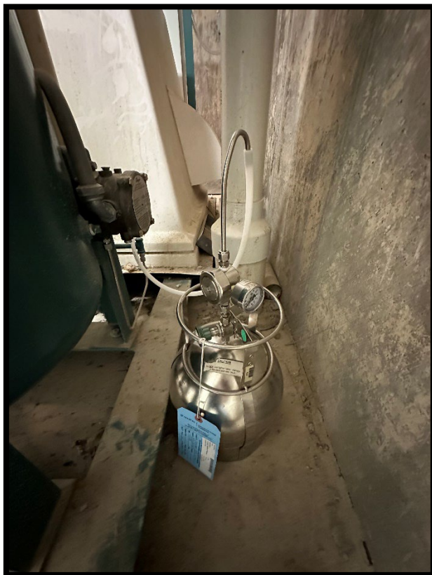
Photograph 9: View of effluent soil vapor sampling activities at garage SSDS Blower sampling port.
