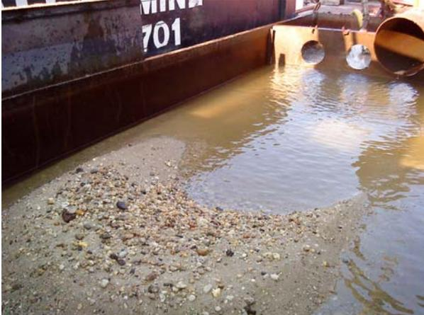
2. Sump to remove water from dumpster
