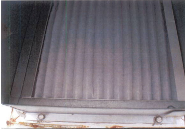
Picture 142 - The exterior filters on System #1 were changed.
