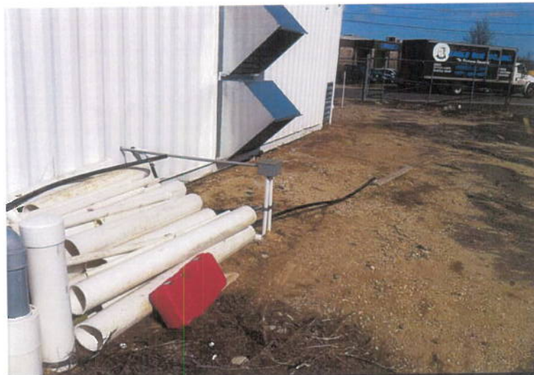
Picture 151 - The PVC piping on the side of System #2 was cut in preparation for removal.
