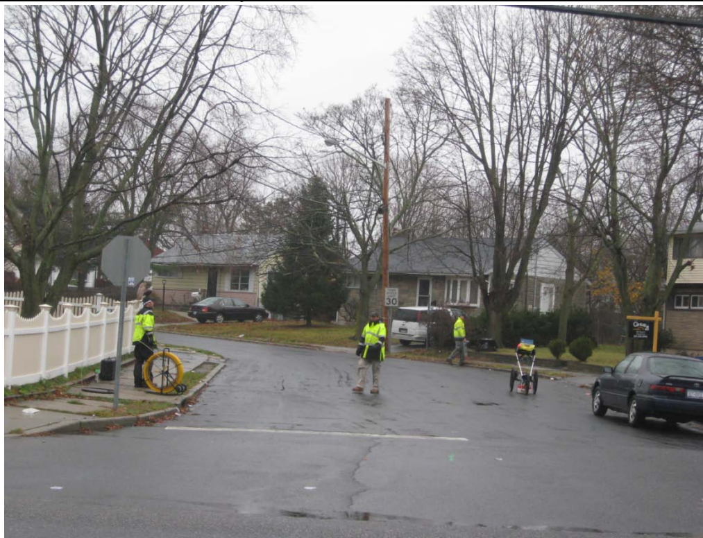
Underground Surveying conducting utility markouts on Benjoe St.
