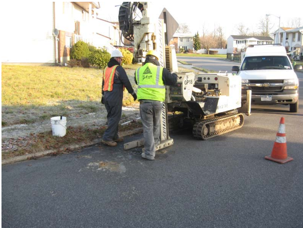
Zebra drilling MW-1D/1S.
