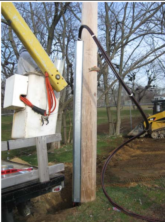
Gray Electric attaching supply lines to utility pole.
