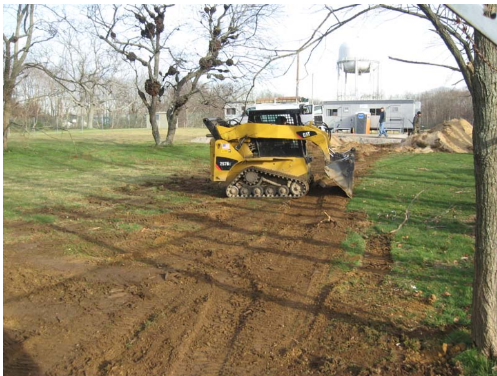
Michalowski backfilling/compacting trenched area.
