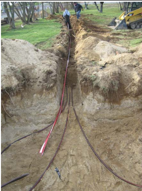
Gray Electric installing supply lines and caution tape.
