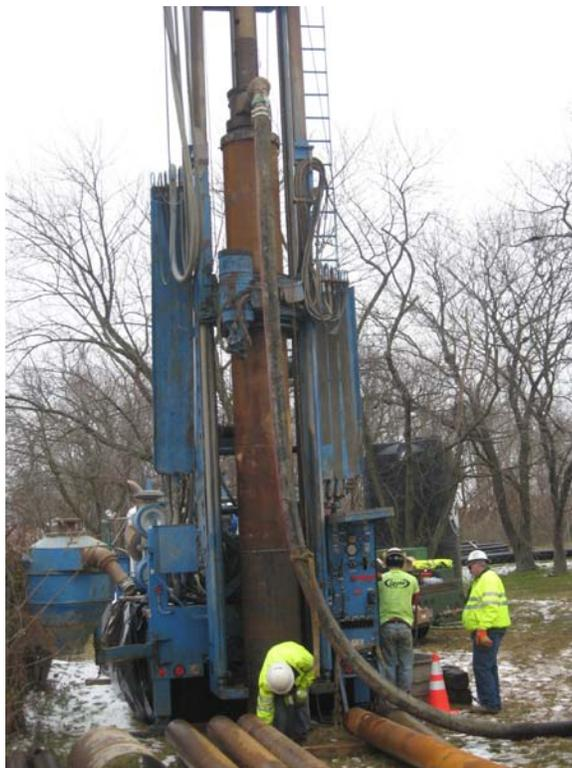
**View of drill string and outer casing at DDC-06, looking north.**
