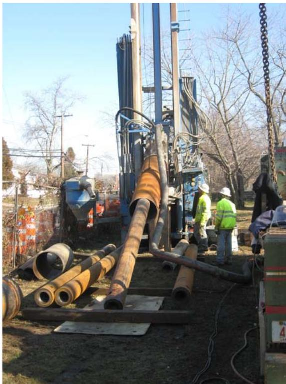
Layne assembling additional 24-in. diameter outer casing and drill string, looking north.
