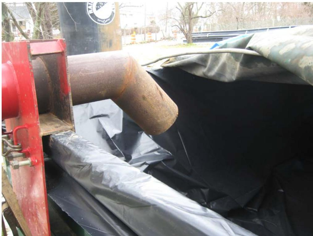
Outlet of drill cutting discharge pipe. Note: roll-off container lined with poly.
