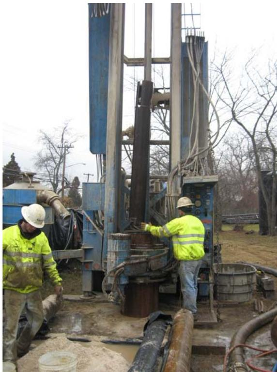
Layne removing material from outer casing via 6-in. steel bailer.
