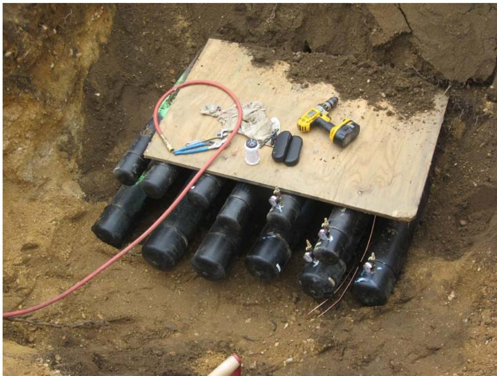
View of HDPE air lines and tapped pressure gauges.
