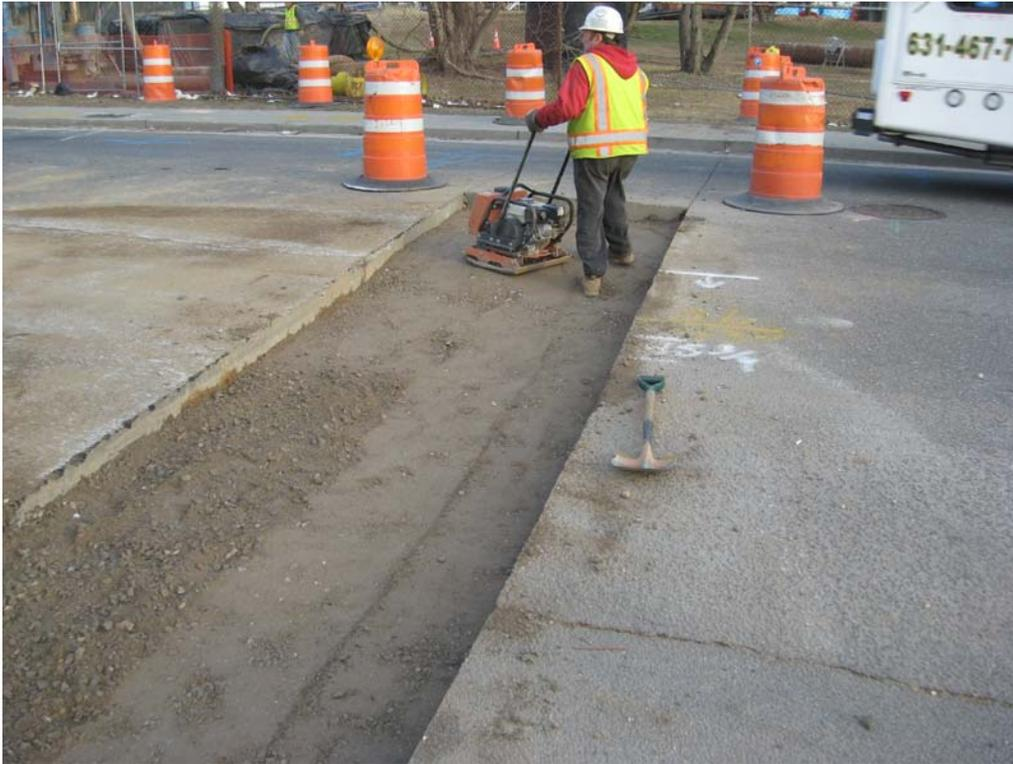
Posillico compacting recycled concrete material near centerline of Albany Ave.
