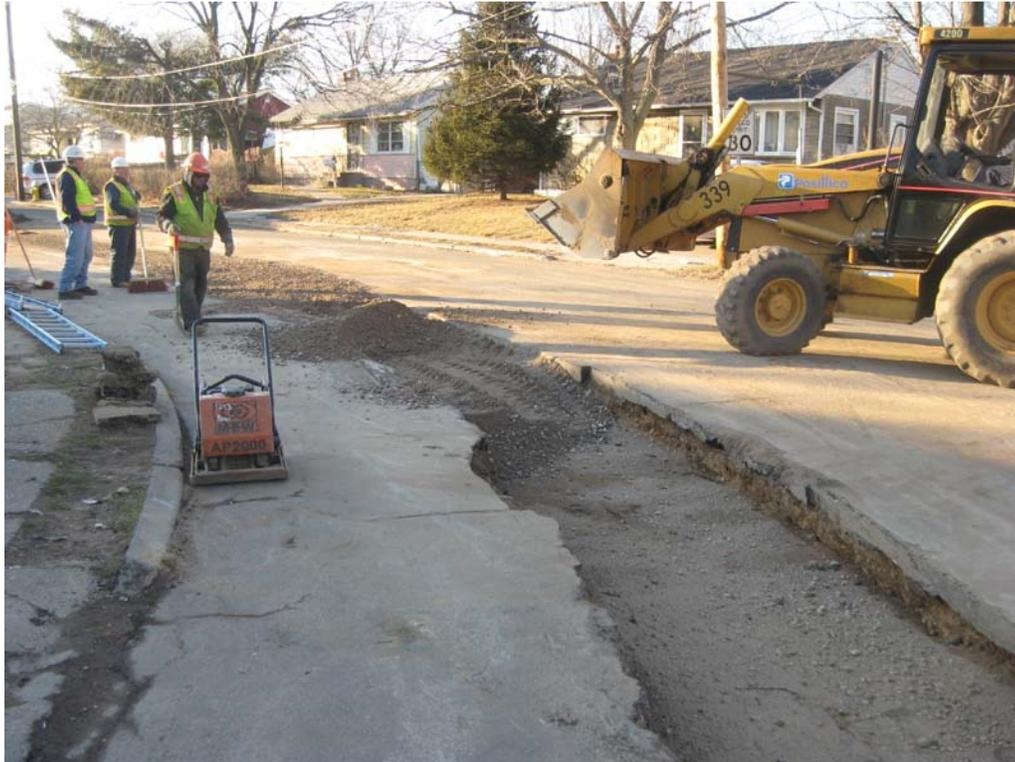
Posillico placing recycled concrete material along trench line for temporary road use.
