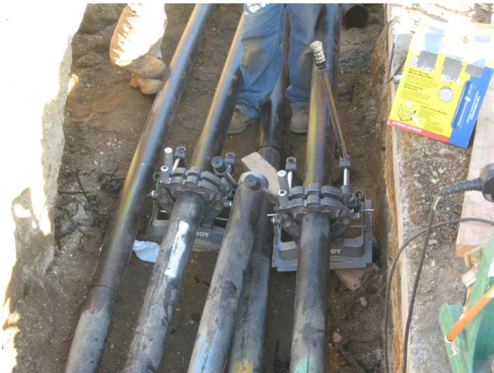
Posillico performing heat fusion welds on 4-in. lines.
