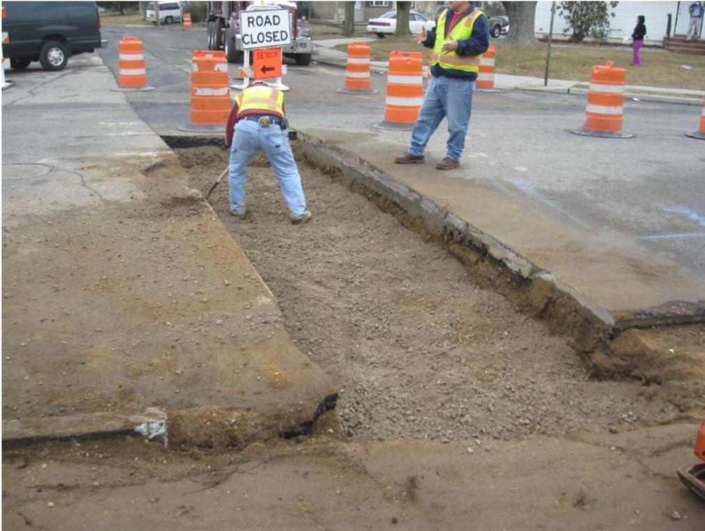
Posillico placing recycled concrete as road base material.
