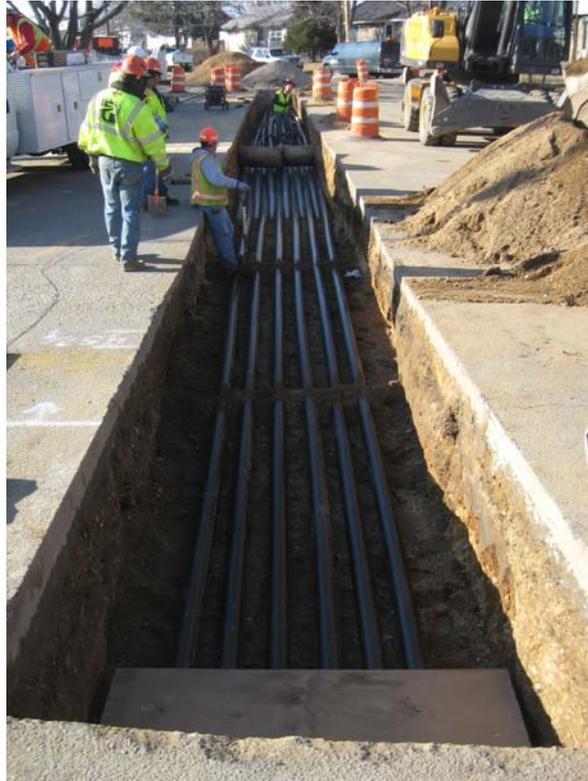
View of 4-in. air lines installed over 6-in. air lines and 2-in. gas line, looking west.
