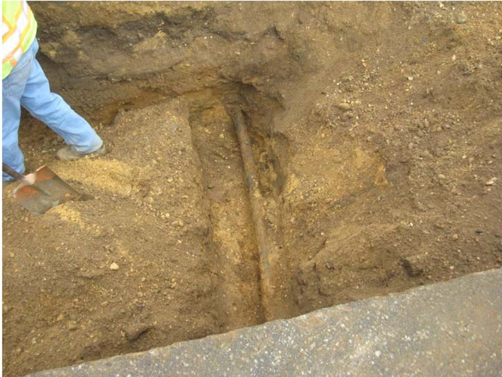
View of unmarked 2-in. gas line transecting trench line.
