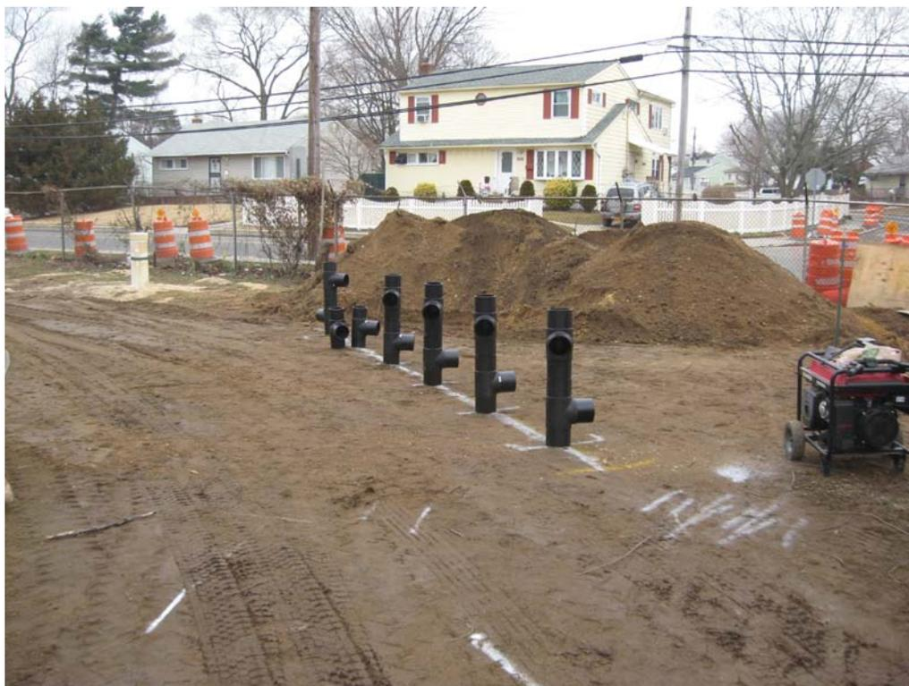
Prefabricated 6-in. sumps aligned at sump location.
