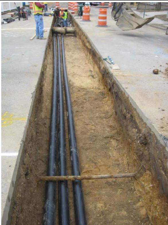
6-in. air lines installed under RCP and 2-in. gas line, looking west.
