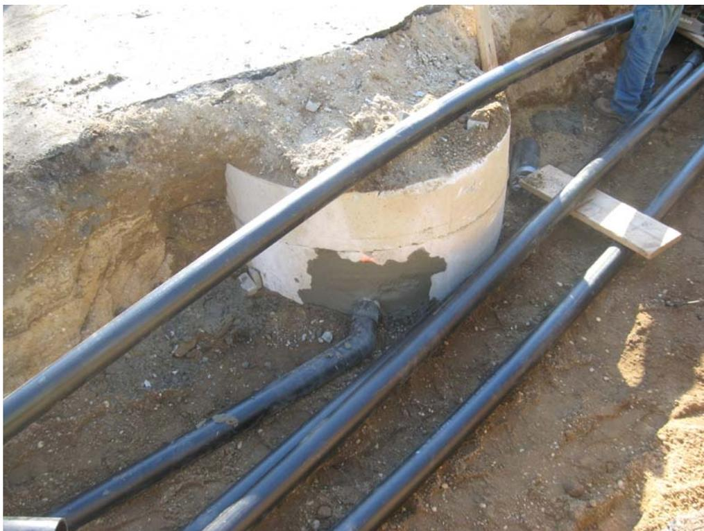
View of 4-in. supply line installed into DDC-07 vault.
