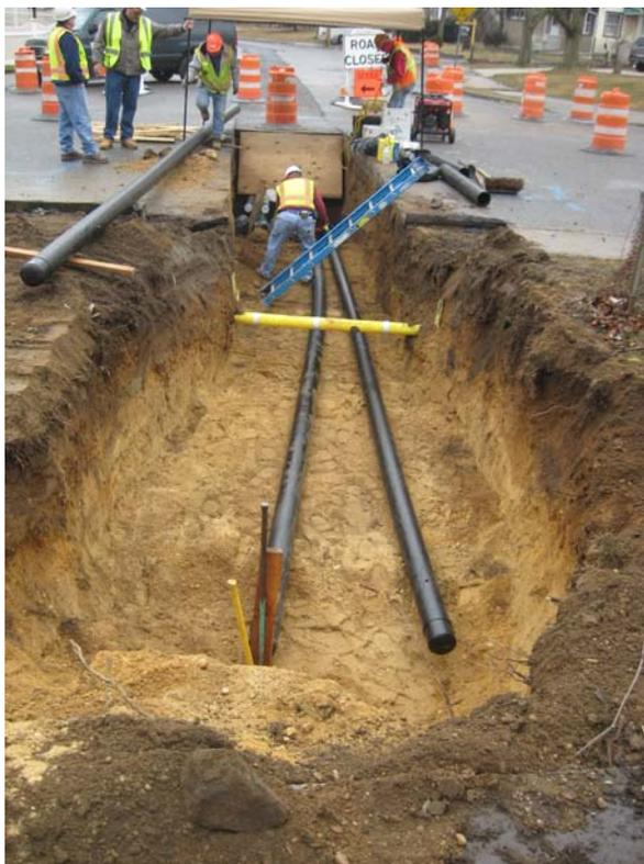
Posillico installing 6-in. air lines under gas main.
