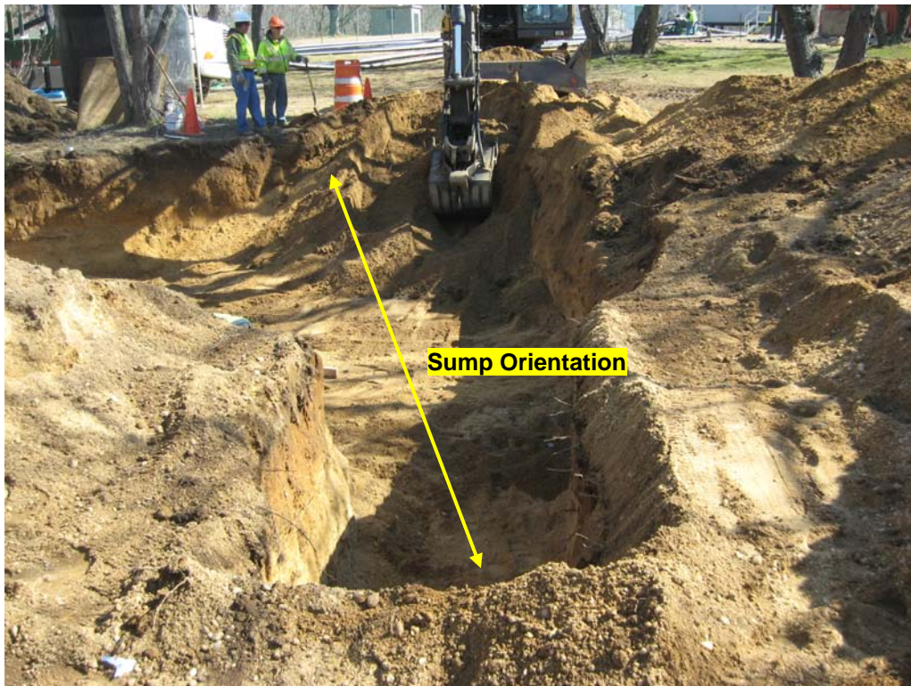
Posillico excavating airline trench and sump, standing at DDC-06 looking east.
