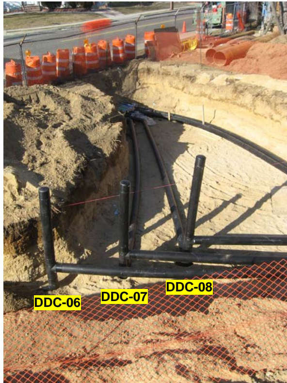
View of sump collection area.
