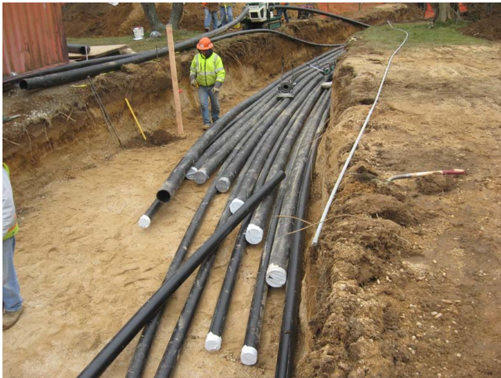
Posillico extending piping to treatment system pad, looking west.
