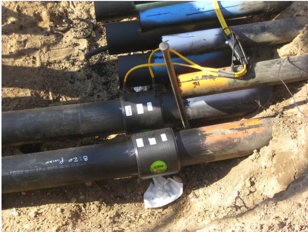
View of 6-in. Type A Couplers being connected via Electrofusion.
