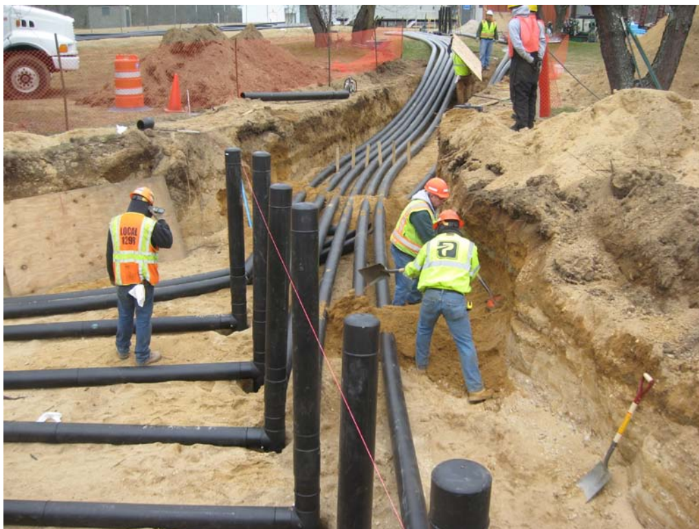
Posillico backfilling around 6-in. return lines.
