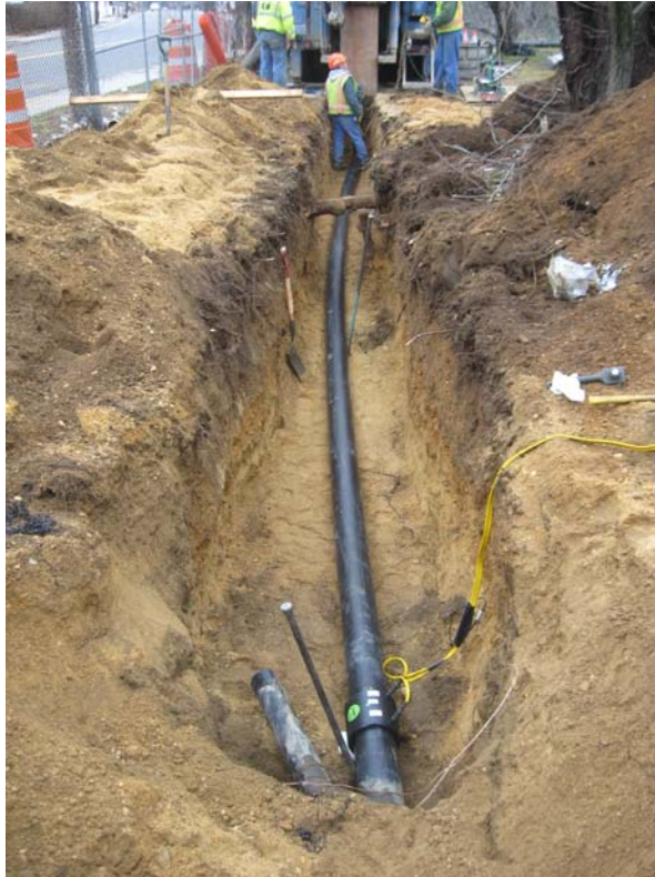
View of 6-in. line being installed to DDC-05, looking north.
