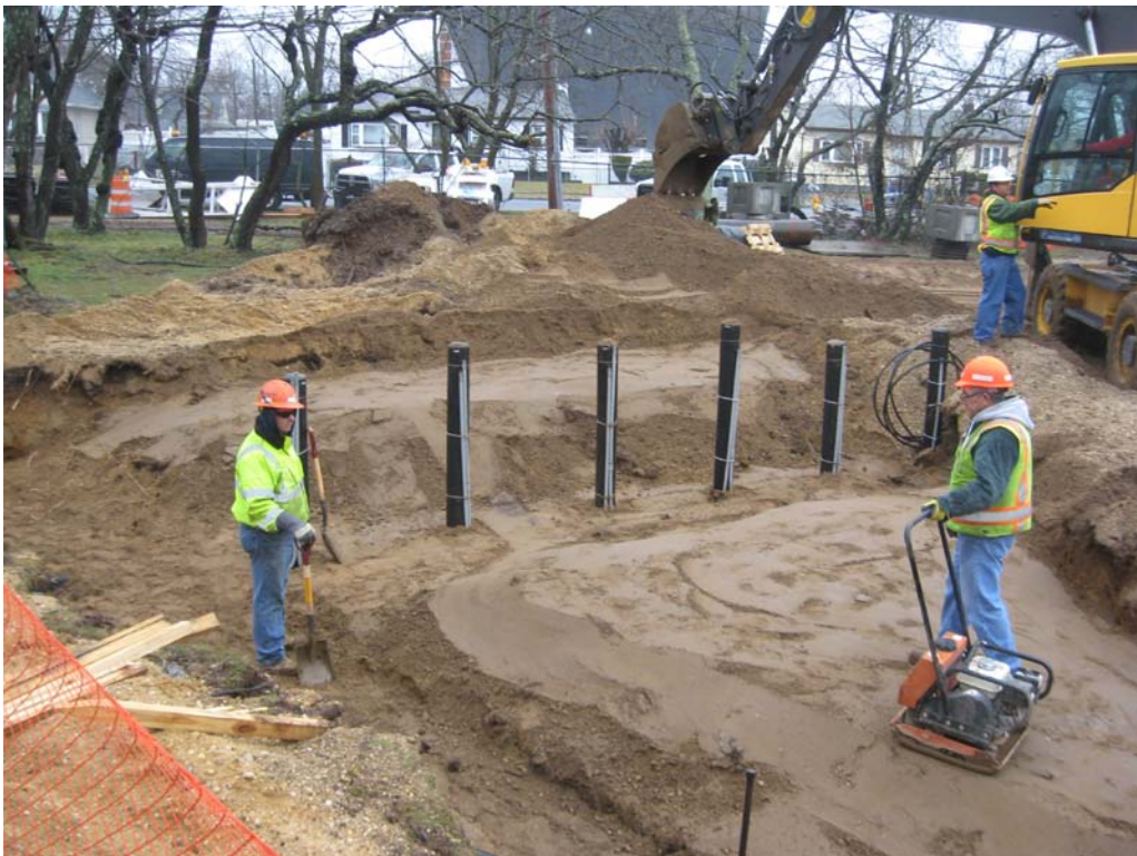
Posillico backfilling/compacting sump collection area.
