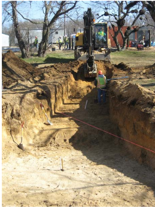
Airline trench extending east towards treatment system pad.
