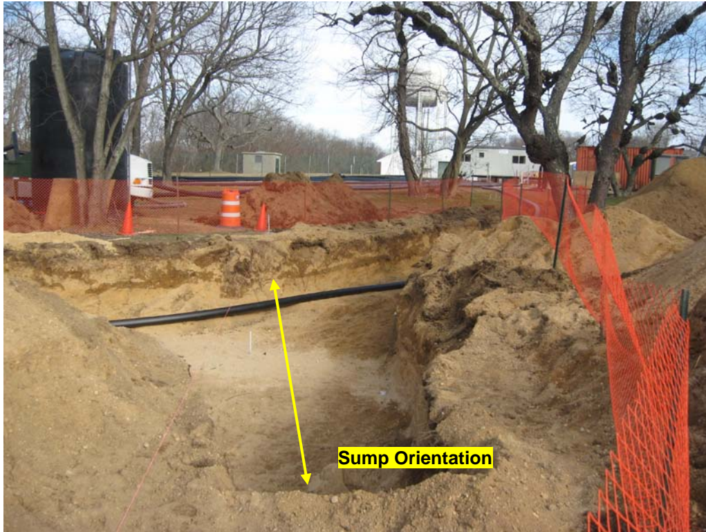
View of open excavation and orange fencing.
