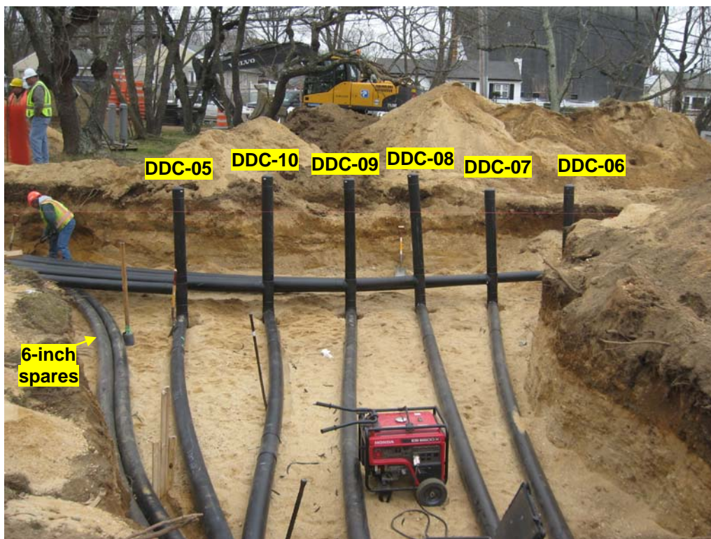
View of sump collection area, looking south.
