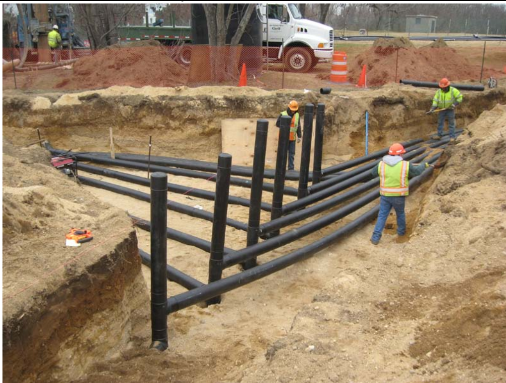
View of sump collection area, at DDC-06 looking northeast.
