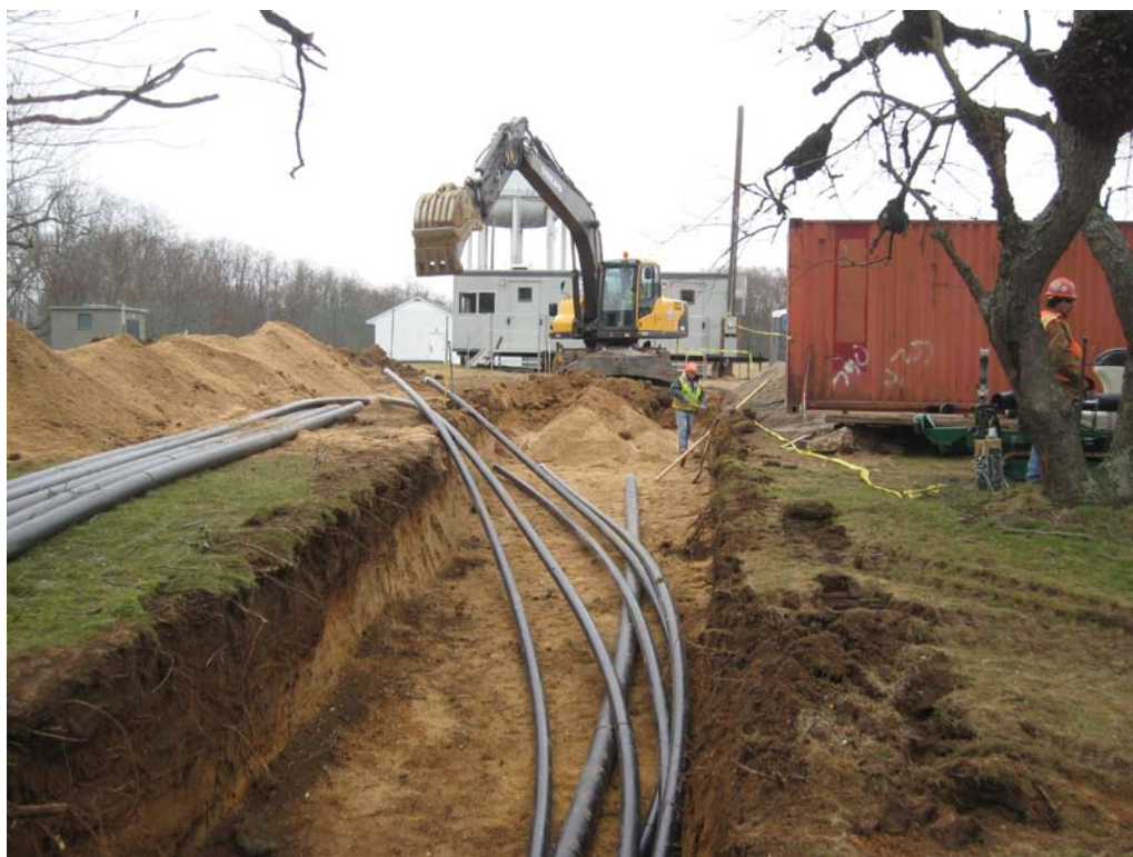
View of trench line to treatment system pad, looking east.
