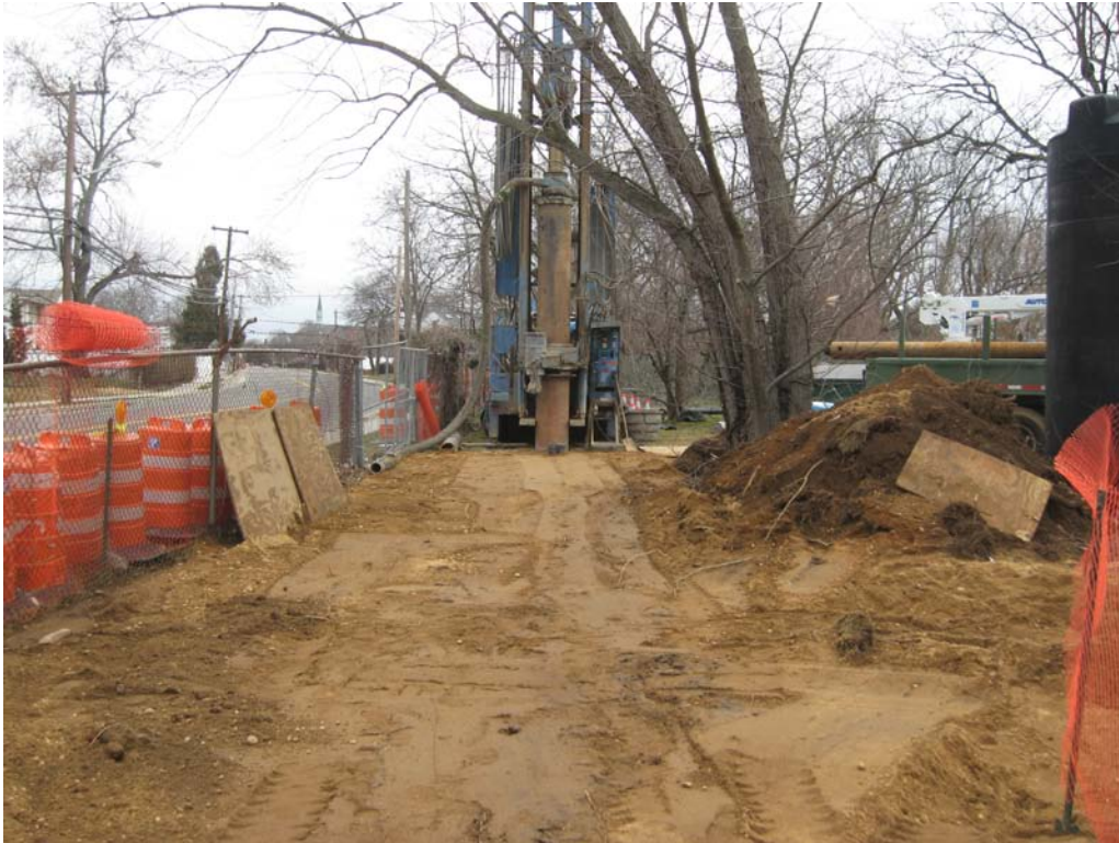
DDC-05 air line trench backfilled/compacted, looking north.
