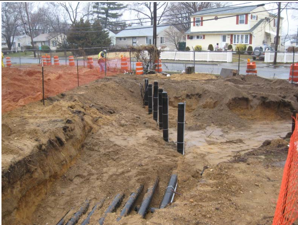
View of partially backfilled/compacted sump collection area.
