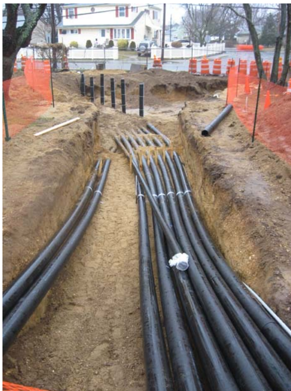
6-in. air return lines extending through trench line, looking west.
