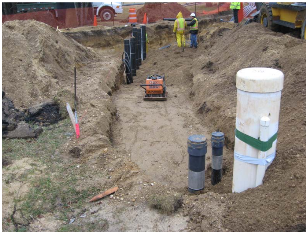
View of backfilled/compacted DDC-06 trench line.
