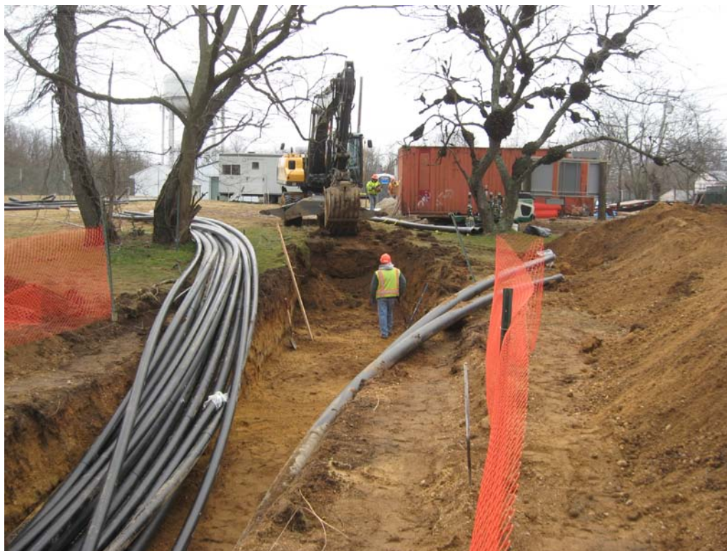
Posillico trenching to treatment system pad, looking east.
