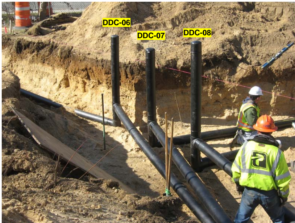
View of DDC-06, DDC-07, and DDC-08 sumps.
