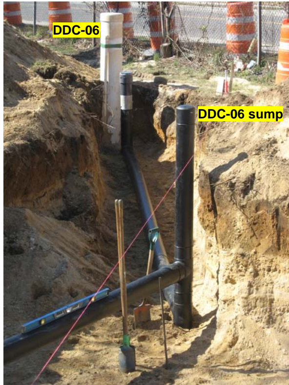
View of DDC-06 and associated sump.
