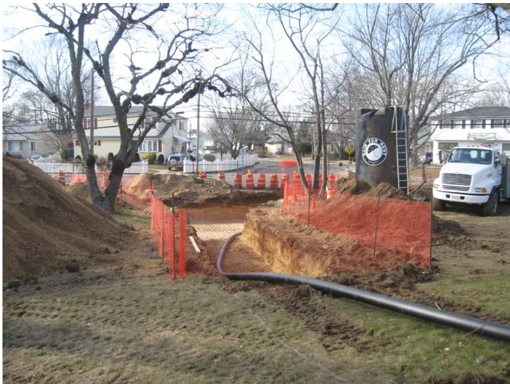
View of orange fencing around open excavation.
