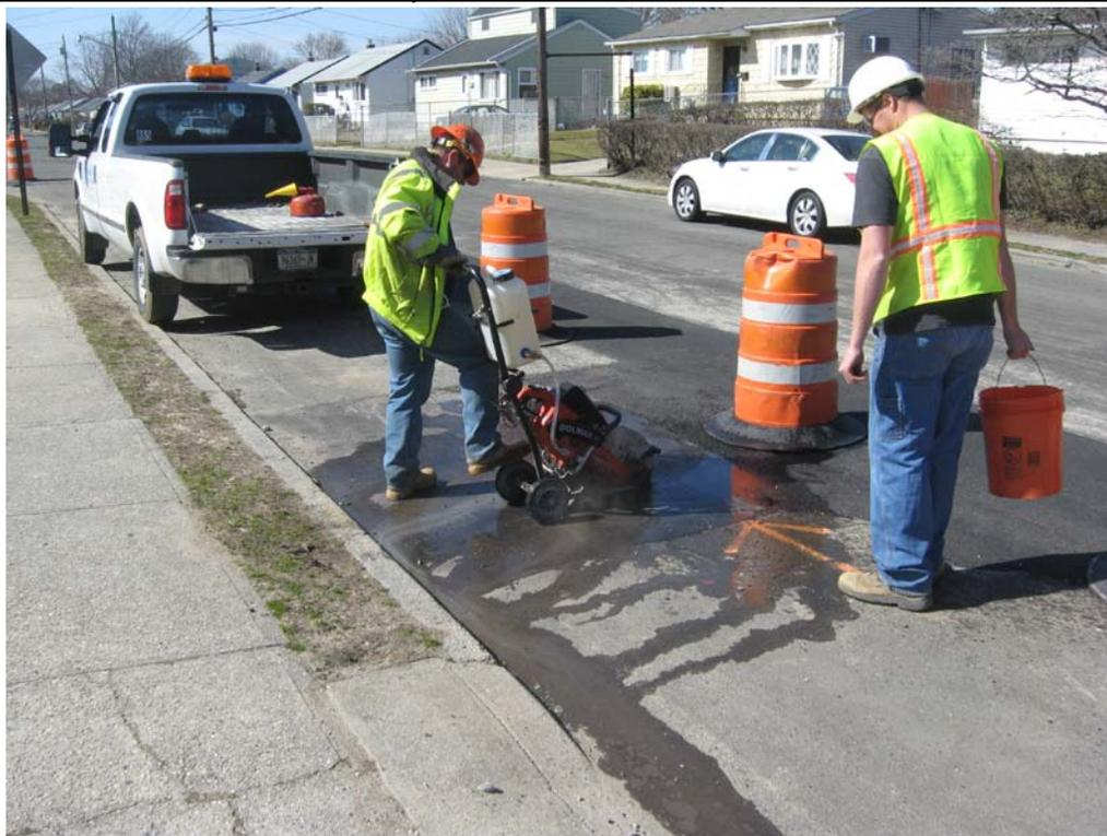
Posillico saw-cutting temporary asphalt patch at DDC-08.
