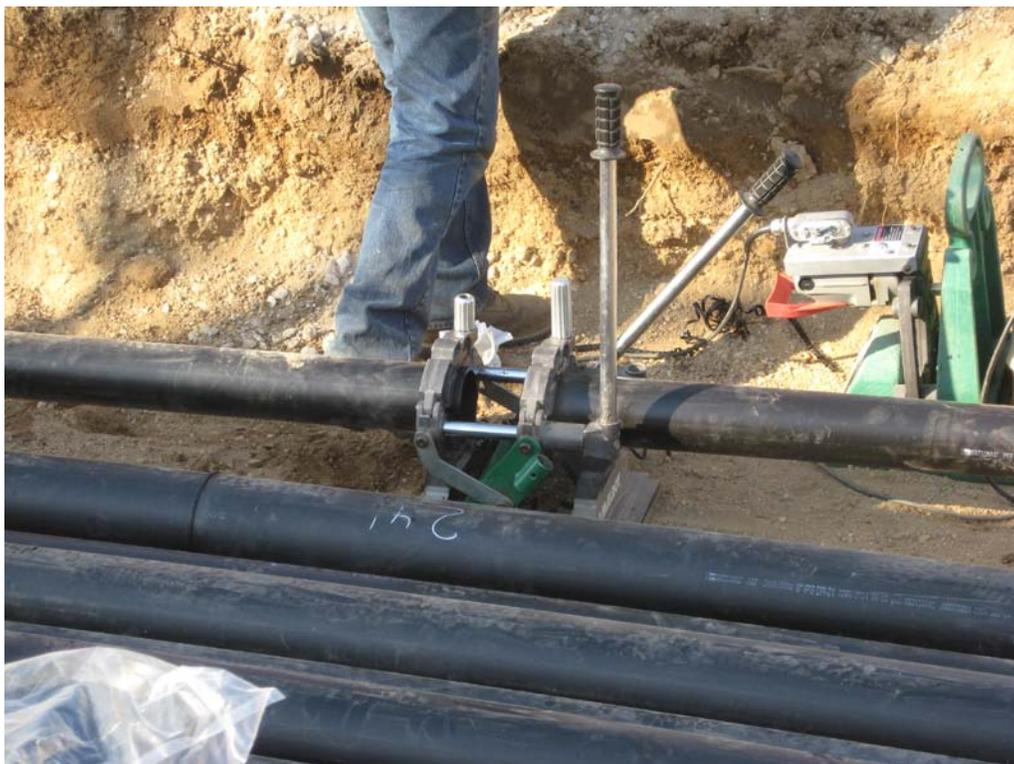
Heat fusion welding 4-in. pipe.
