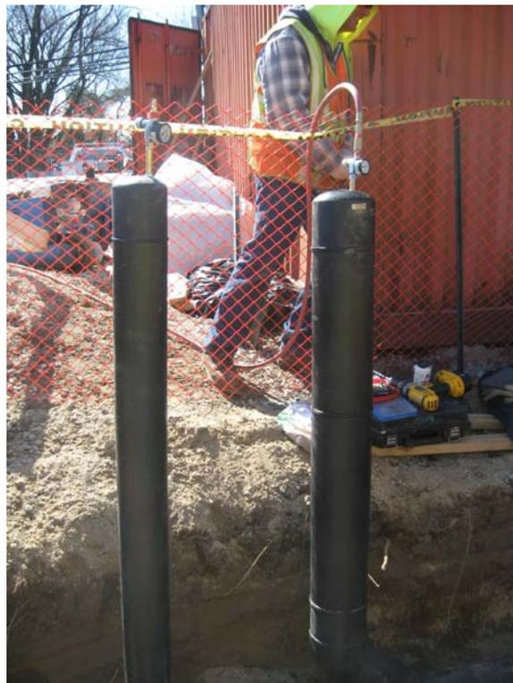
Posillico pressure testing piping.
