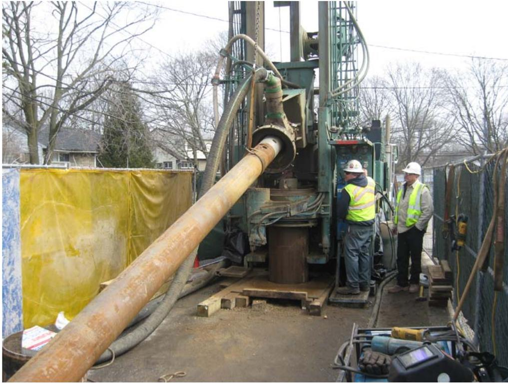
Layne threading additional drill rod at DDC-08.
