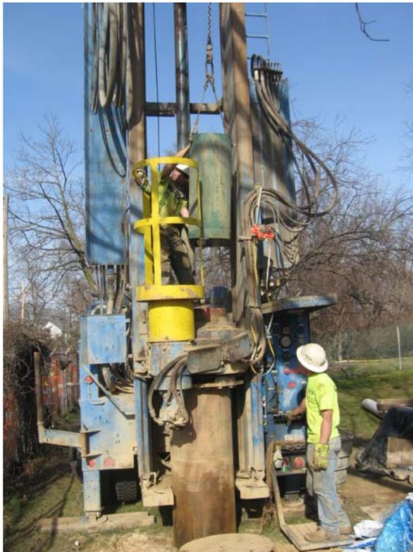
**Layne installing annular materials at DDC-05.**
