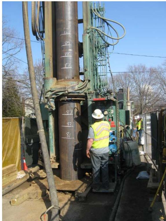
Layne drilling casing/drill string at DDC-08.
