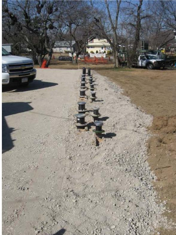
View of backfilled piping manifold area on north side of treatment system pad, looking west.
