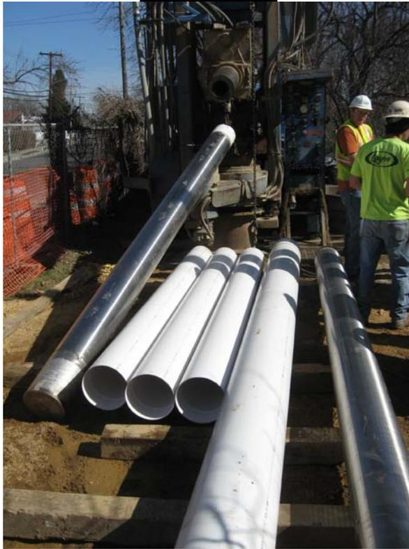
**Layne installing DDC-05 well screen and riser.**
