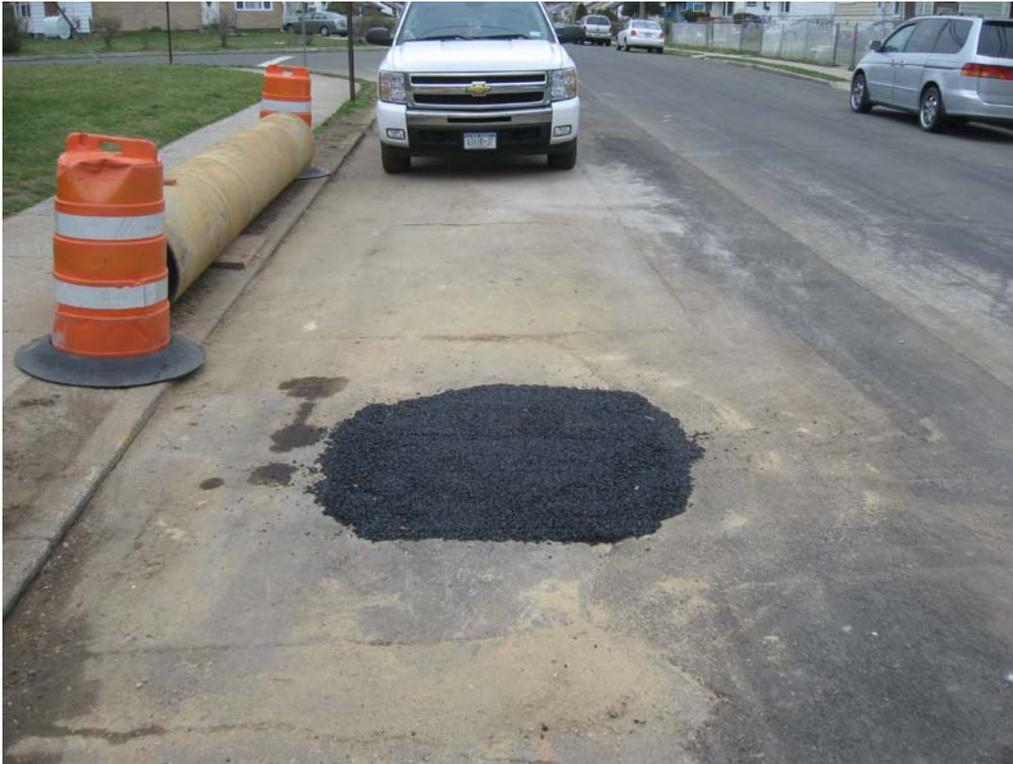
View of temporary asphalt patch over DDC-08 vault man-way.
