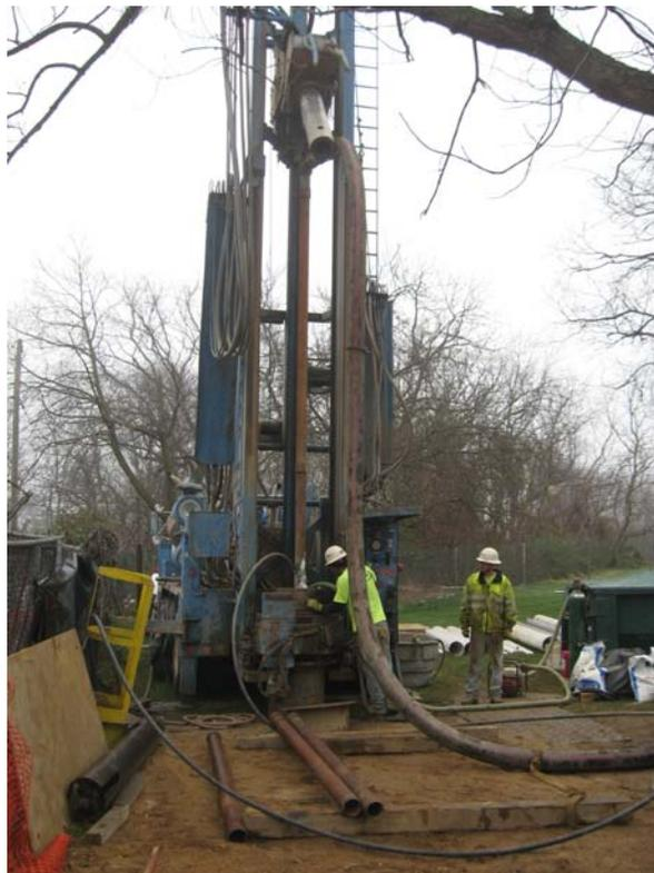
View of Layne bailing sediment from DDC-05 borehole.
