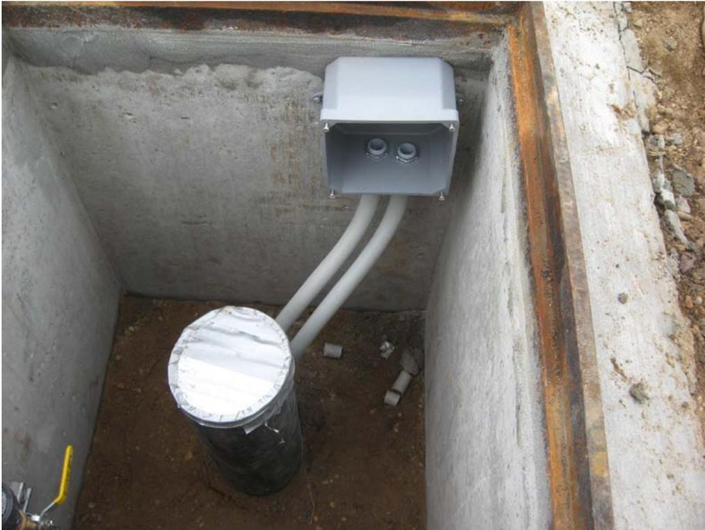
View of electrical box partially installed in sump vault.
