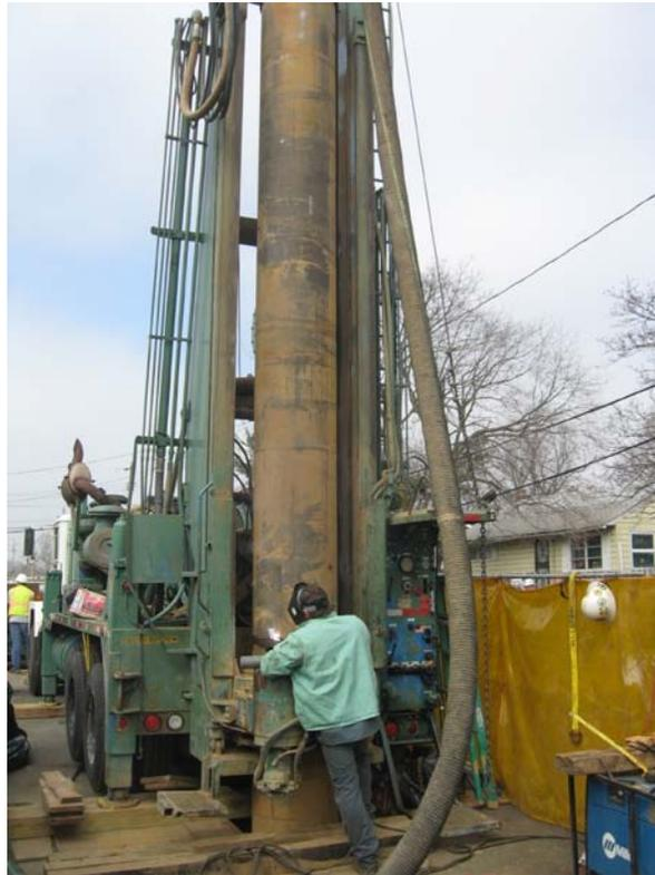
Layne welding additional section of casing at DDC-07.
