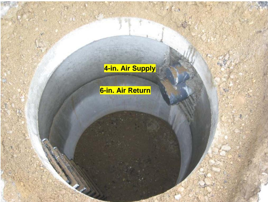
View of DDC-07 vault. Note: Treatment system air line piping.
