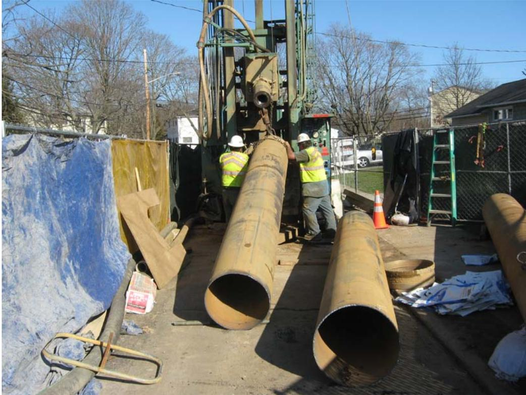
**Layne removing outer casing at DDC-08.**
