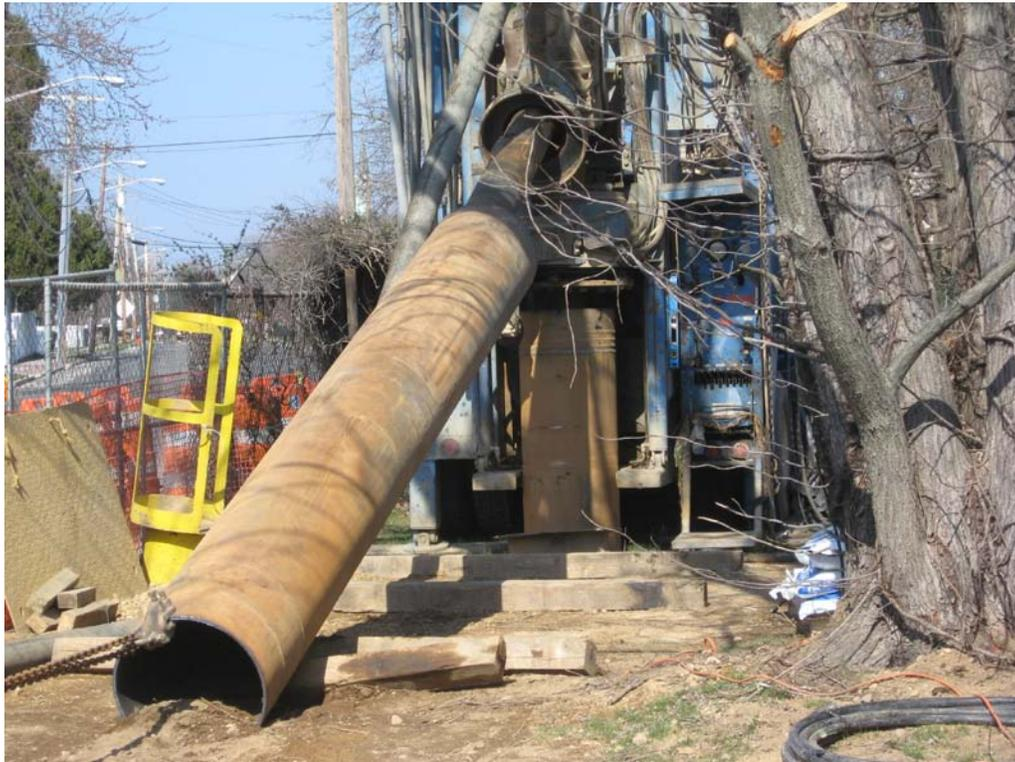
Layne installing additional section of outer casing at DDC-05.
