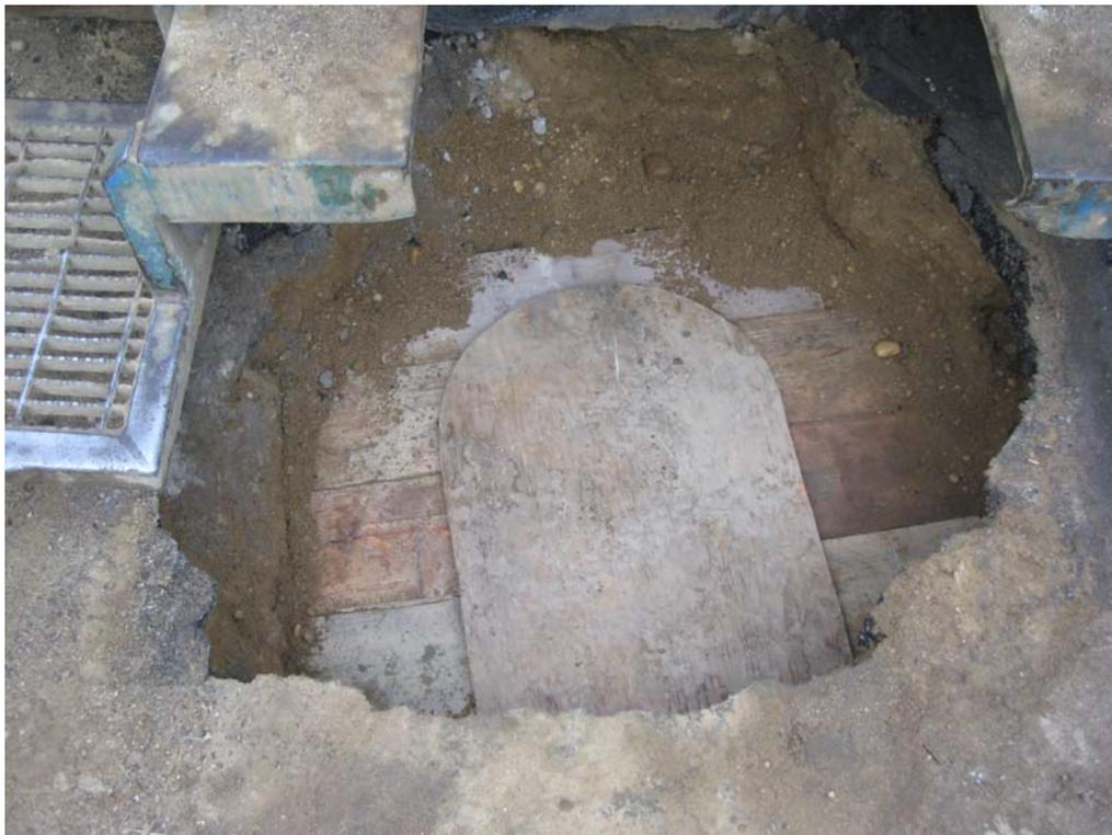
Timber used to seal DDC-08 man-way.
