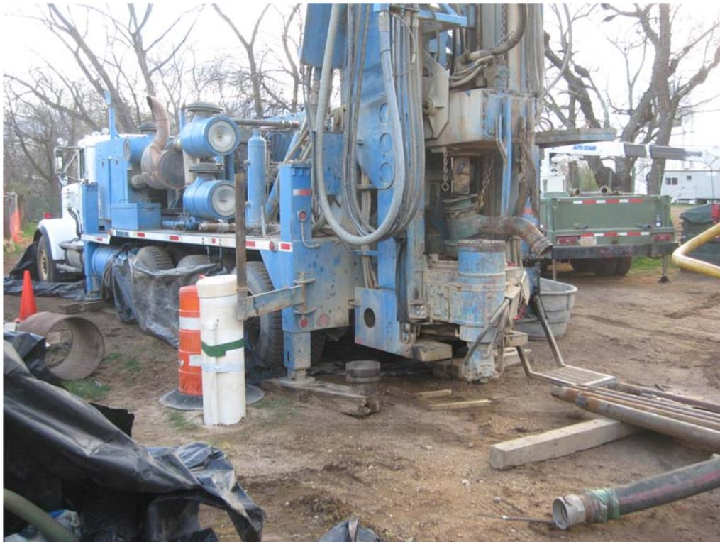
Layne mobilizing rig to install DDC-06 piezometers (7-ft east of DDC-06).
