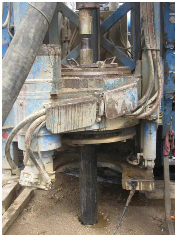
**View of 6-inch outer diameter casing and drill string installing DDC-06 piezometer borehole.**
