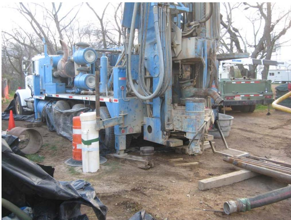
**Drill rig mobilized for DDC-06 piezometer re-installation.**
