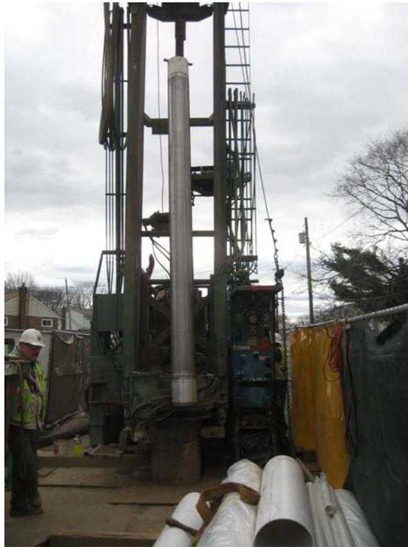
Layne installing lower screen at DDC-07.
