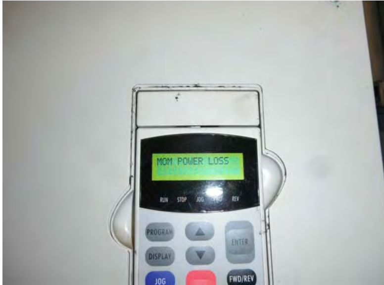
Picture 387 - View of the variable frequency drive (VFD) for System #2, with the alarm of, "Mom Power Loss".
