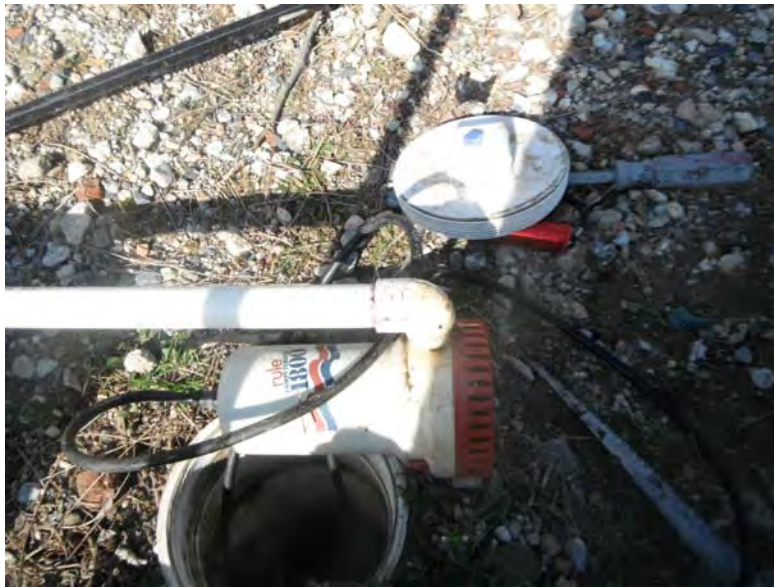
Picture 539 - The sump pump associated with DDC-3 was observed to be consistently running, even if not submerged in water.
