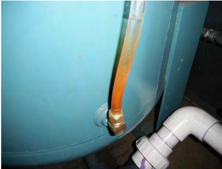
Picture 390 - Five inches of water was noted in the site glass of the knock-out tank in System #2.
