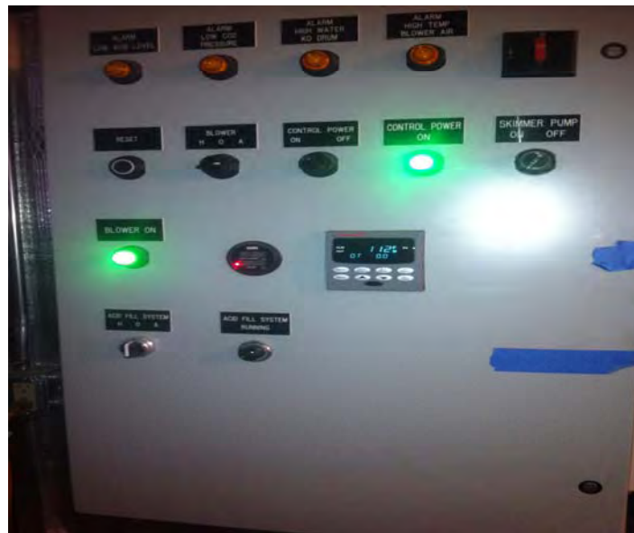
Picture 358 - View of the control panel associated with System #1. No alarms were tripped upon arrival.
