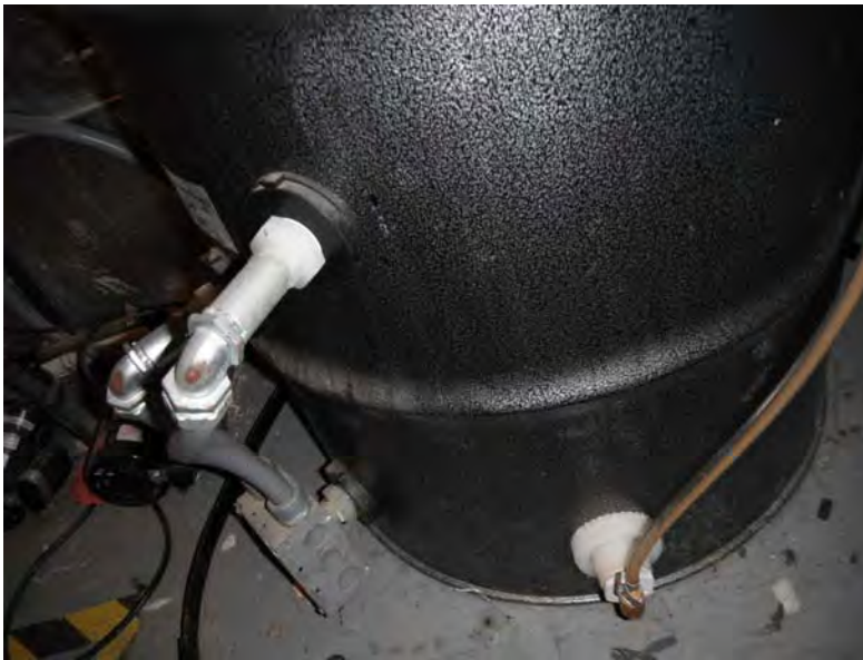
Picture 367 - View of a knock-out tank associated with System #1. No water was observed within the site glass.
