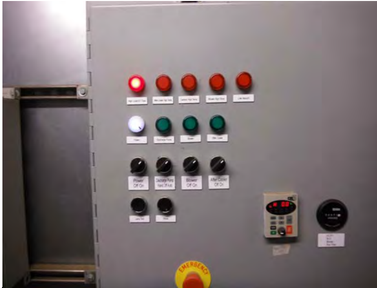
Picture 387 - The "High Level K.O. Tank" alarm was noted to be triggered upon arrival.
