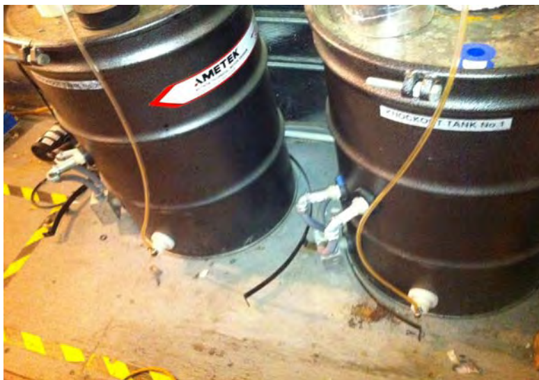
Picture 351 - View of the two Knock-out Drums associated with System #1. No water was detected in either site glass.
