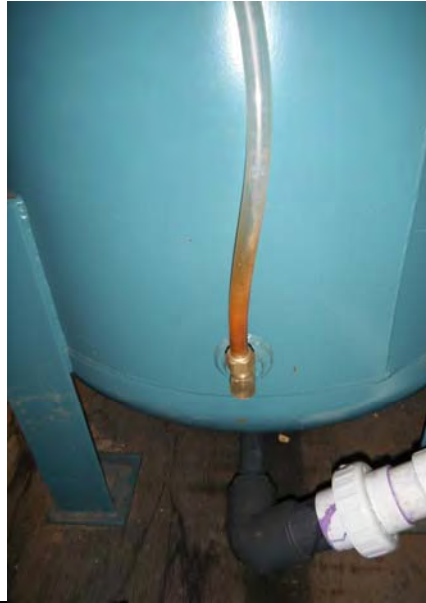
Picture 480 - No water was detected within the site glass of the KO tank prior to restating the system.
