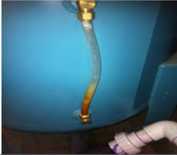
Picture 437 - No water was detected within site-glass of the K.O. Tank in the System #2 shed.
