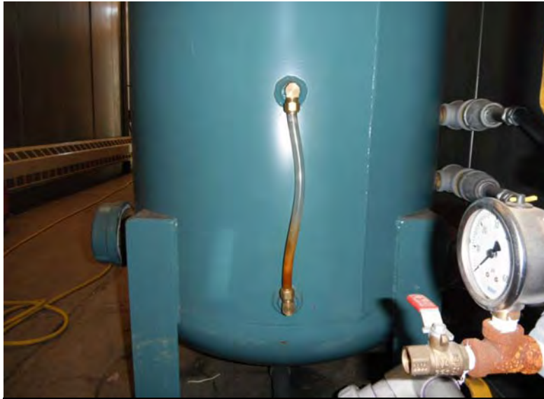
Picture 391 - No water was noted within K.O. tank associated with System #2 upon arrival.
