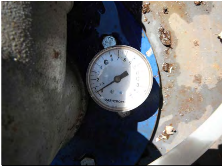
Picture 401 - View of the pressure gauge attached to DDC-4. The pressure went down to 0.4 PSI after the system was turned off, due to a previous pressure reading of 1.3 PSI, when the system was on.
