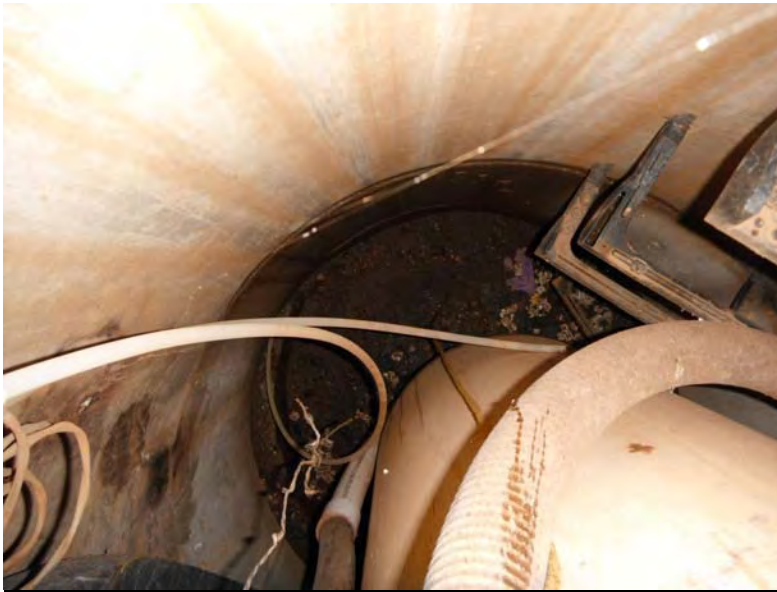
Picture 355 - While System #1 was off, no water was observed pooling outside the casing of DDC-1.
