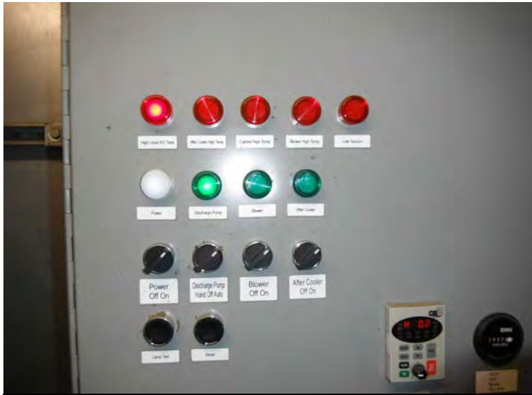
Picture 505 - System #2 was off upon arrival, with a "High Level KO Tank" alarm.
