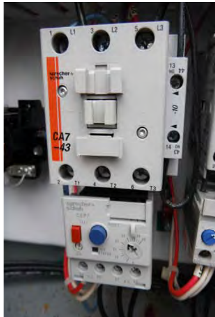
Picture 1449 - The Control Starter, along with the heating control for the blower needs to be replaced for the SVE System.
