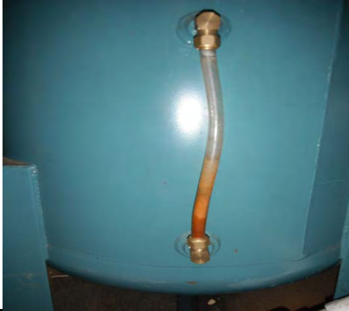
Picture 530 - The knock-out tank in System #2 had no water within its site-glass.
