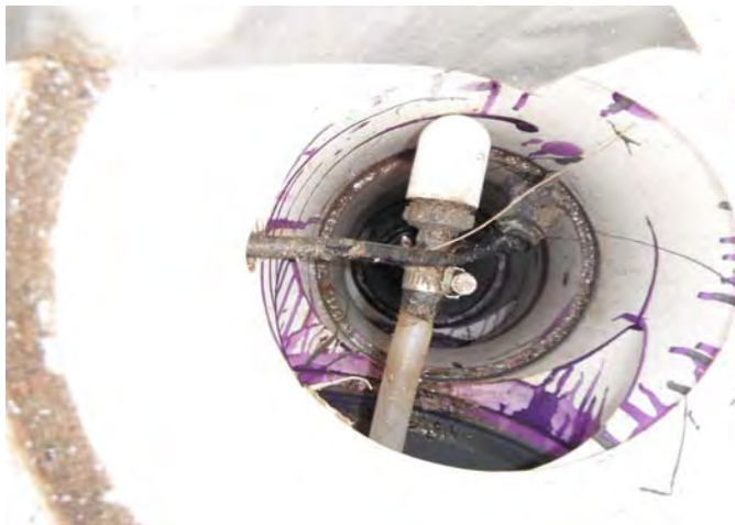
Picture 526 - The sump associated with DDC-4 was purged after it was observed to contain over a foot of water from within.
