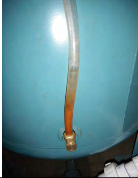
Picture 521 - Five inches of water was observed in the site glass of the knock-out tank in System #2, upon arrival.
