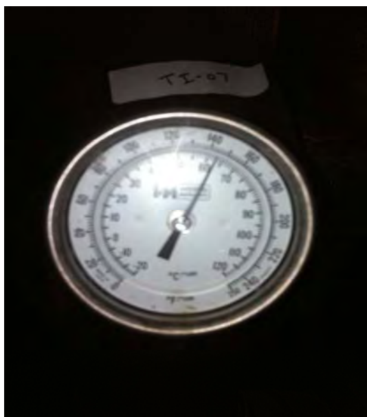
Picture 362 - View of temperature gauge TI-07 reading 64.0 degrees Celsius.
