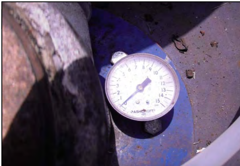
P6280026 - View of pressure gauge on well head of DDC-4 associated with System #2.
