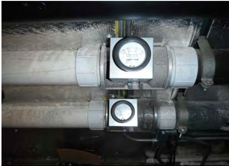
Picture 268 - View of FI-01 and FI-02 gauges reading 243 SCFM and 225 SCFM, respectively.
