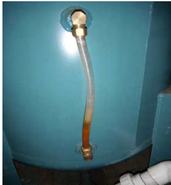
Picture 479 - About two and 3/8 inches of water was noted within the knock-out tank's site glass in System #2.
