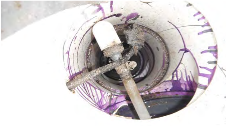
Picture 529 - The sump associated with DDC-3 was observed to only contain a half inch of water.
