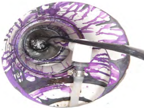
Picture 536 - The sump associated to DDC-4 was observed to contain over a foot of water. This water was pumped out in an effort to reduce the amount of water within return pipes.
