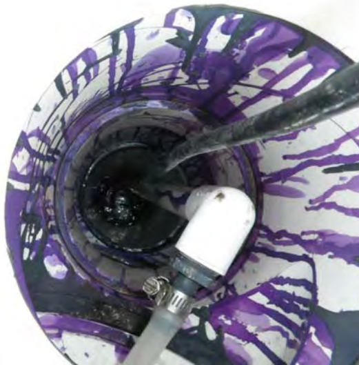
Picture 410 - Over a foot of water was noted within the sump associated with DDC-2.
