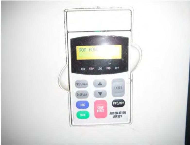
Picture 1784 - View of System #2's Variable Frequency Drive (VFD) with a, "Mom Power Loss" alarm.
