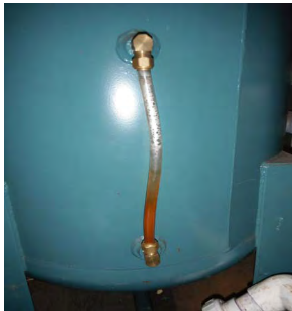
Picture 532 - The knock-out tank within System #2 was observed to contain 5.5-inches of water within the site glass upon arrival. During the O&M visit the water was completely discharged from the tank to the DDC-3 well.
