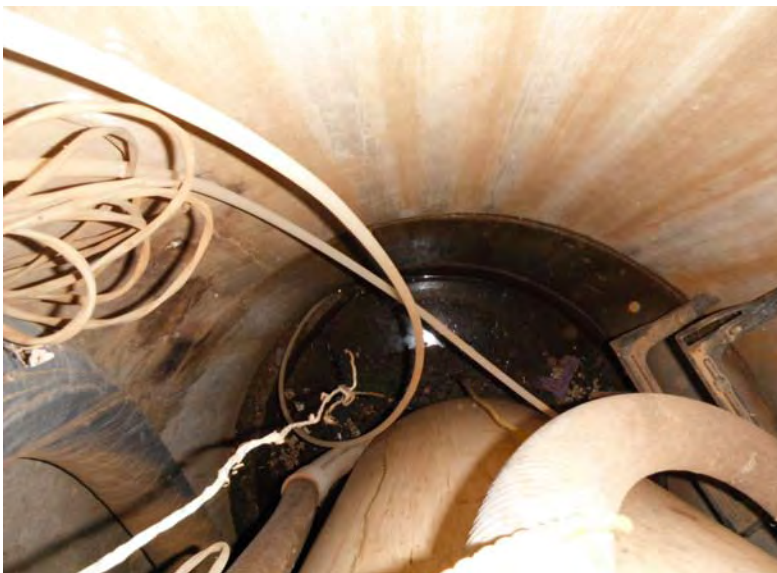
Picture 401 - View of pooled water that accumulated after System #1 was turned on.
