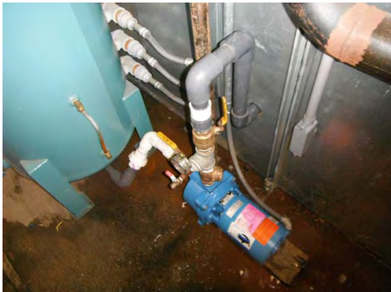
Picture 528 - The knock-out pump was replaced and the piping reconnected within the System #2 shed.
