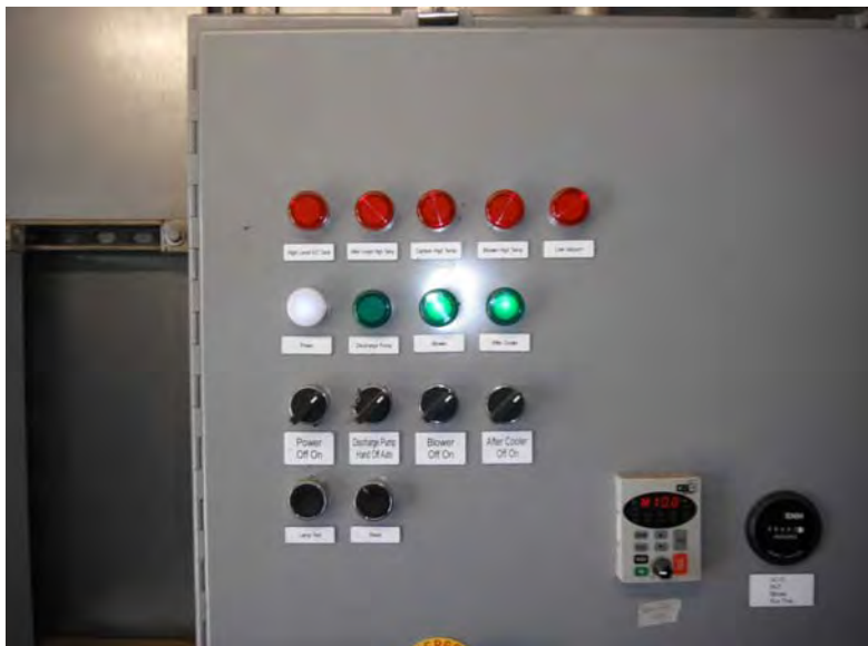
Picture 387 - View of System #2 control panel, showing no alarms triggered upon arrival.
