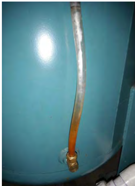
Picture 484 - 1-inch of water was observed within site glass once System #2 was restarted.
