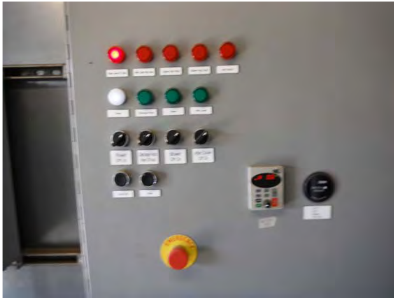
Picture 415 - View of System #2 control panel, showing, "High Level K.O." alarm triggered.
