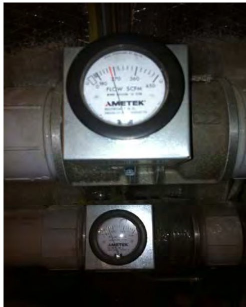
Picture 356 - View of FI-01 and FI-02 flow gauges associated with System #1.
