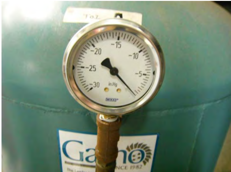
Picture 532 - View of T01, vacuum gauge attached to knock-out tank within System #2, reading -0.5 in.Hg.
