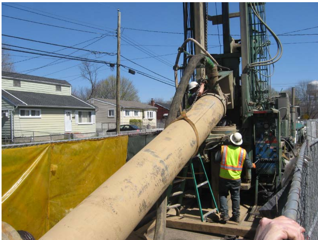
Layne attaching additional outer casing at DDC-10.
