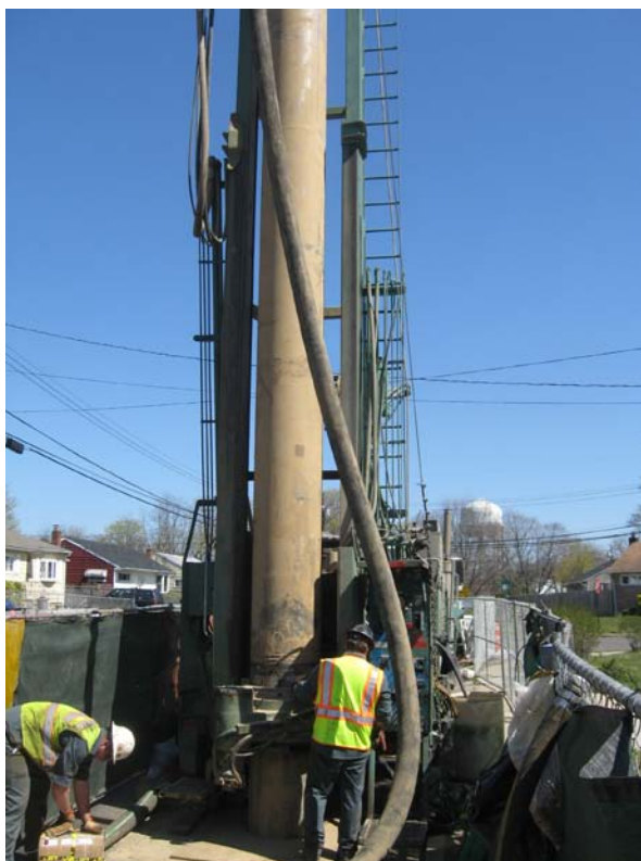
Layne advancing outer casing at DDC-10.
