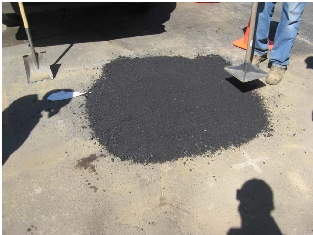
AECOM installing temporary asphalt patch at DDC-07.
