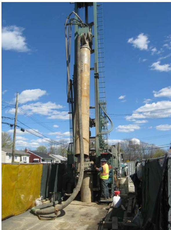
Layne attaching additional outer casing at DDC-10.
