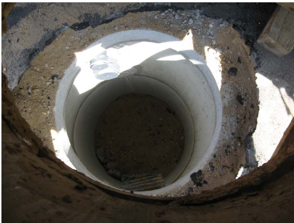
View of DDC-10 vault. Note: 4 in. and 6 in. airline piping entering vault.
