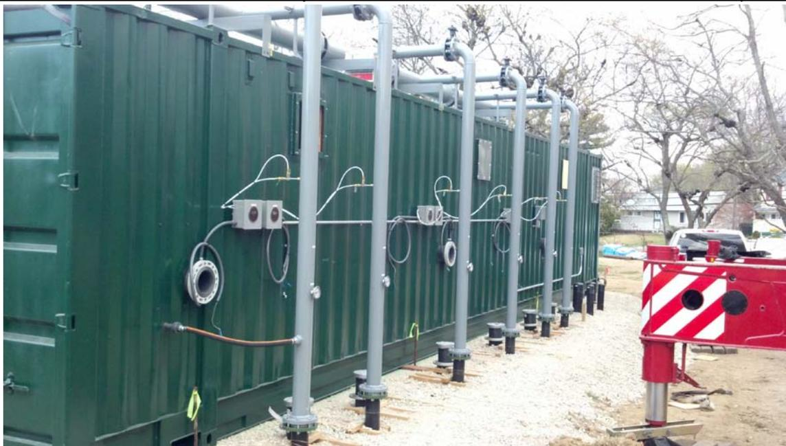
View of 4-in. DDC air supply lines connected to Treatment Trailer #1.
