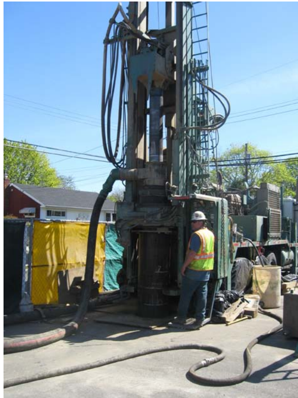
Layne drilling DDC-09, looking north.
