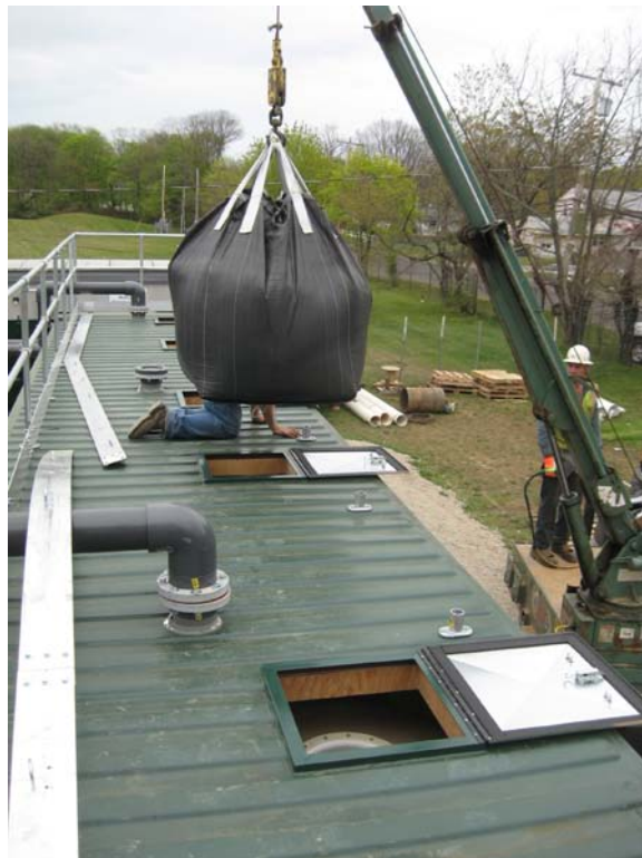
AECOM and Layne installing carbon through rooftop access panels.
