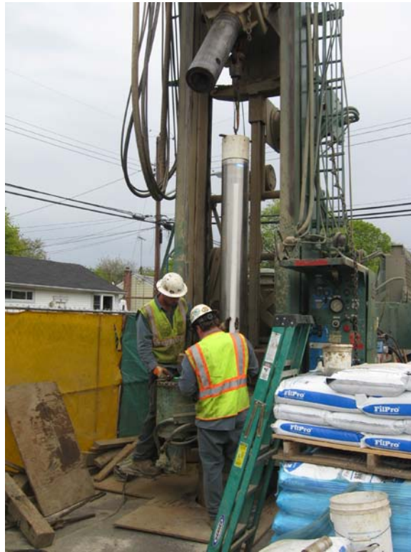
Layne installing upper screen at DDC-09.
