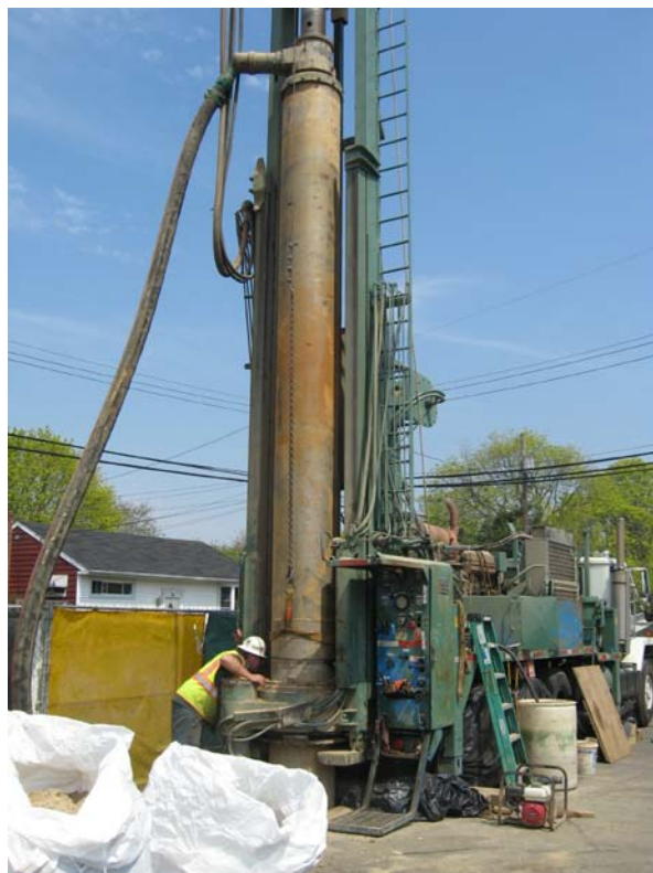
Layne drilling DDC-09, looking north.
