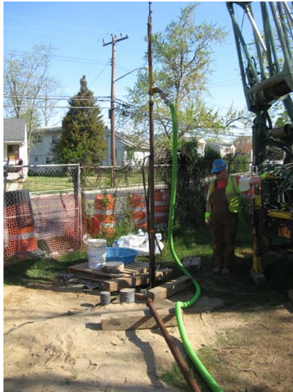
Layne developing DDC-05 recirculation well, looking north.
