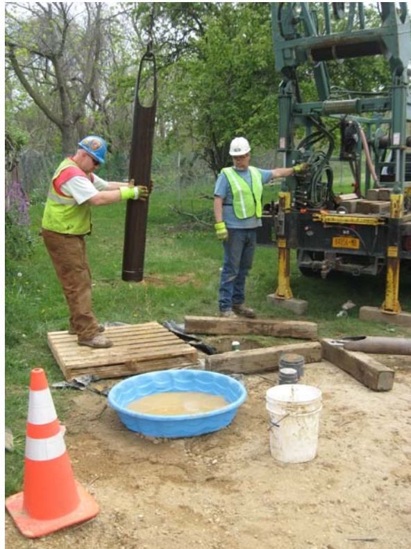
Layne bailing sediment from DDC-05, looking north.
