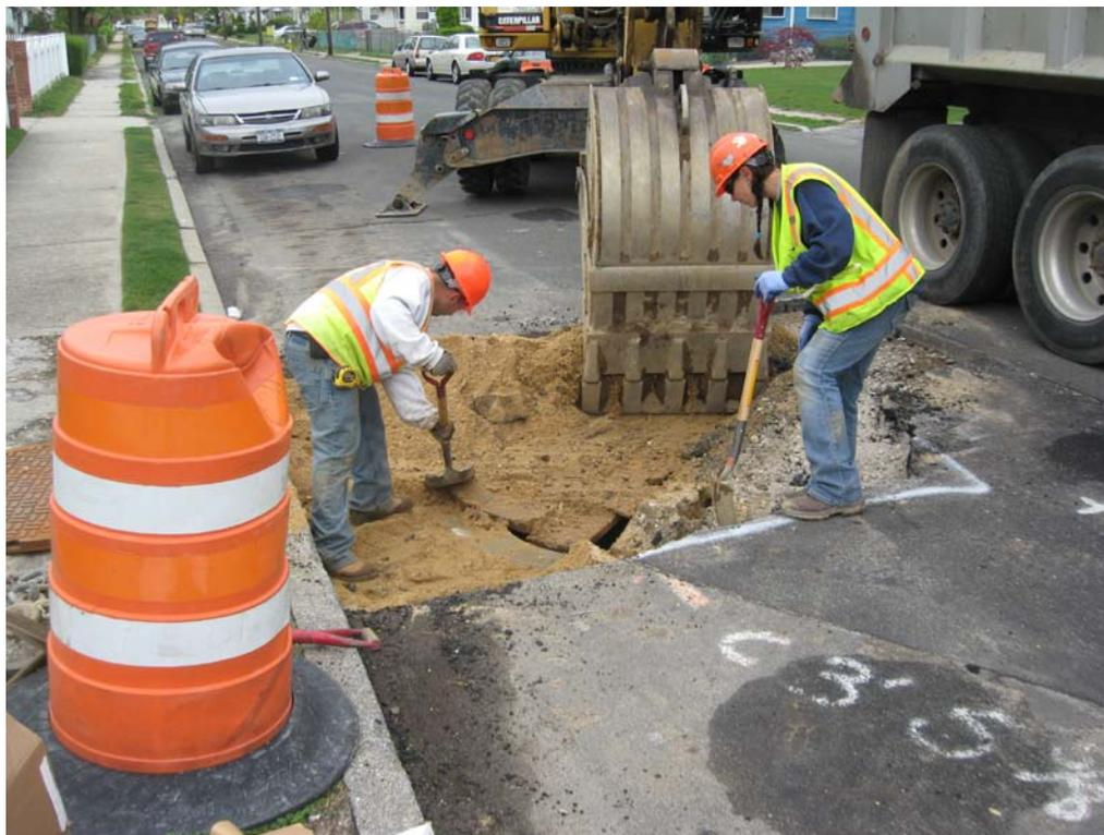
Posillico removing asphalt patch, timber, and sediment from DDC-10.
