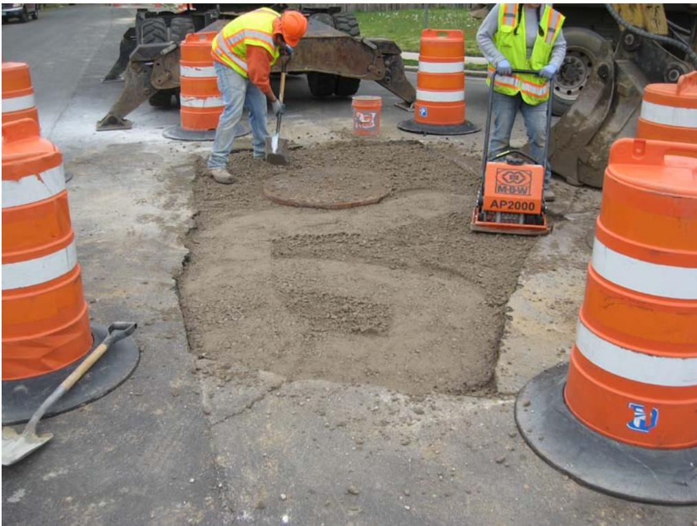
Posillico compacting road base material at DDC-09, looking east.
