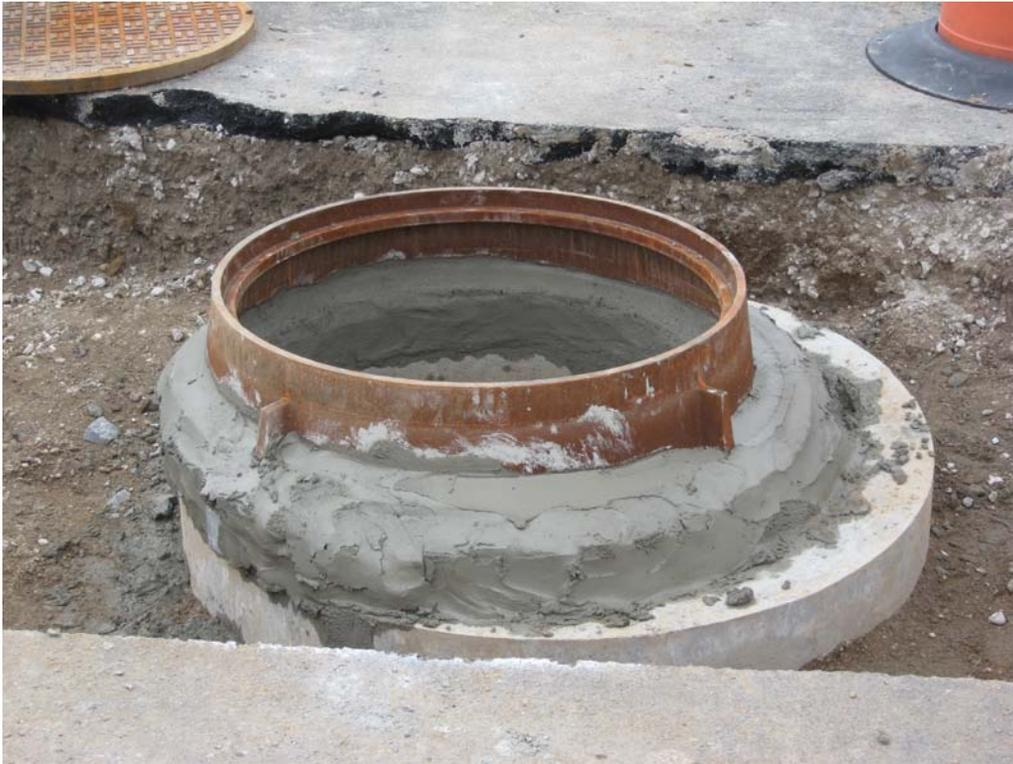
View of DDC-10 manhole frame and cover mortared to concrete vault collar.
