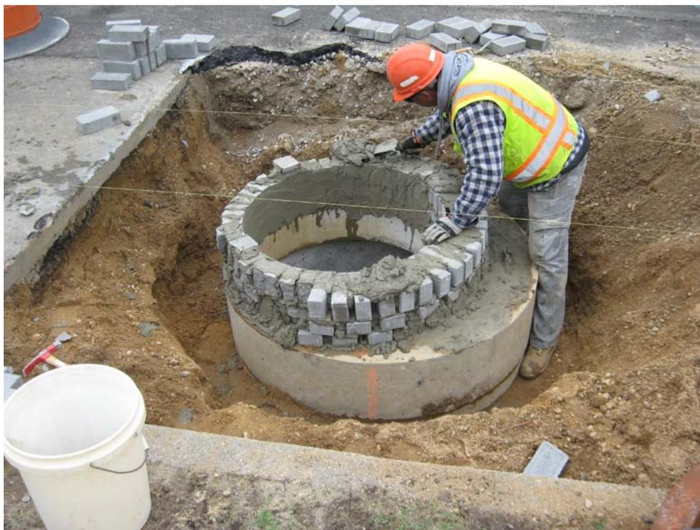
Bricks and mortar being placed to elevate manhole cover to grade.
