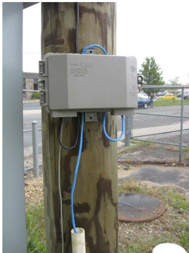
Close up view of Treatment System #2 phone line connection box.
