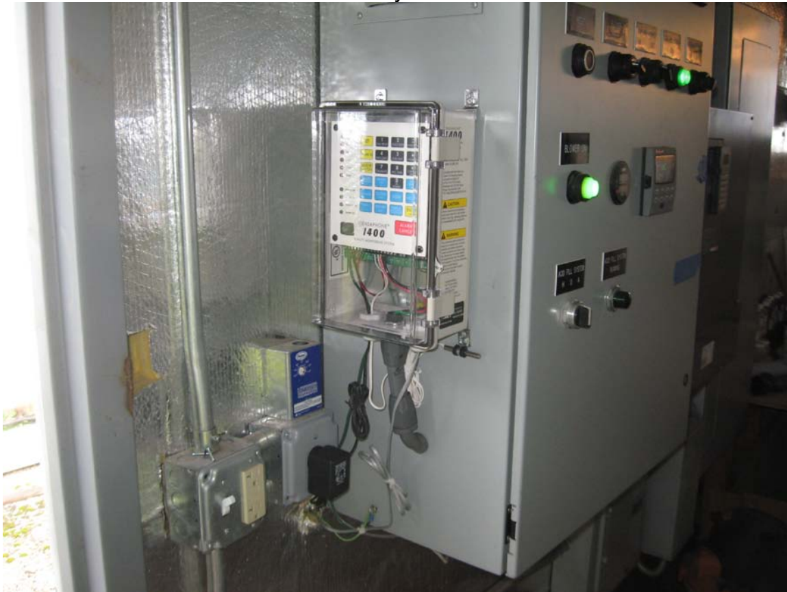
View of Treatment System #1 Sensaphone mounted to system control panel.
