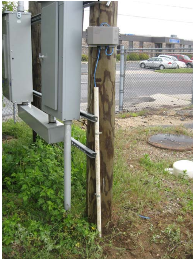
Verizon phone line connection box mounted to Treatment System #2 utility pole.
