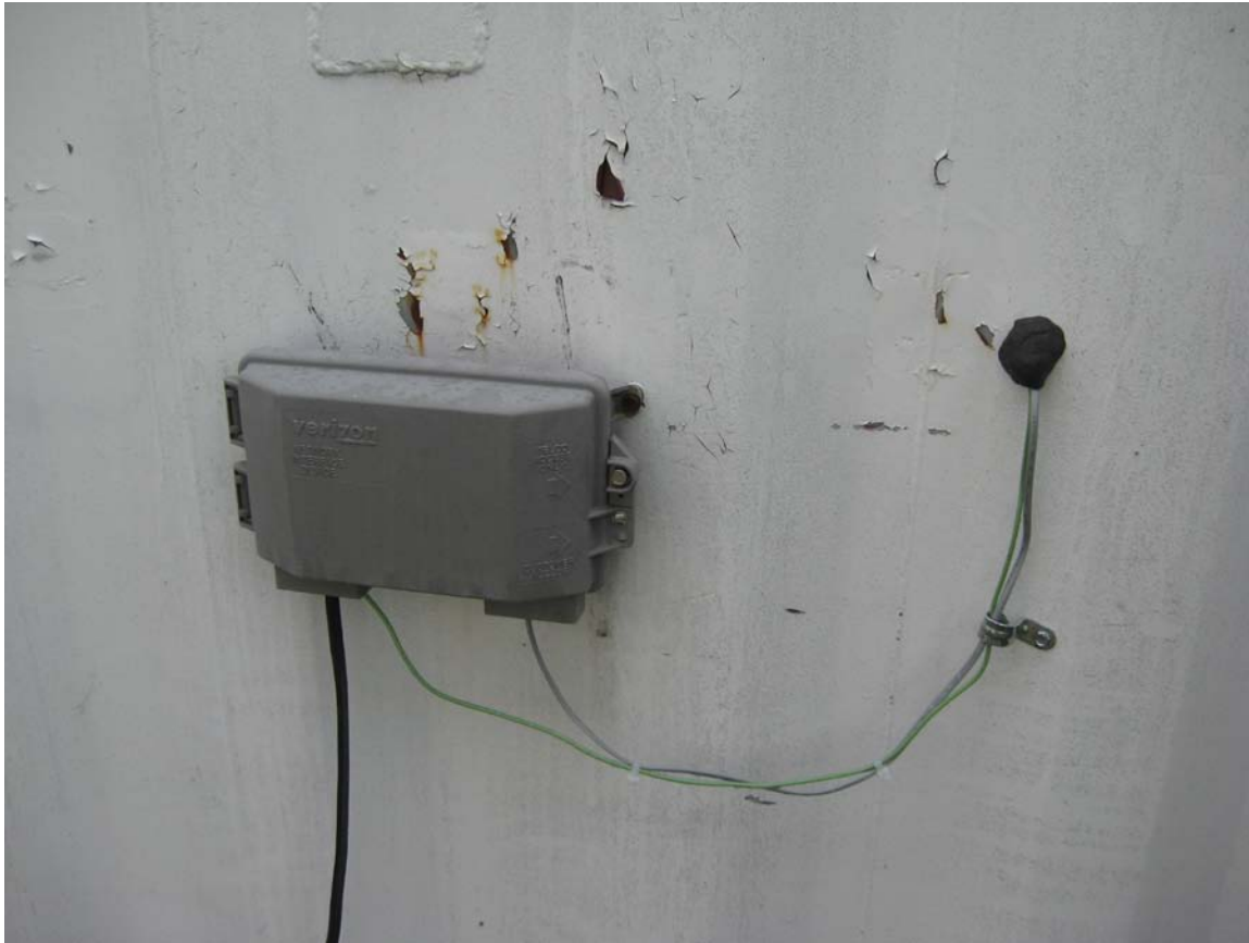
Verizon phone line connection box mounted to the exterior of Treatment System #1.
