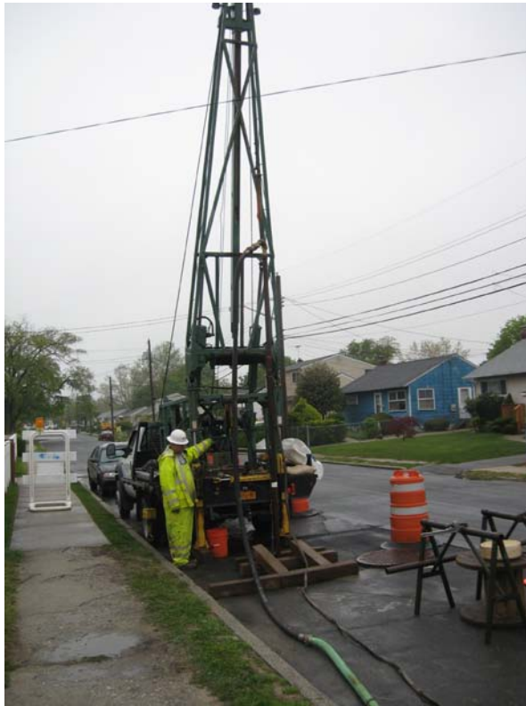
Layne surging and pumping DDC-10, looking west.
