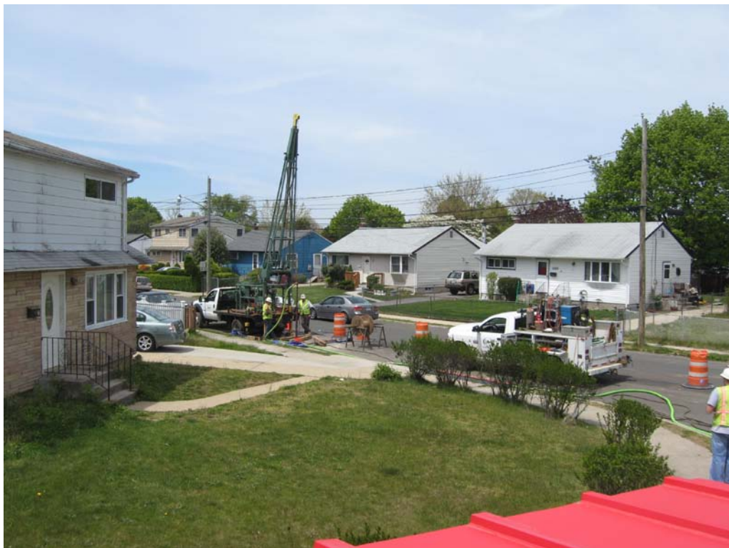
View of Layne pumping DDC-10, looking northwest.
