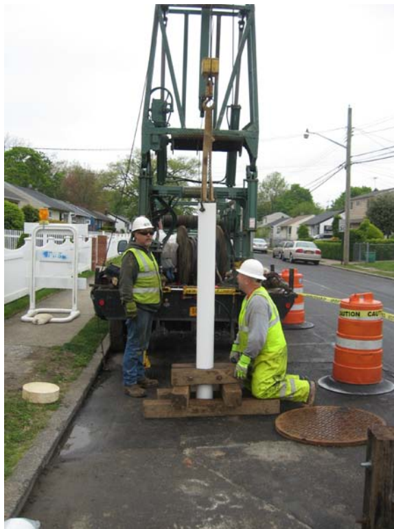
Layne installing DDC-10 eductor piping, looking west.
