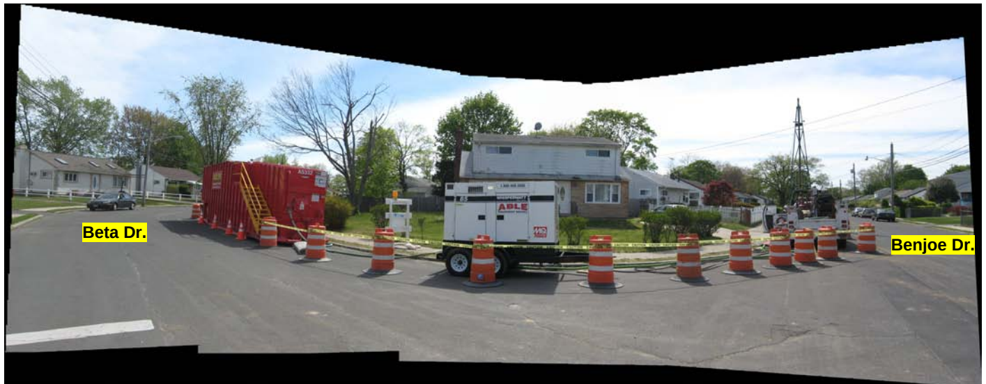
Panoramic view of traffic controls and exclusion zone. Standing at Benjoe & Beta Dr. intersection.
