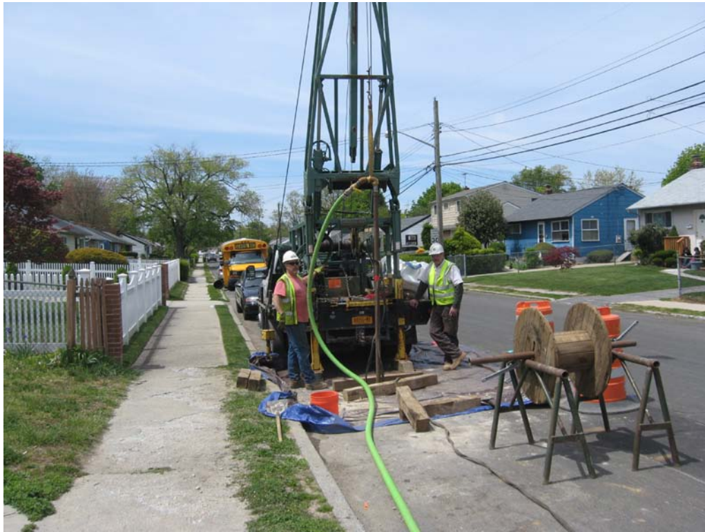
Layne surging and pumping DDC-10, looking west.
