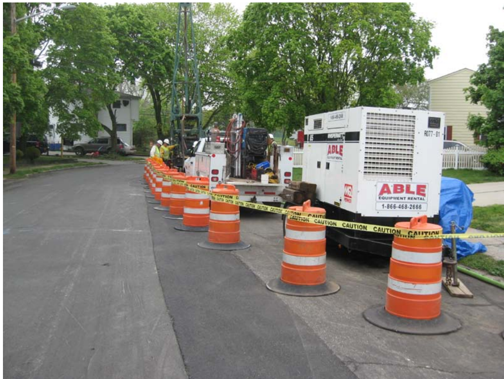
Traffic controls installed around DDC-07 development exclusion zone.
