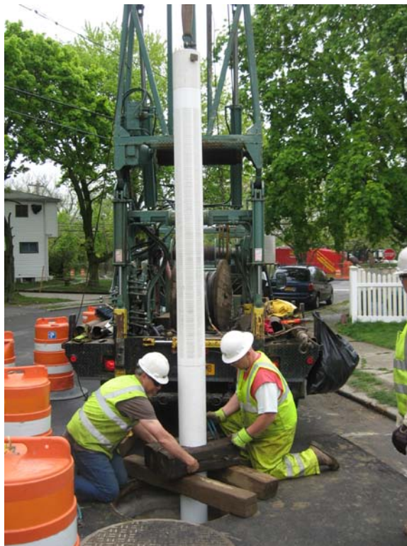
Layne installing DDC-07 eductor piping.
