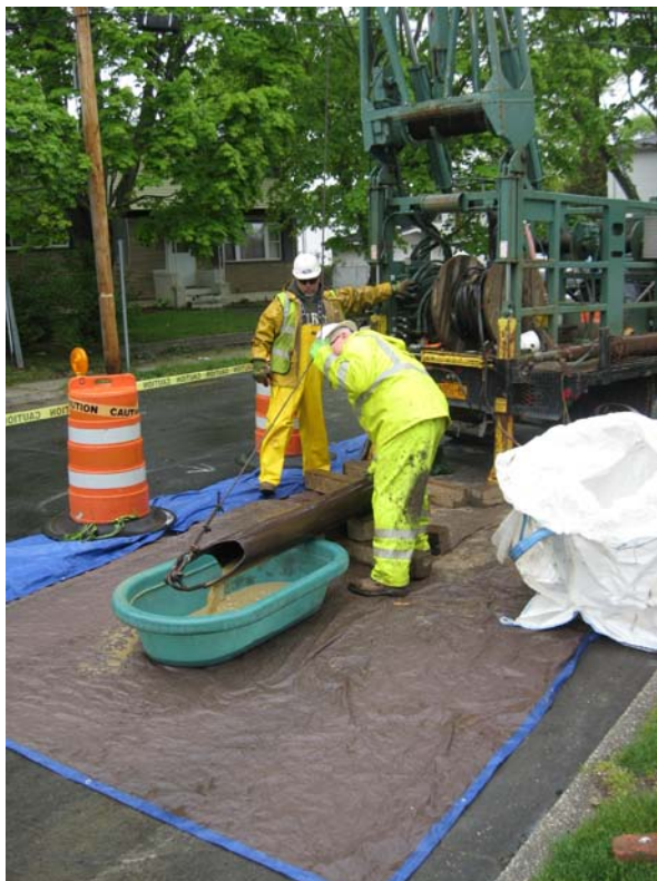
Layne bailing sediment from DDC-07 recirculation well.
