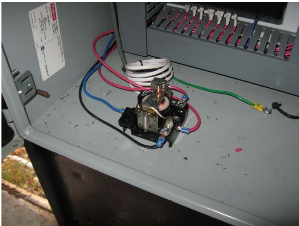
System #1 additional relay and associated connections.
