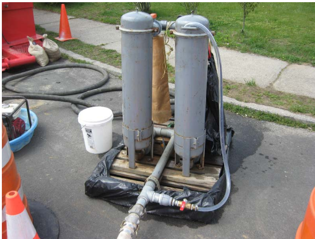
View of two vessel water filtration system mounted on secondary containment.
