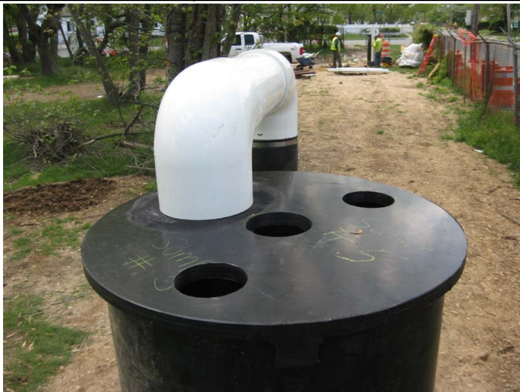
View of DDC-05 well head cover and 6-in. air return connection.
