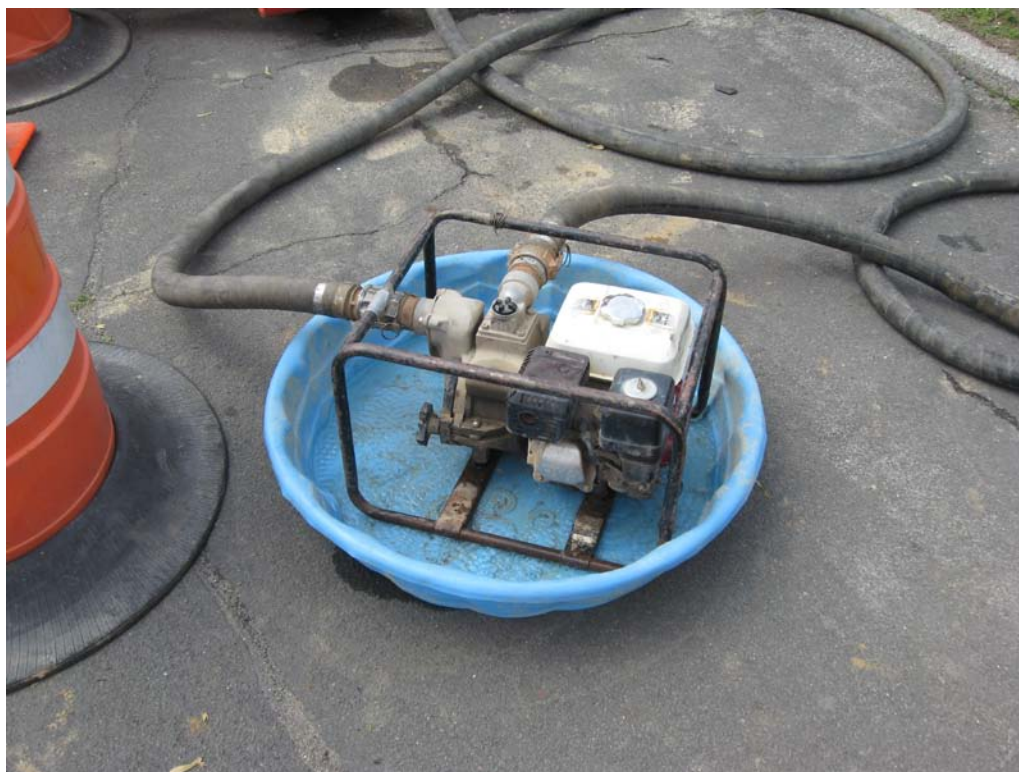
Development water discharge pump placed in secondary containment.
