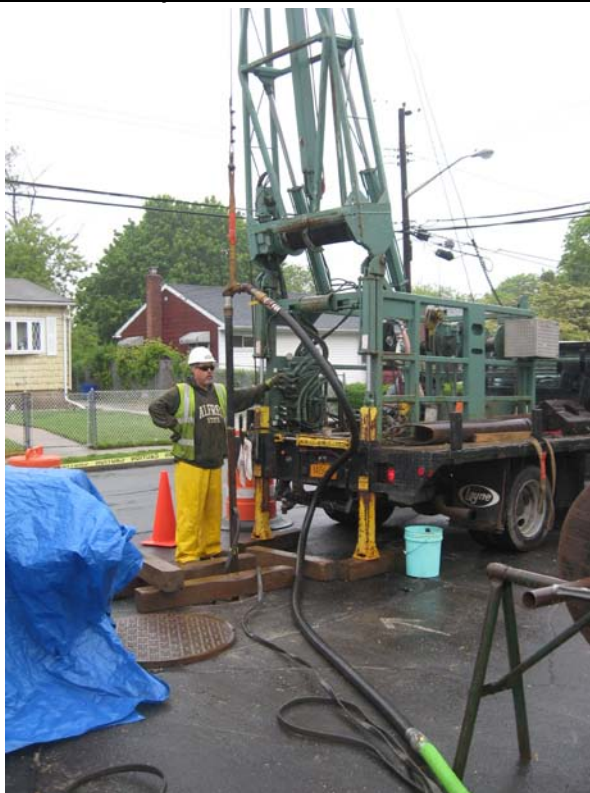
Layne surging and pumping DDC-09 lower screen.
