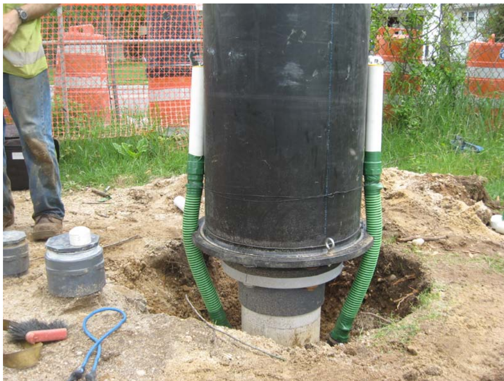
View of DDC-05 piezometers (green flexible piping).
