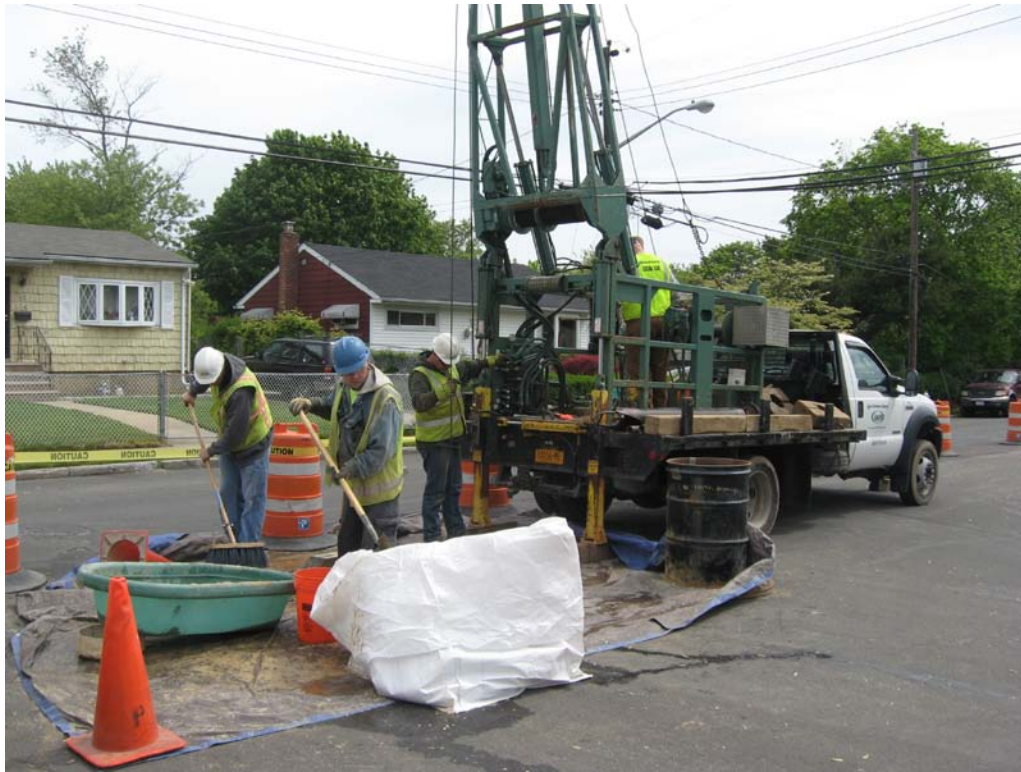
Layne bailing sediment from DDC-09.
