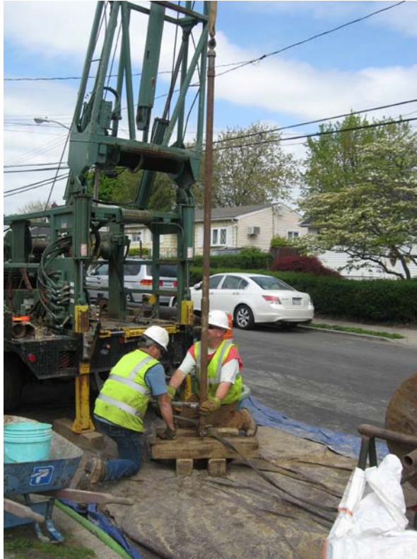
Layne pump/surge rods at DDC-08.
