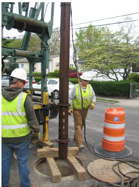
Layne lowering development pump at DDC-08.
