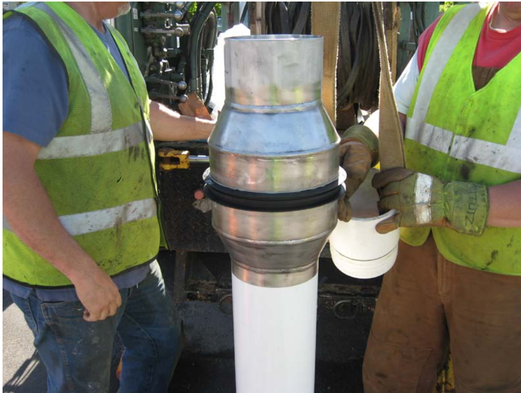
View of eductor piping and packer being installed.
