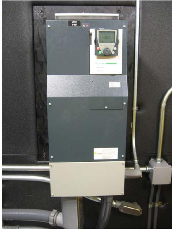
View of variable frequency drive (VFD).
