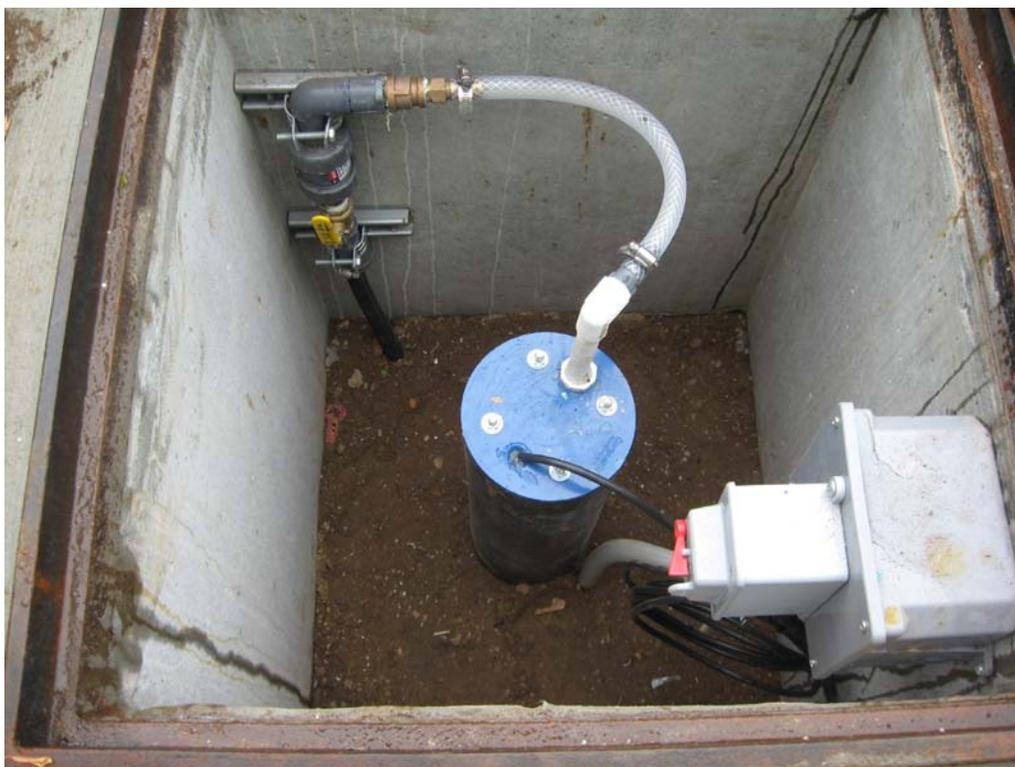
View of DDC-05 sump vault and sump discharge line.
