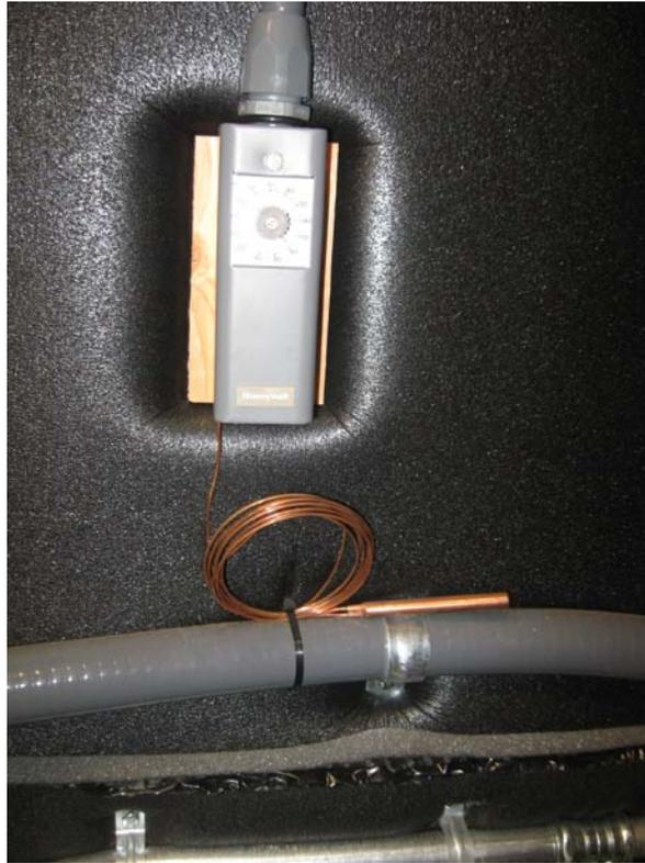
Thermostat control and temperature probe.
