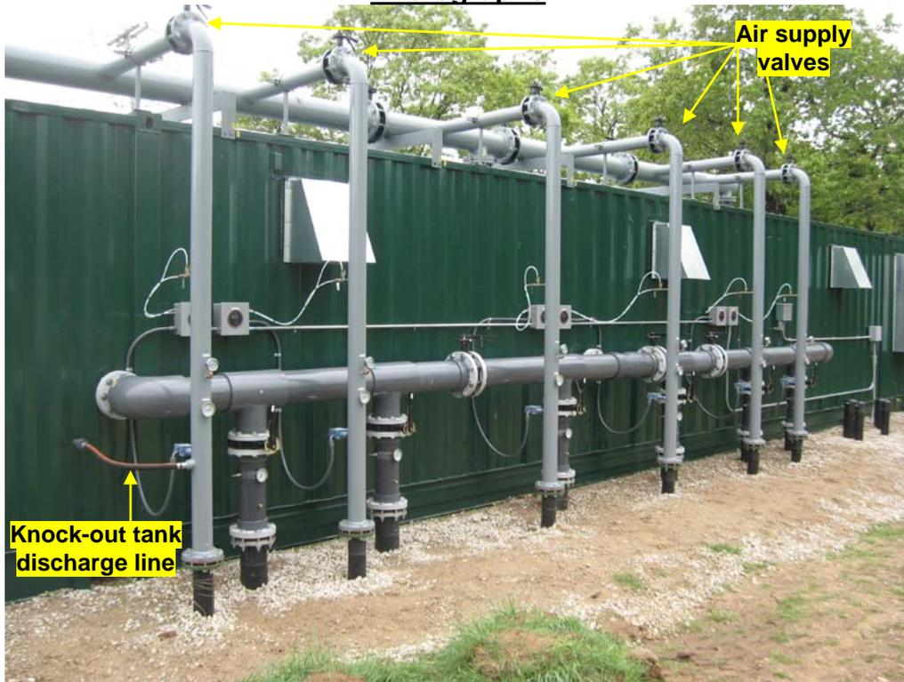
View of air-line piping manifold on exterior of system. Note location of knock-out tank discharge line and air supply valves.
