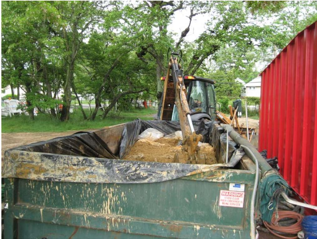
**Aarco solidifying sediment from frac tanks using saw dust and excavator.**
