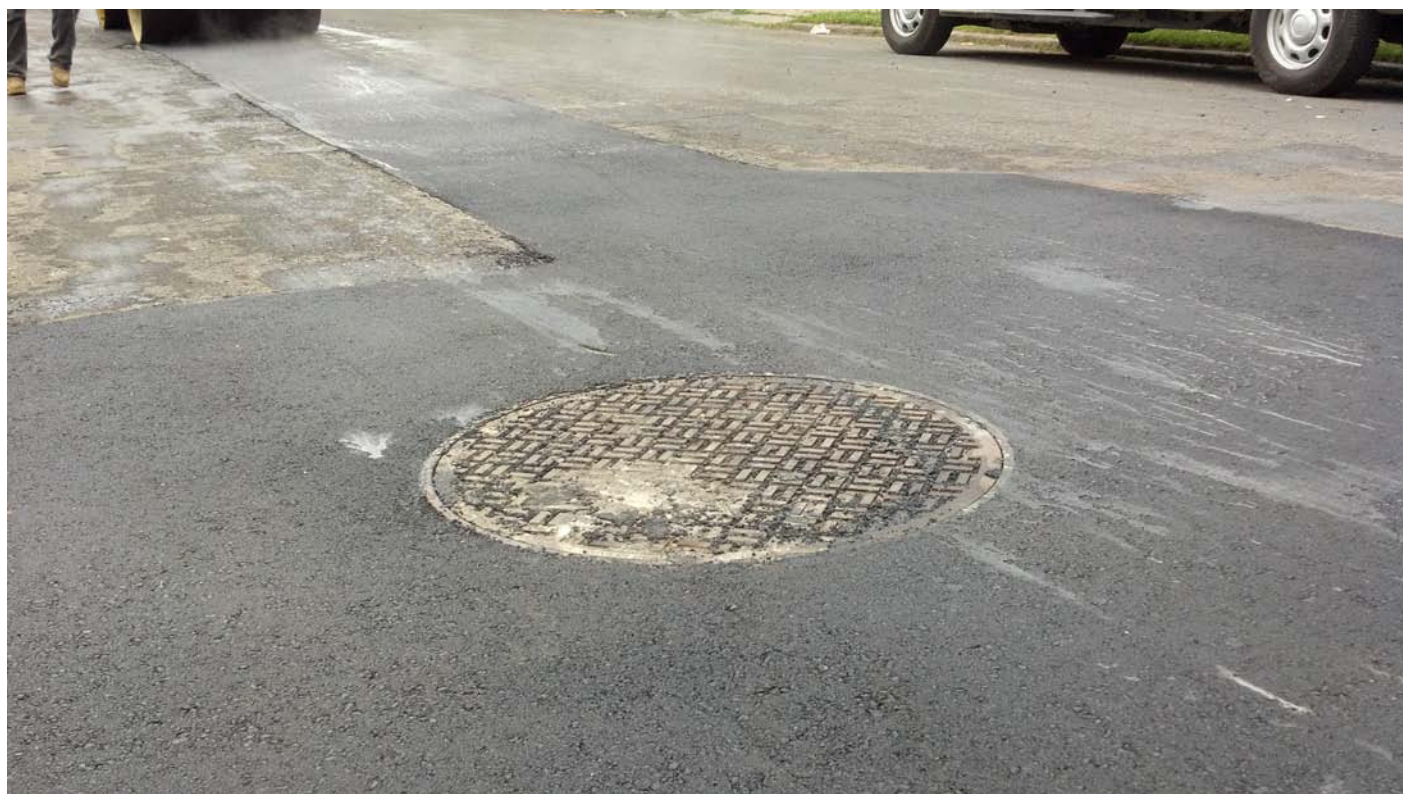
View of DDC-07 manhole cover and permanent asphalt.
