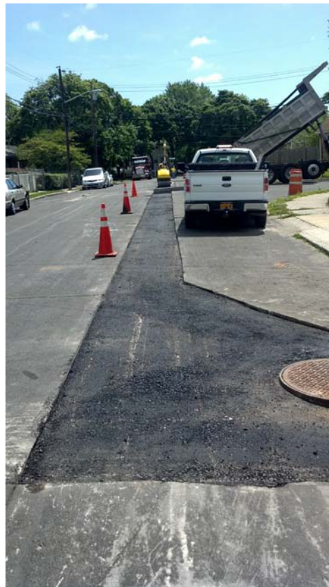
View of compacted asphalt binder. Standing at DDC-10 looking east.
