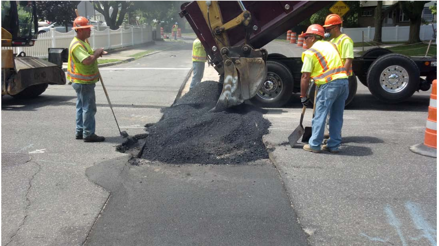
Posillico placing permanent asphalt binder along offsite DDC trench line.
