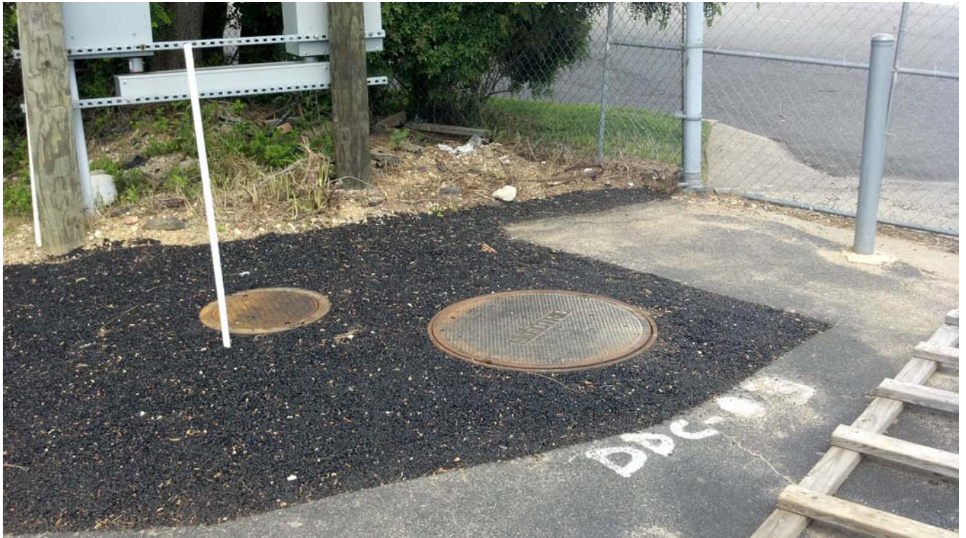
View of onsite cold patch asphalt around DDC-03 and sump.
