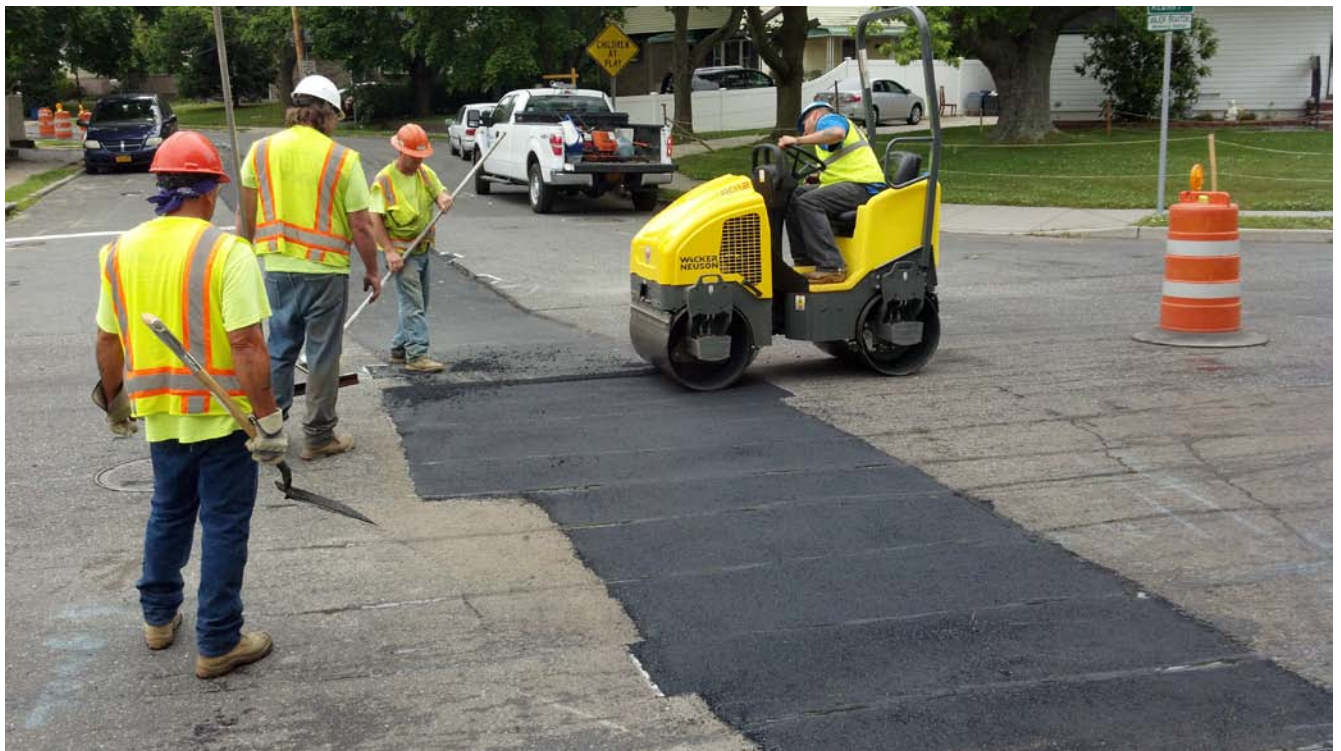
Posillico compacting permanent asphalt top coat using a roller compactor.
