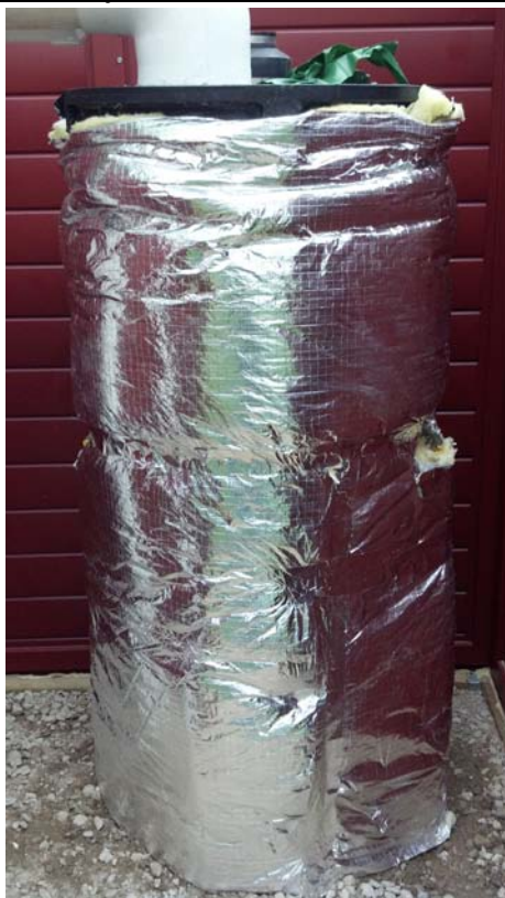
View of DDC-05 well head wrapped with insulation.
