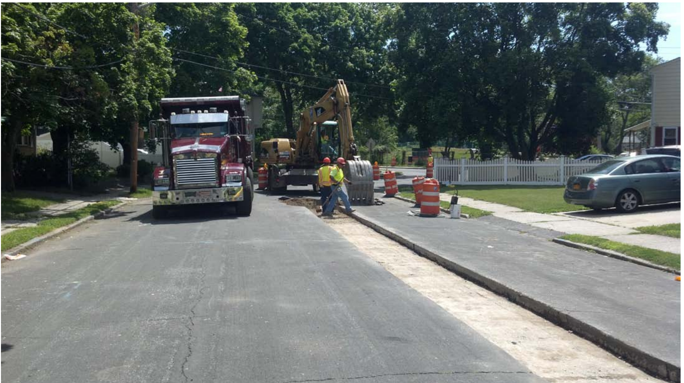
Posillico removing temporary asphalt along offsite DDC trench line.
