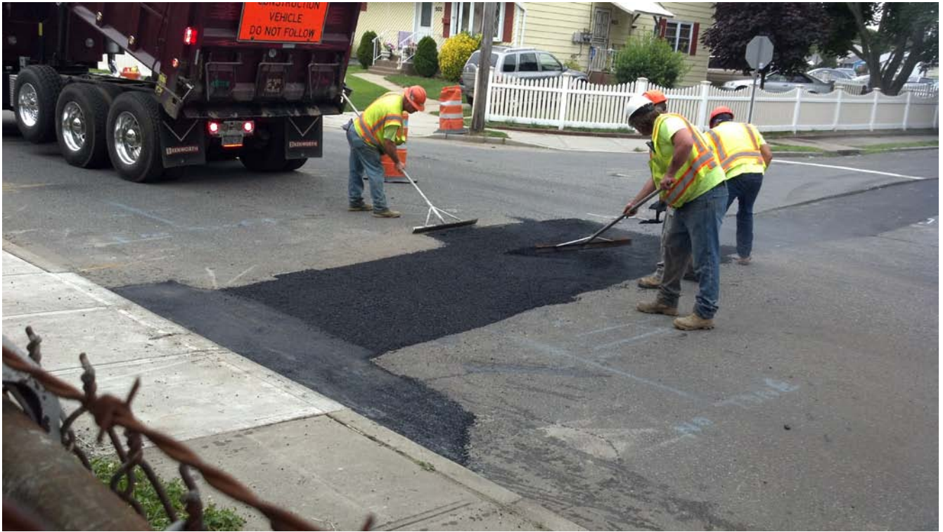
View of Posillico placing permanent asphalt top coat along Albany Ave.
