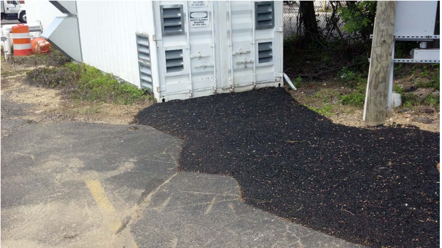
View of onsite cold patch asphalt along DDC-03 trench line and Treatment System #2.
