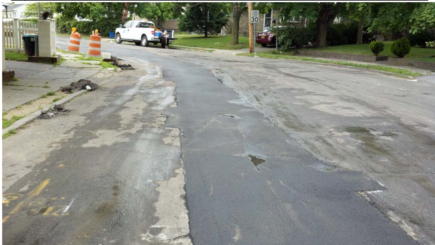
View of permanent asphalt along DDC trench line.
