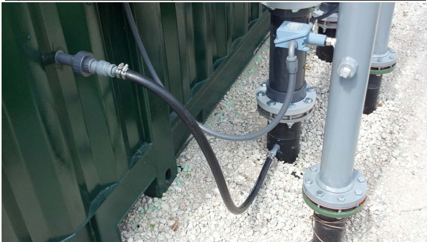
View of relocated knock-out tank discharge line.
