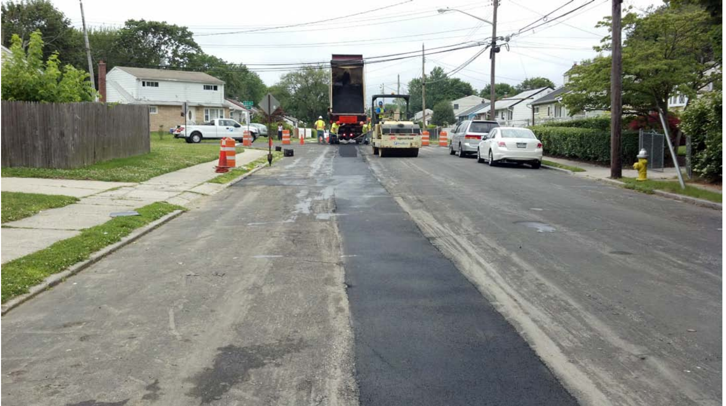
View of permanent asphalt along DDC trench line, looking west.
