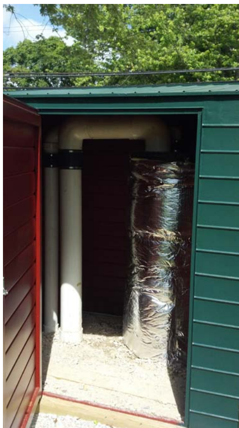
View of DDC-06 well head and piping in shed.
