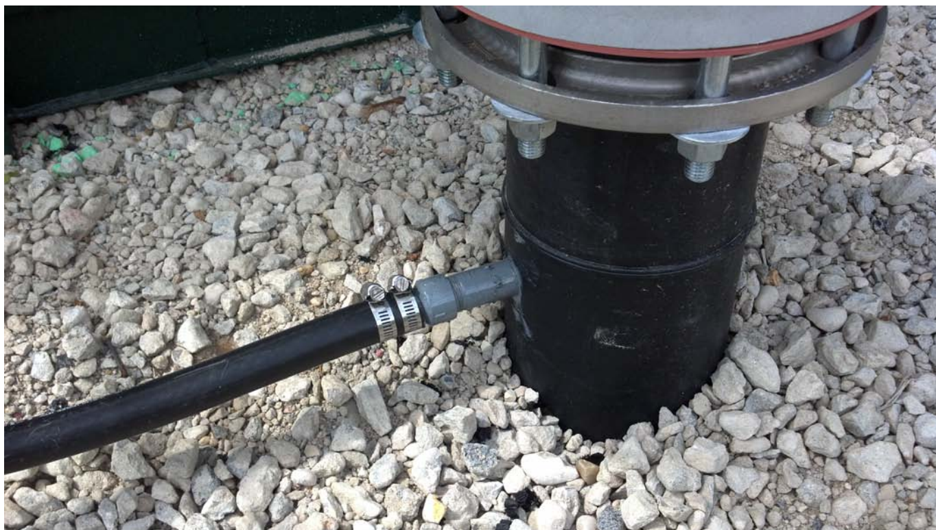
Close-up view of knock-out discharge line connection to DDC-06 air return pipe.
