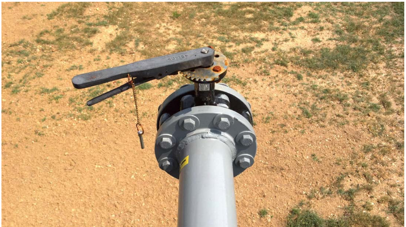
View of existing 4-in. air supply valve handle.
