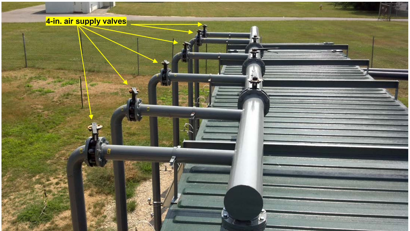
View of overhead 4-in. air supply valves.
