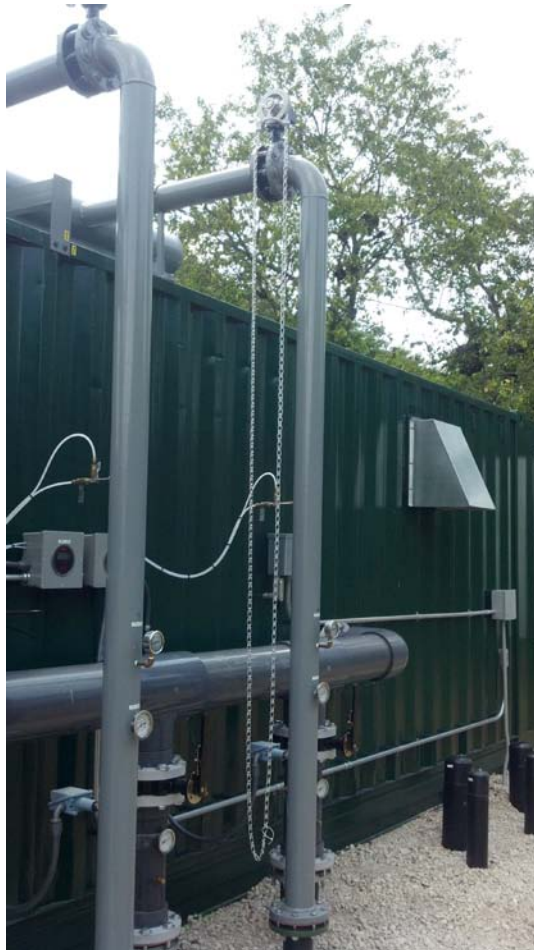
View of chain extending down to ground level.
