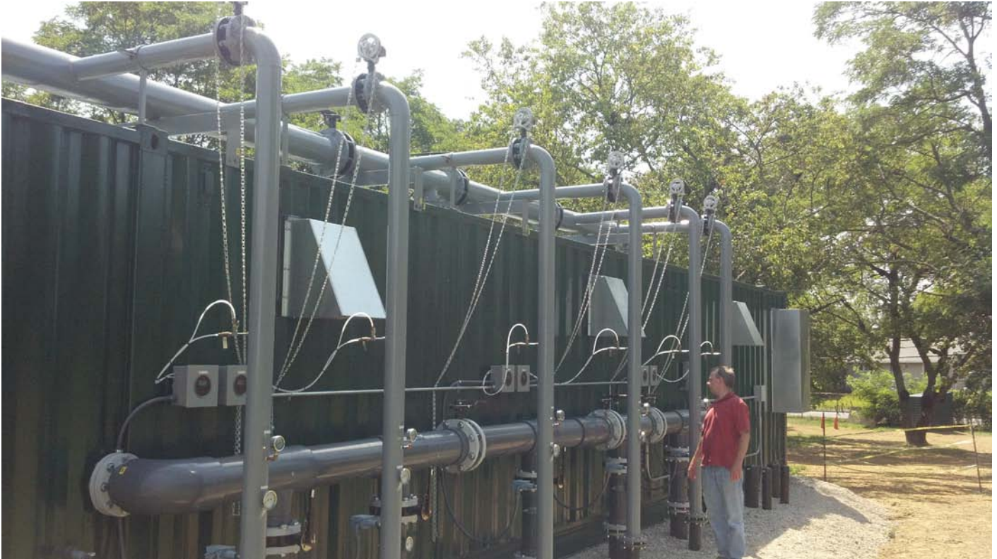
View of piping manifold area and chain wheel drives. Chains pulled behind conduit pipe located on treatment trailer. Locks were placed on each chain to prevent tampering.
