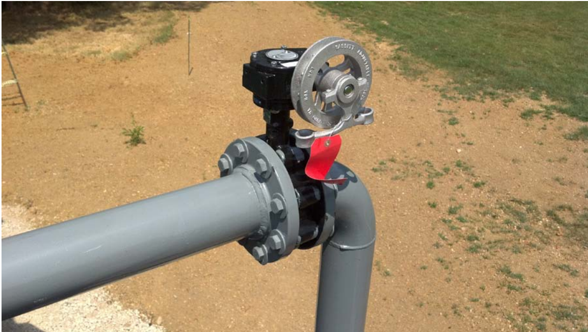
View of newly installed chain wheel drive on 4-in. air supply valve.
