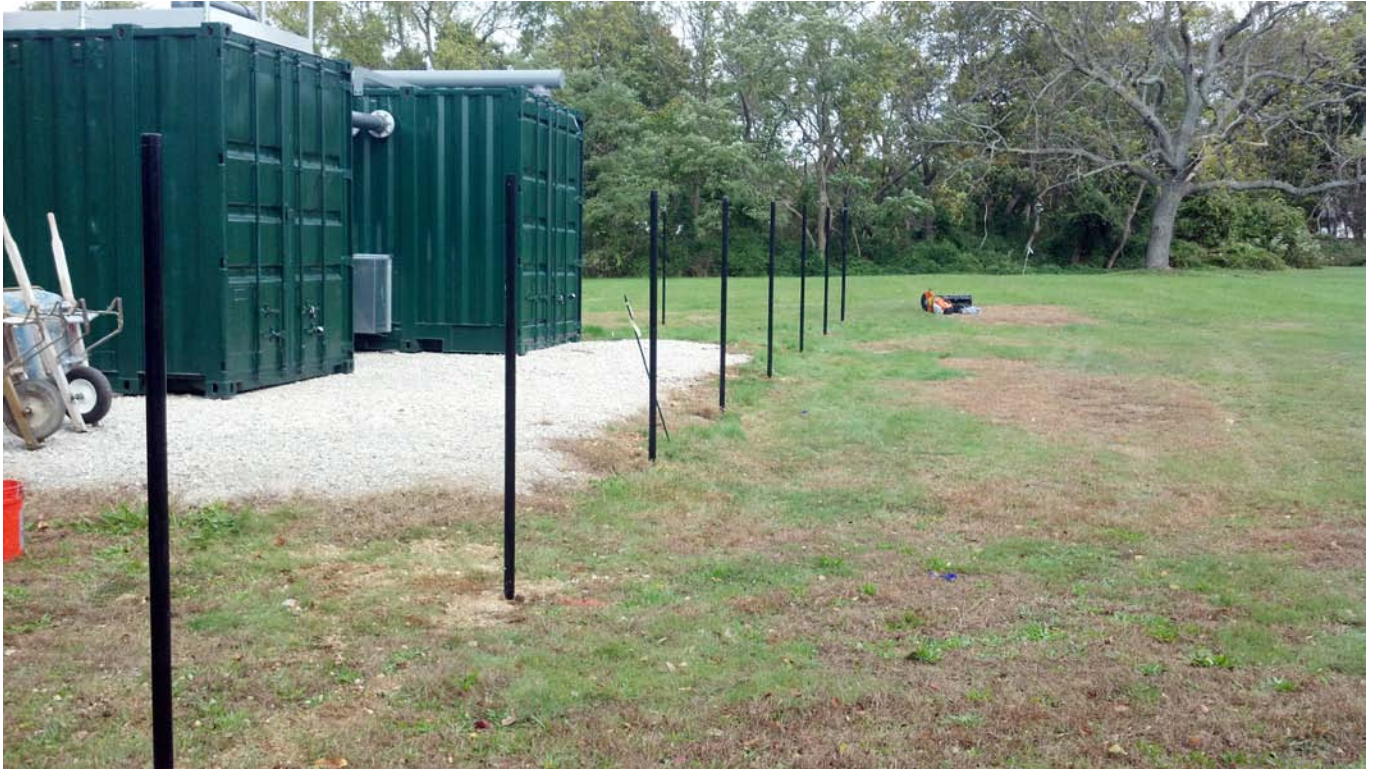
View of fence posts along eastern side of treatment system pad.
