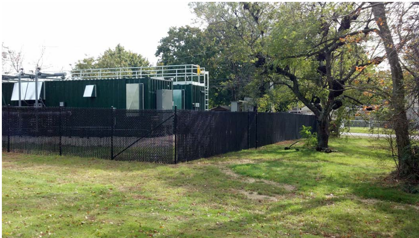
View of fencing along western side of treatment system pad.
