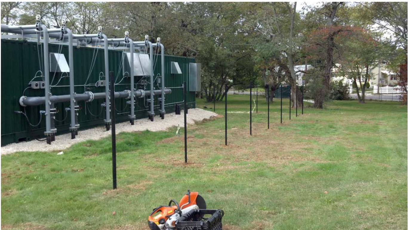
View of fence posts along north side of treatment system pad.
