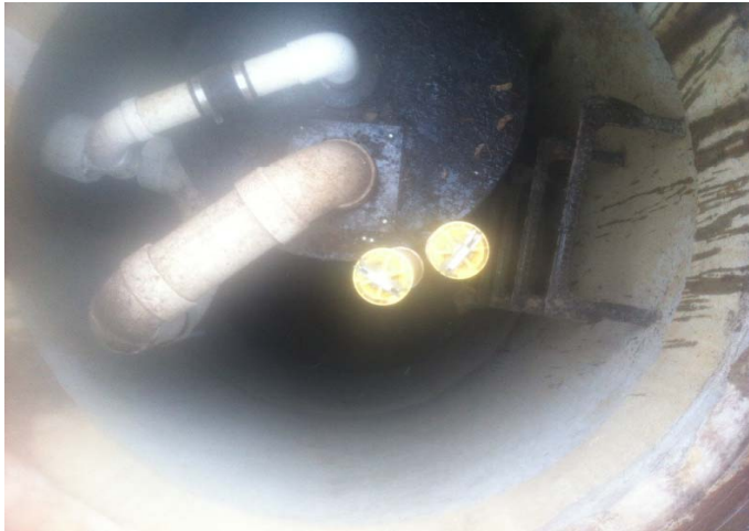
Picture 303- All DDC wells within the SCWA property and along Benjoe Drive were gauged and inspected.
