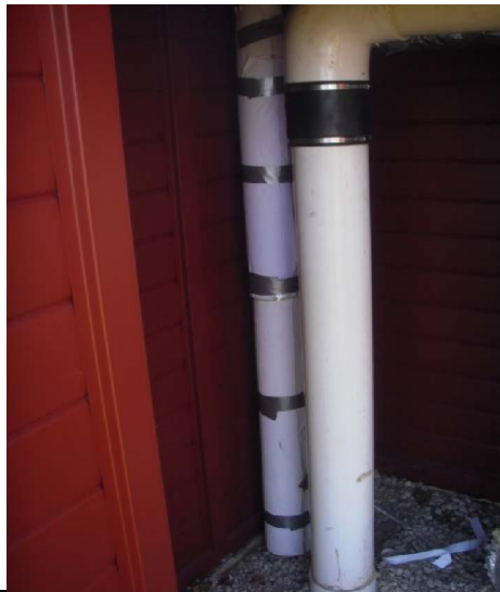
Picture 352- Pipe insulation was installed on the four (4)-inch injection lines within the DDC-5 & 6 sheds.
