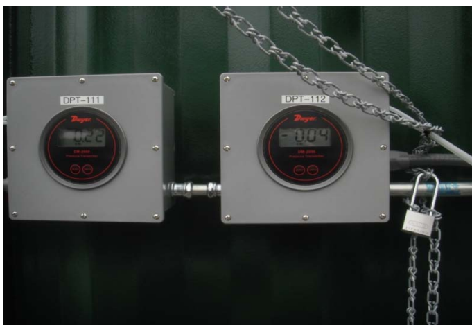
Picture 350- The vacuum gauge, DPT-112, was reading a negative number.
