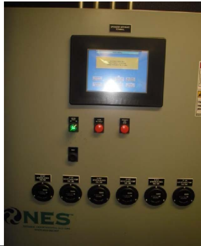
Picture 333- All alarms were reset, with blowers B-501 & B-502 up upon departure.
