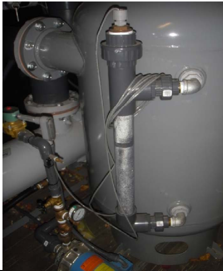
Picture 336- No water was observed within the ST-201 separator's site glass.
