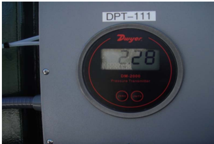
Picture 396- The differential pressure gauges associated with the four (4)-inch injection lines were observed to read elevated compared to prior readings.
