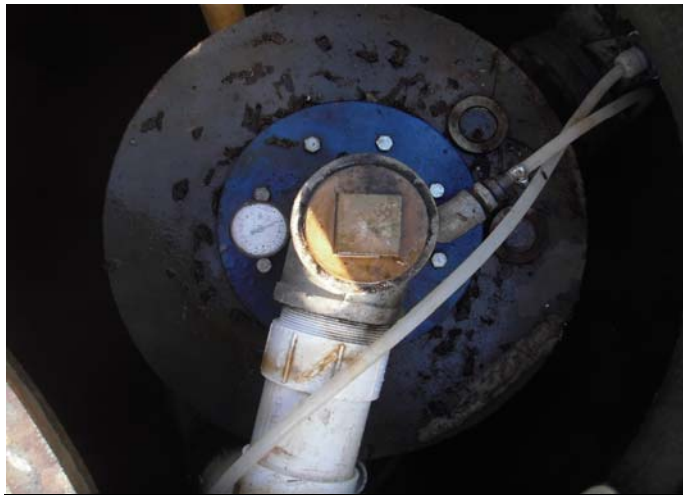
Picture 399 - View of the DDC-4 well with its associated pressure gauge reading 0.4 PSI.
