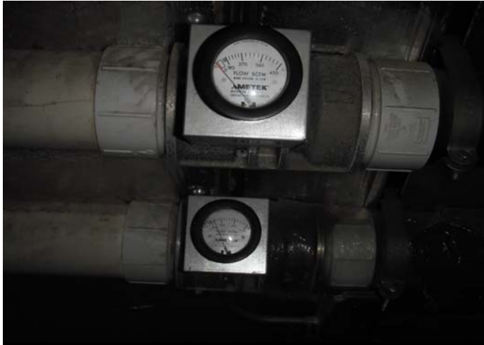
Picture 389 - Flow Gauge, FI-01, is non-functioning and needs to be replaced.
