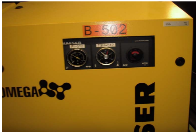
Picture 396- The temperature gauge (TSH-512) on the B-5012 blower panel was reading 155 degrees Fahrenheit.
