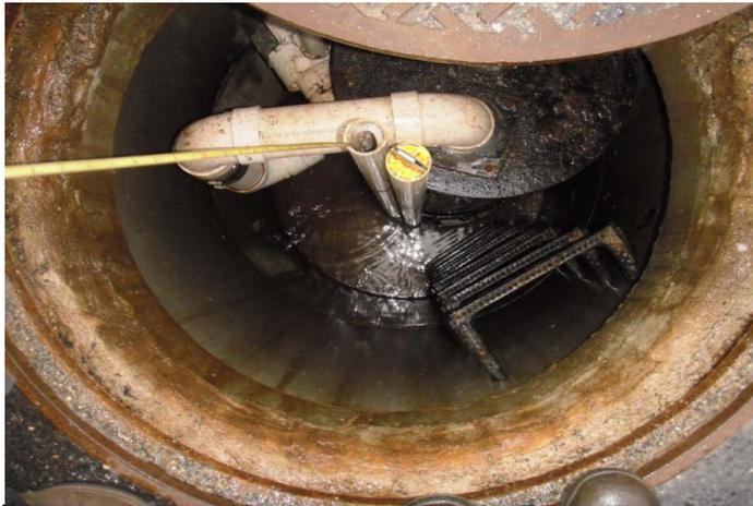
**Picture 464-** The shallow and deep piezometer wells were gauged within each DDC well.
