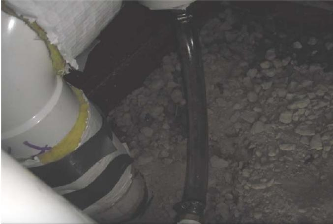
**Picture 462-** Trapped water was observed within the DDC-5's 1-inch condensate drain when the ball valve was turned off.
