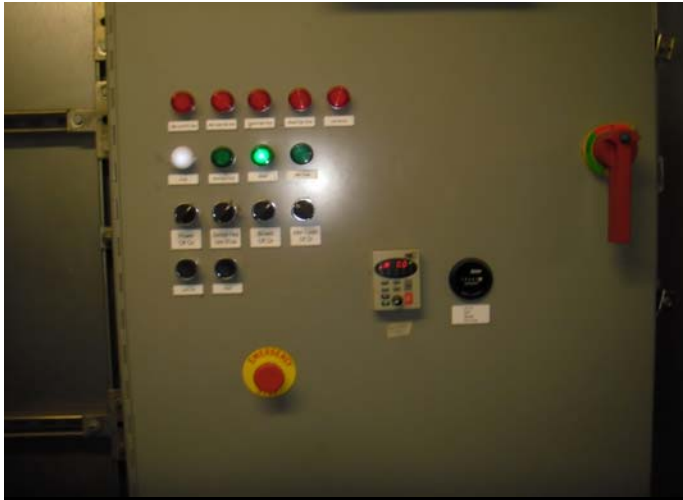
Picture 452 - System #2 was on upon arrival with no alarms triggered on the control panel.
