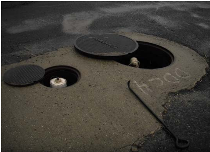
Picture 458 - DDC-4 and its associated sump was visually inspected. The sump pump has continued to be non-functioning since 1/17/2013.
