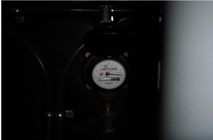
Picture 458- No additional water has been observed to have discharged out of the shed from the moisture separators as per the FM-601 gauge.
