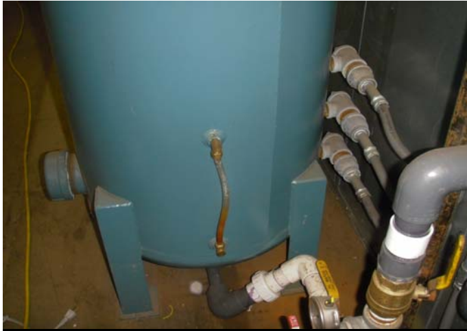
Picture 014 - No water was detected within the System #2's knock-out tank.
