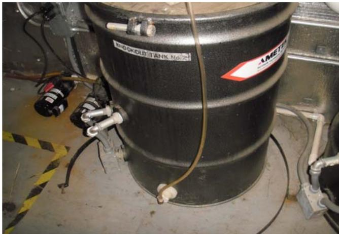
**Picture 008** - No water was observed in the site glass associated with either knock out tank in System #1.
