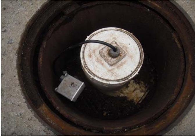
**Picture 006** - DDC-4's sump pump was replaced. Water was observed to discharge from sump into DDC-4 after installation.
