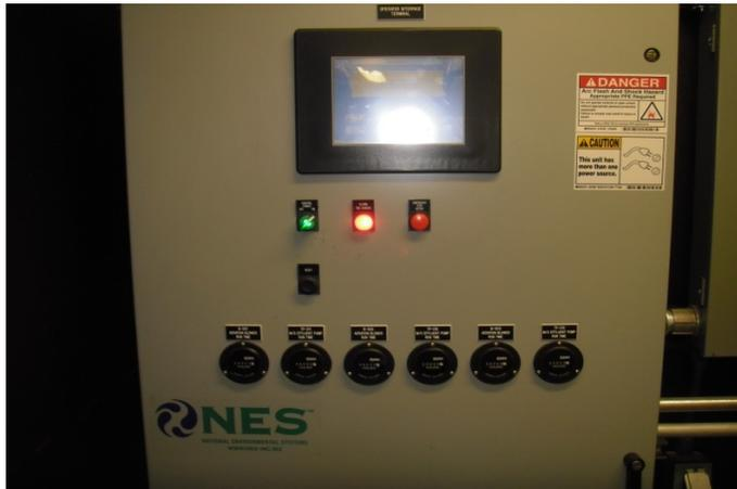
**Picture 009-** Four (4) low-pressure alarms were noted on the control panel upon arrival.
