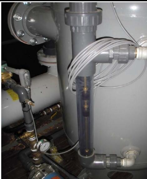
**Picture 011-** No water was observed within the site glasses of either of the blowers.
