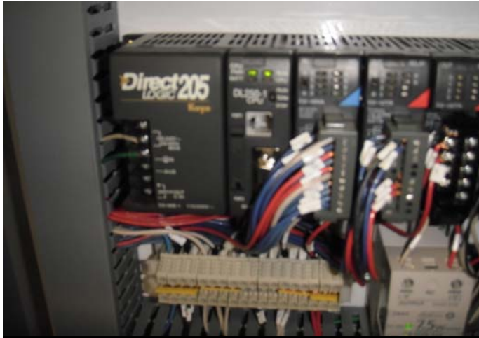
Picture 002 - View of the Direct Logic 205 unit within the control panel of System #2.
