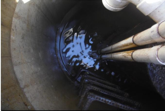
**Picture 008-** Two (2) feet of water was observed within the DDC-08 vault.
